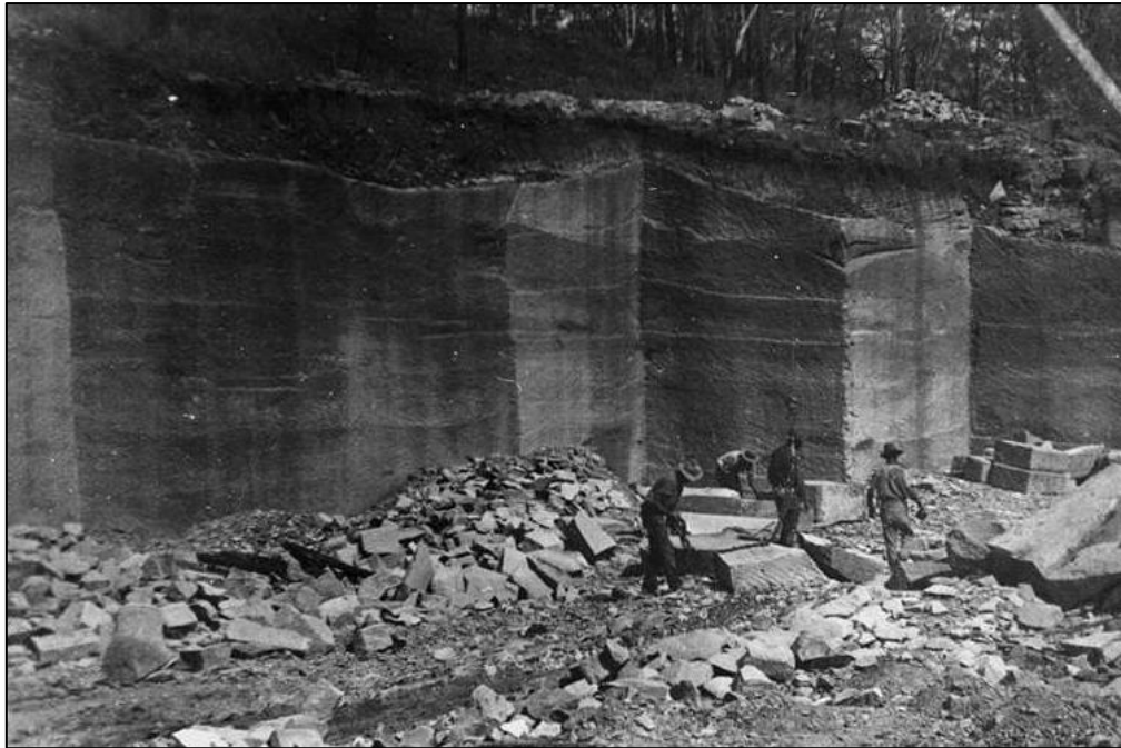
Figure 1. Workers at Stanwell Quarry, circa 1898, preparing stone for the Catholic Cathedral, Rockhampton. Image courtesy of State Library of Queensland.
