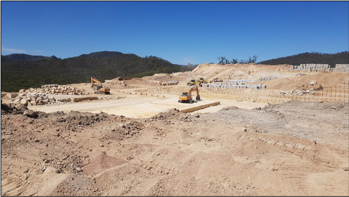
Figure 11. Excavator mounted saw cutting blocks at the site.
