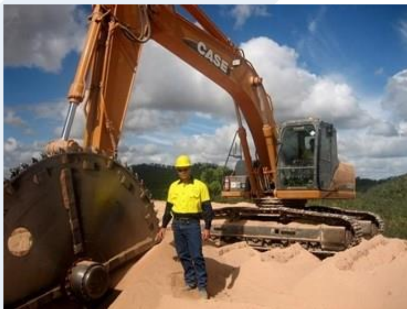
Figure 2. Excavator mounted stone saw.
