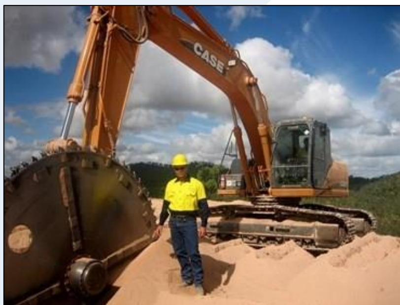
Figure 2. Excavator mounted stone saw.
