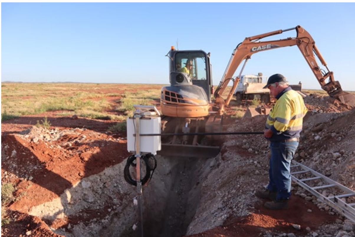
Photo 1 Example of the installation of an instrument tree at Wallace South Project
