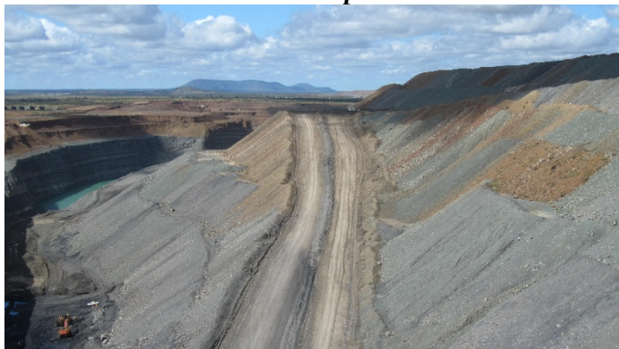
Photo taken 11/05/2017, looking SE
