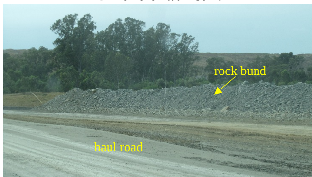
Photo taken 9/05/2017, looking E
