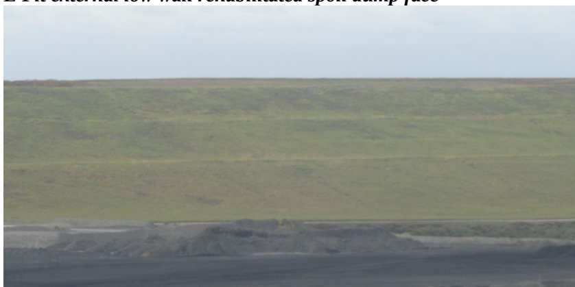
Photo taken 9/05/2017, looking NE
