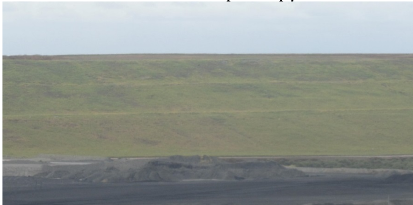
Photo taken 9/05/2017, looking NE
