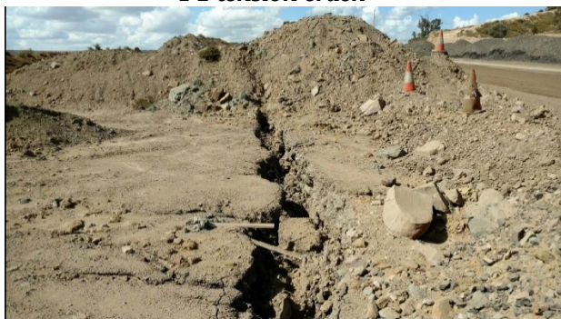
Site Photo taken 9/05/2017, looking NE
