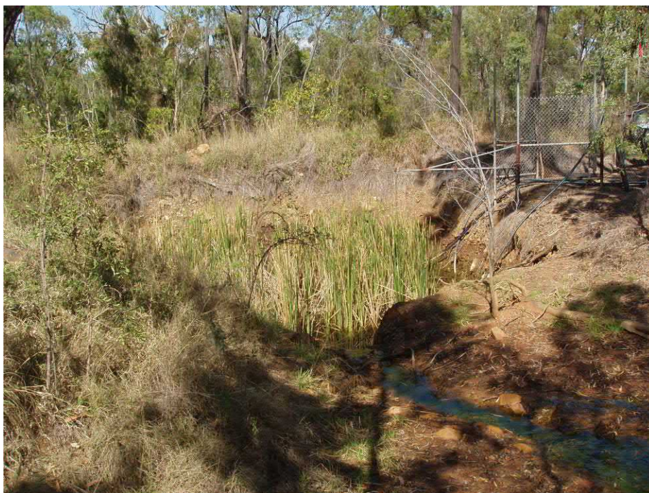
Settlement Dam Sump
