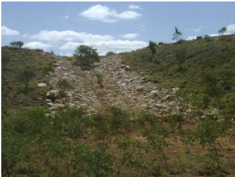
Drop structure on Roche Hill
