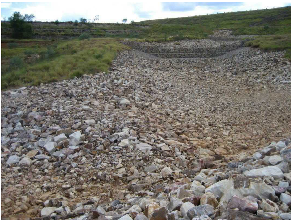
Mt Hope Dam high flow bypass facility
