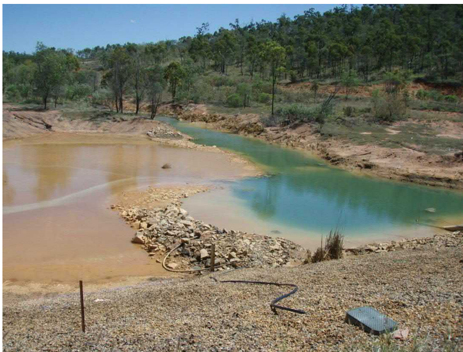
Plum Tree Creek Dam
