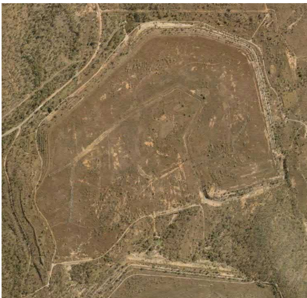
Figure 3.4: Recent Imagery – NNTSF (Source: Queensland Globe)
