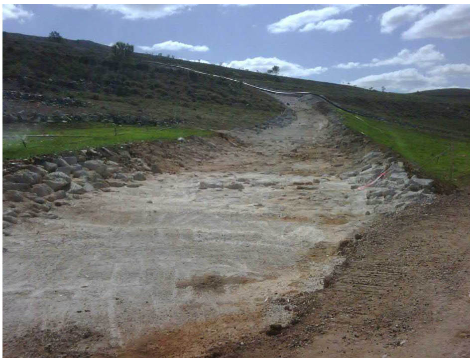
Diversion of drop structure above Mt Mawe Dam
