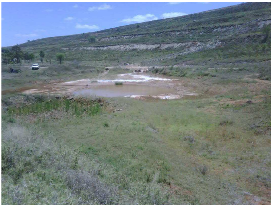
Mt Hope Extension Dam
