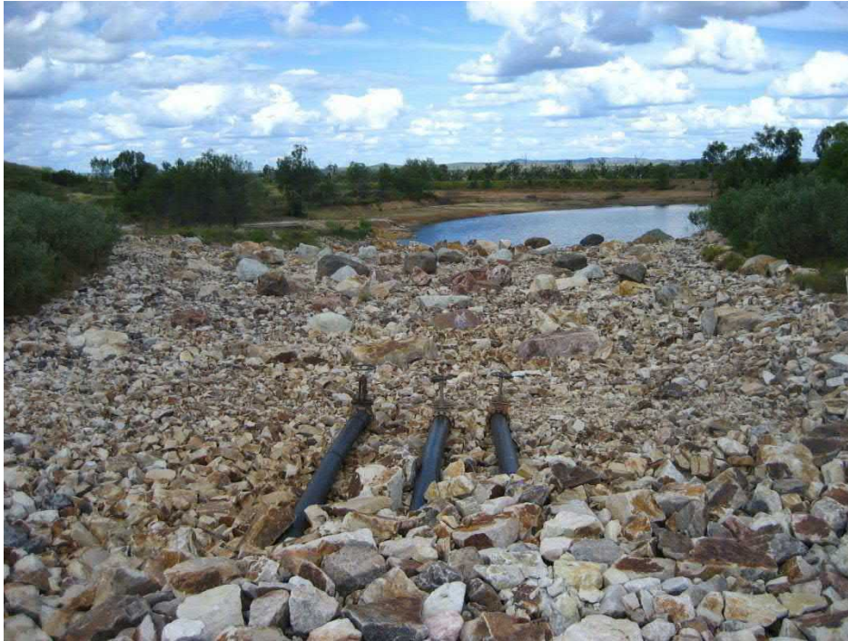
Mt Hope Dam high flow bypass facility
