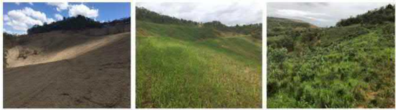
Figure 1.49: Roche Hill after 2017 Rehabilitation Works
