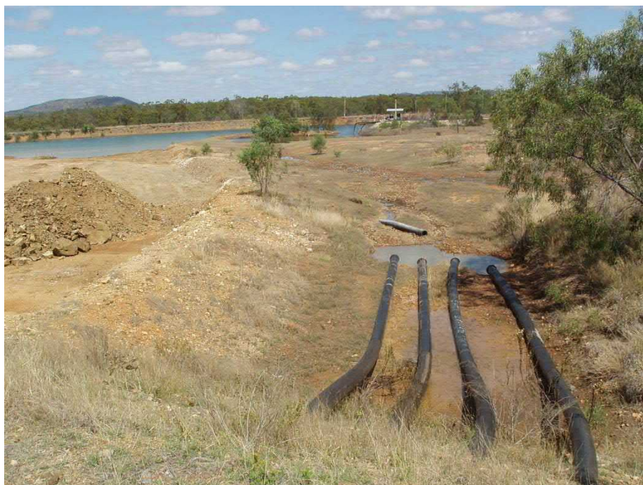
Settlement Dam high flow bypass facility
