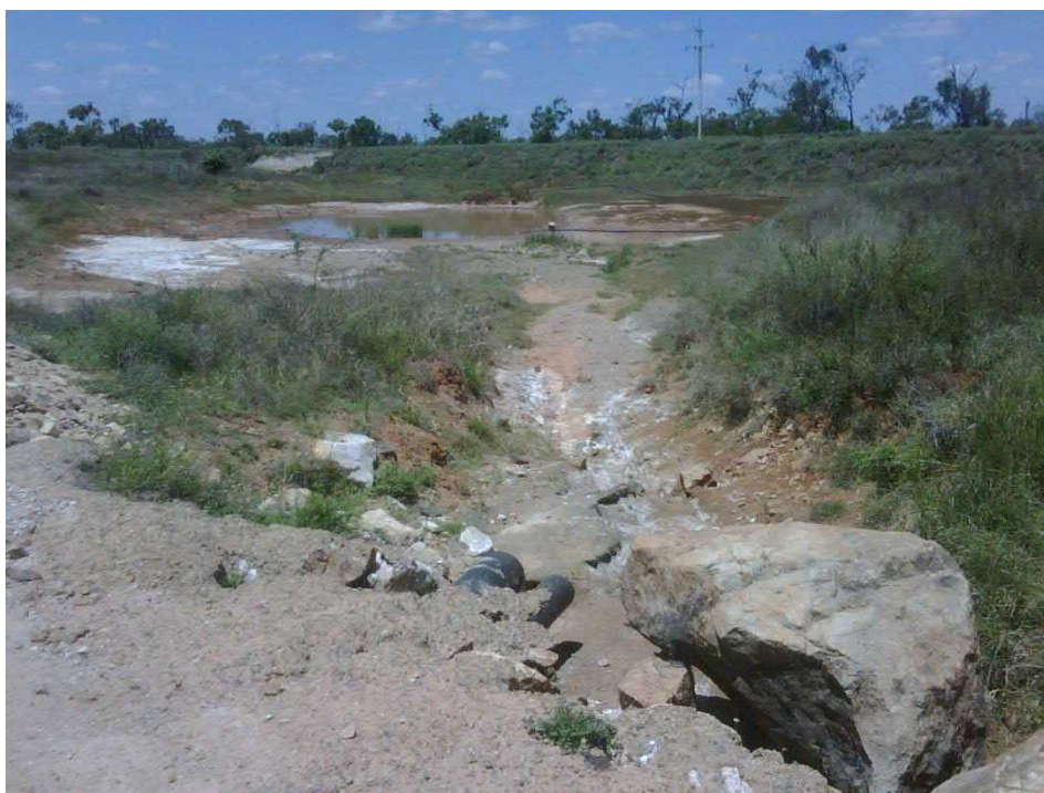
Mt Hope Extension Dam
