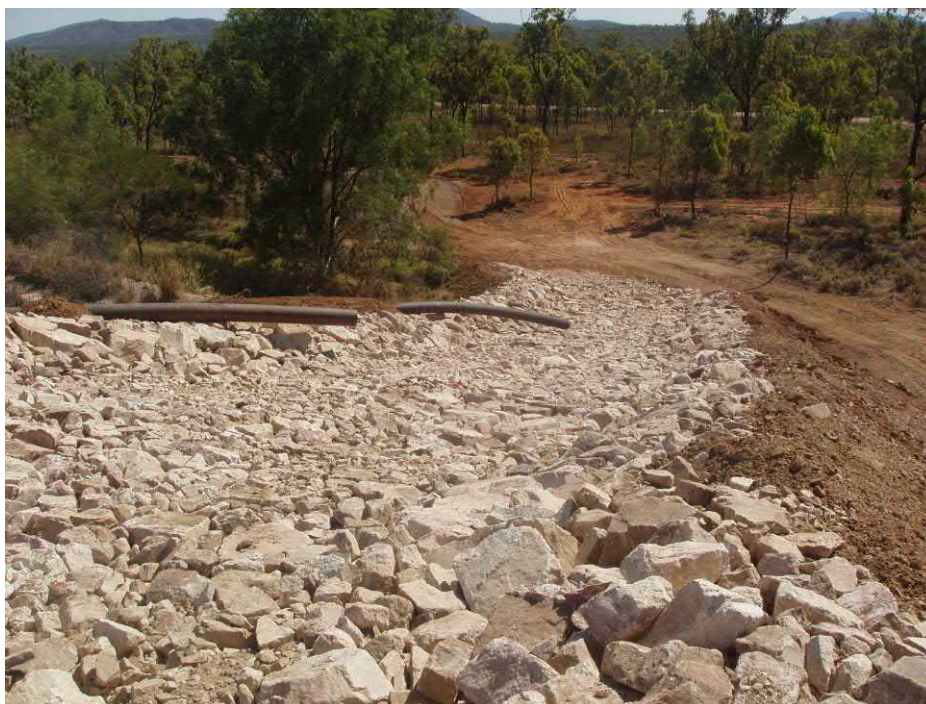
Southern Tailings Storage Facility Diversion
