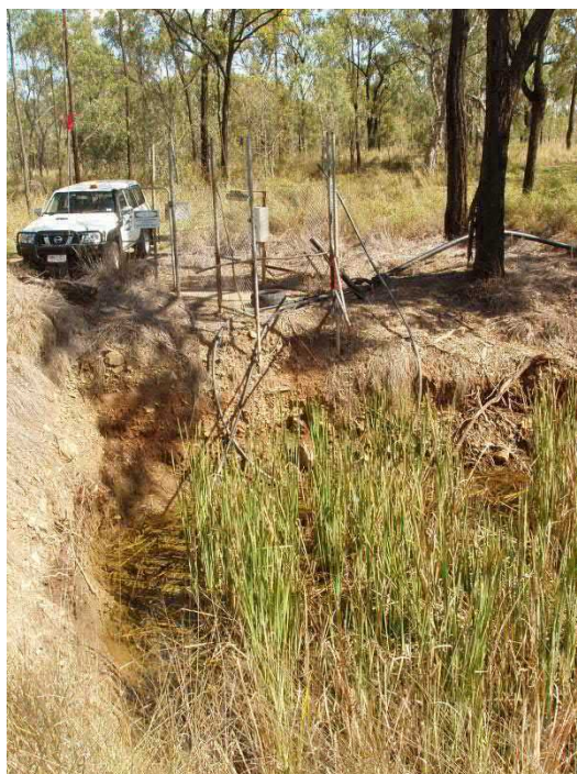
Settlement Dam Sump electric pump (submersible pump)
