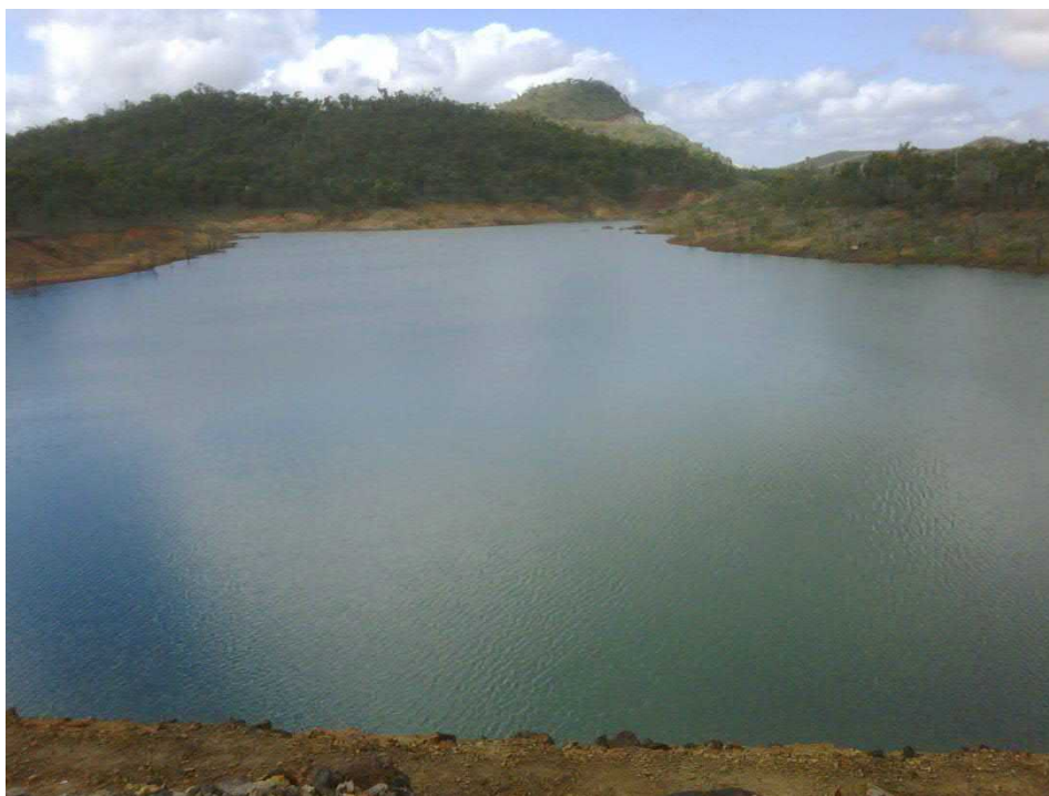
Raw Water Dam
