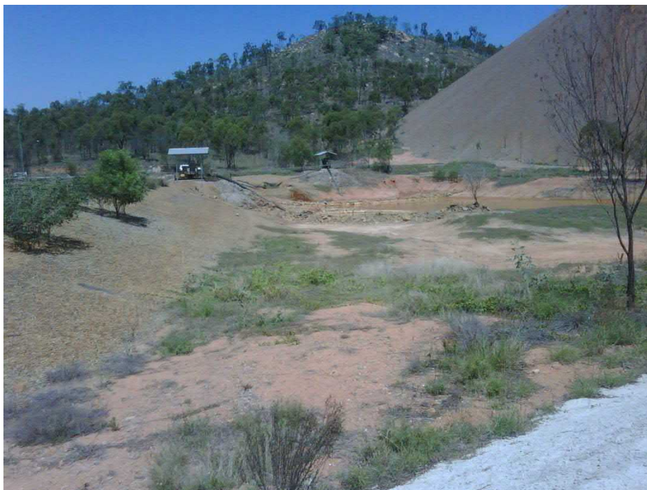
Plum Tree Creek Dam
