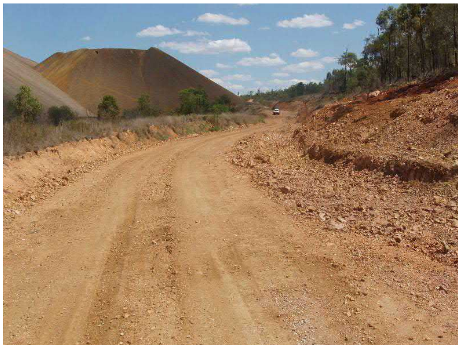
Plum Tree Creek Dam external catchment diversion channel
