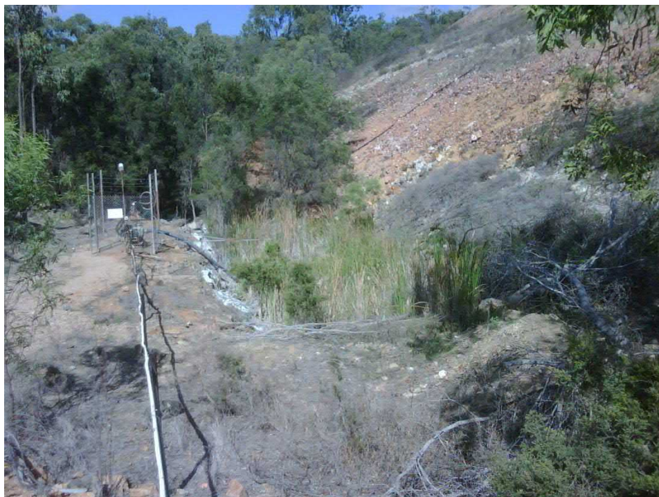
Raw Water Dam Sump
