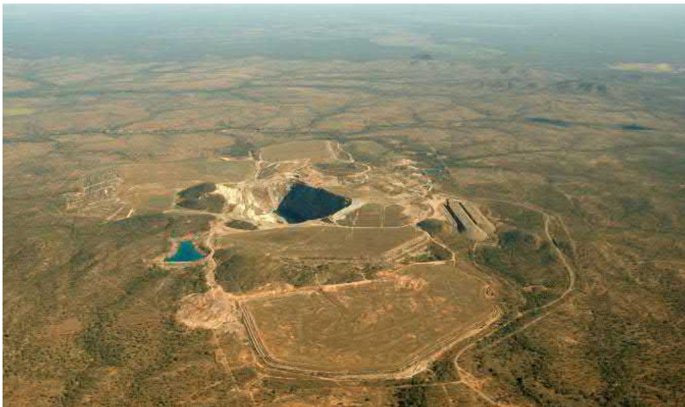
Figure 1.6: Landforms at Mt Leyshon Mine ~2005 (view to the south)
