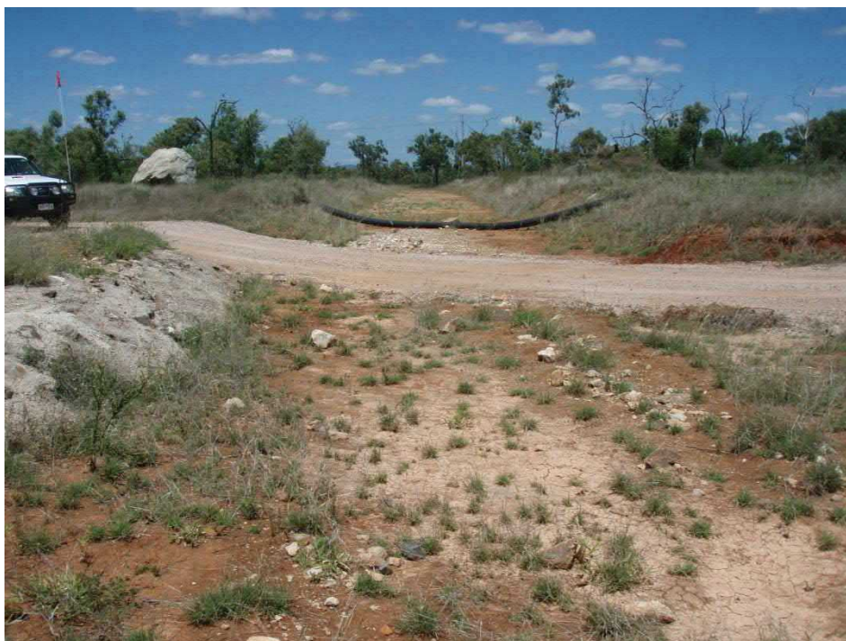
Diversion drain around western side of Mt Hope Extension Dam
