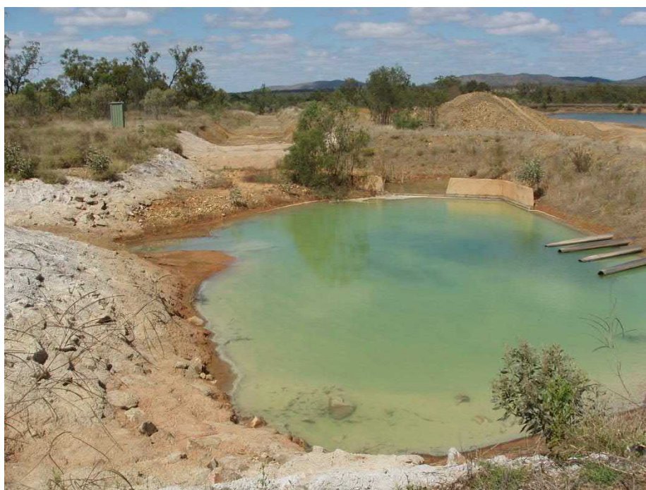
Settlement Dam high flow bypass facility
