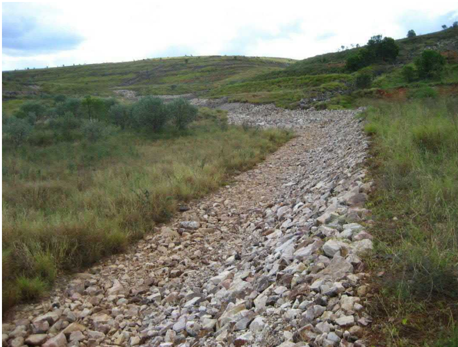
Mt Hope Dam high flow bypass facility
