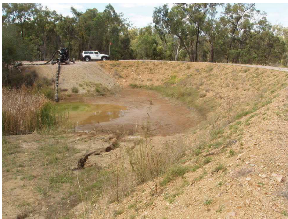
Flood protection levee around STD SW Sump
