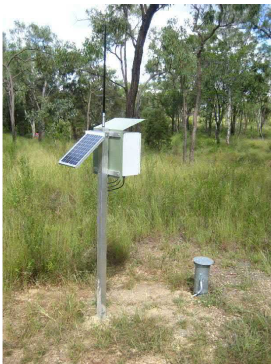
Typical monitoring bore automatic monitoring station
