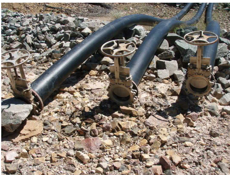
Supergene Stormwater Dam low flow bypass facility
