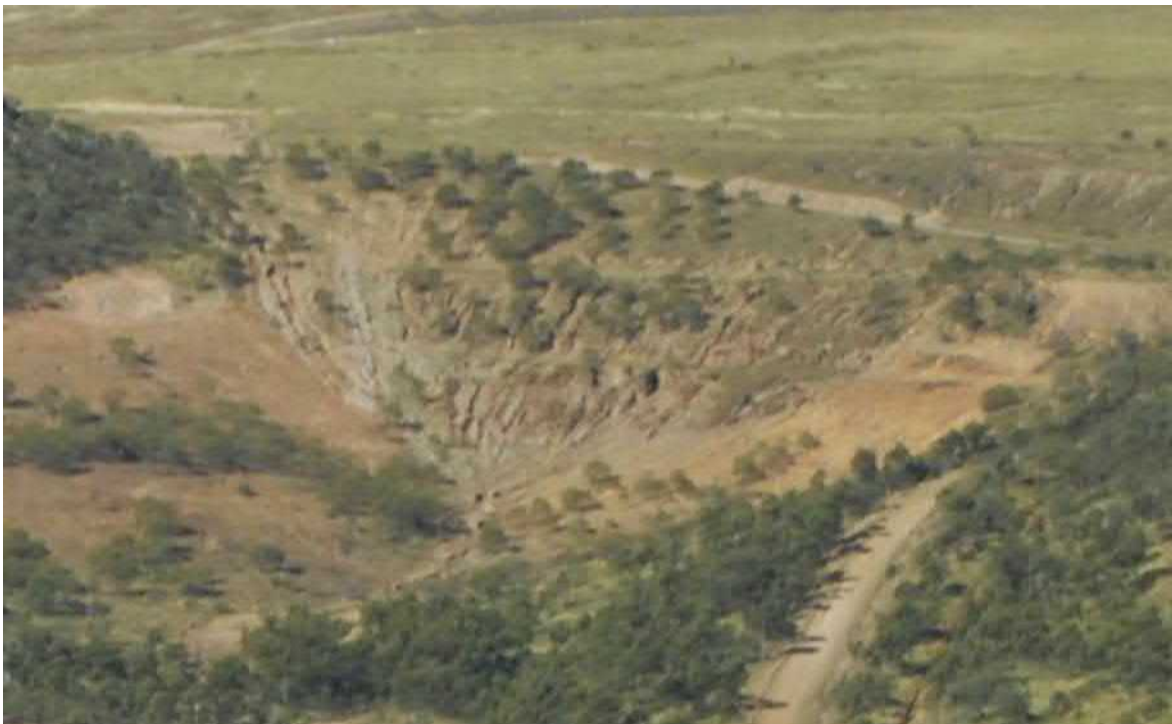
Figure 1.58: Western Section of Roche Hill prior to Rehabilitation Repair Works in 2017
