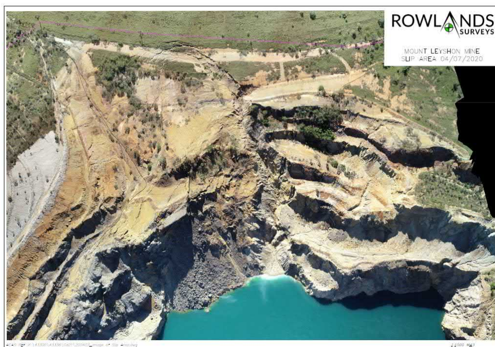
Figure 5.4: July 2020 Aerial Imagery of Open Pit North Wall Slope Failure Area
