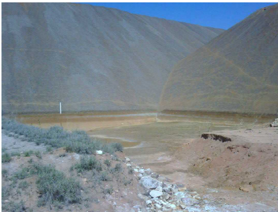
Upper Plum Tree Creek Dam
