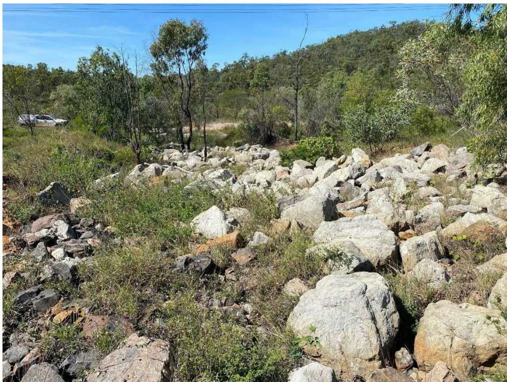
Figure 1.69: ONTSF Closure Spillway – Eastern Side of Landform
