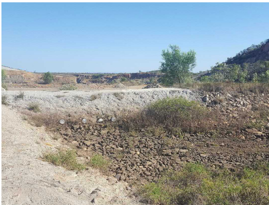
Eastern Waste Rock Dump low flow bypass facility
