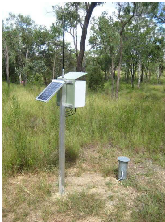
Typical monitoring bore automatic monitoring station
