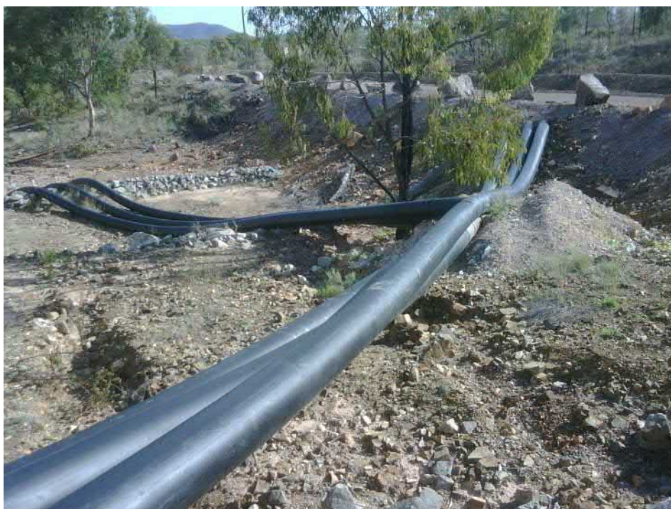
Supergene Stormwater Dam low flow bypass facility
