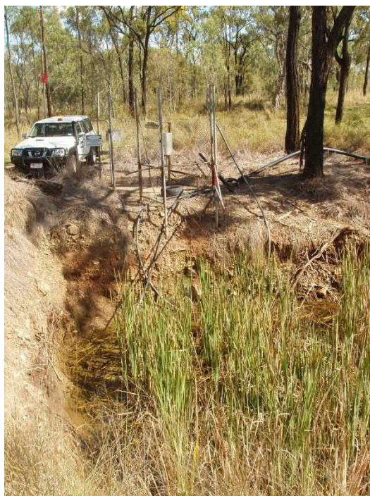
Settlement Dam Sump electric pump (submersible pump)
