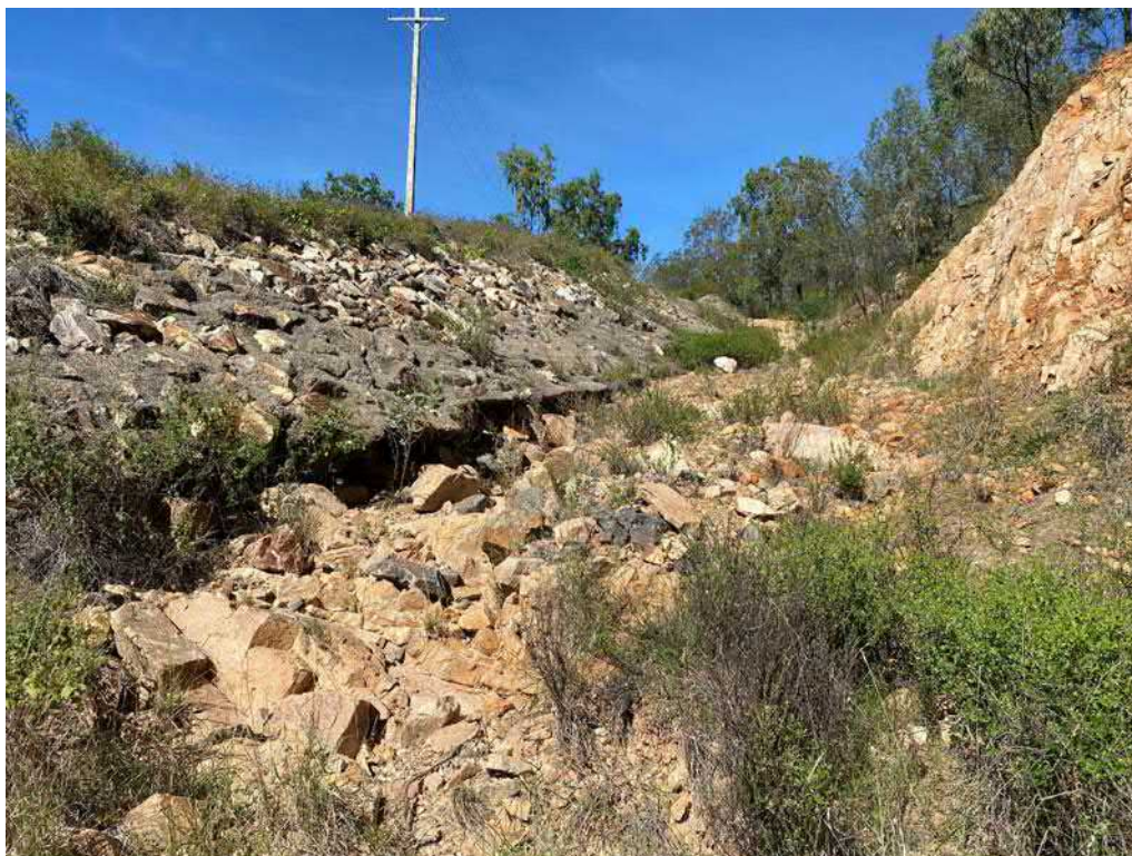
Figure 1.68: ONTSF Closure Spillway – Western Side of Landform
