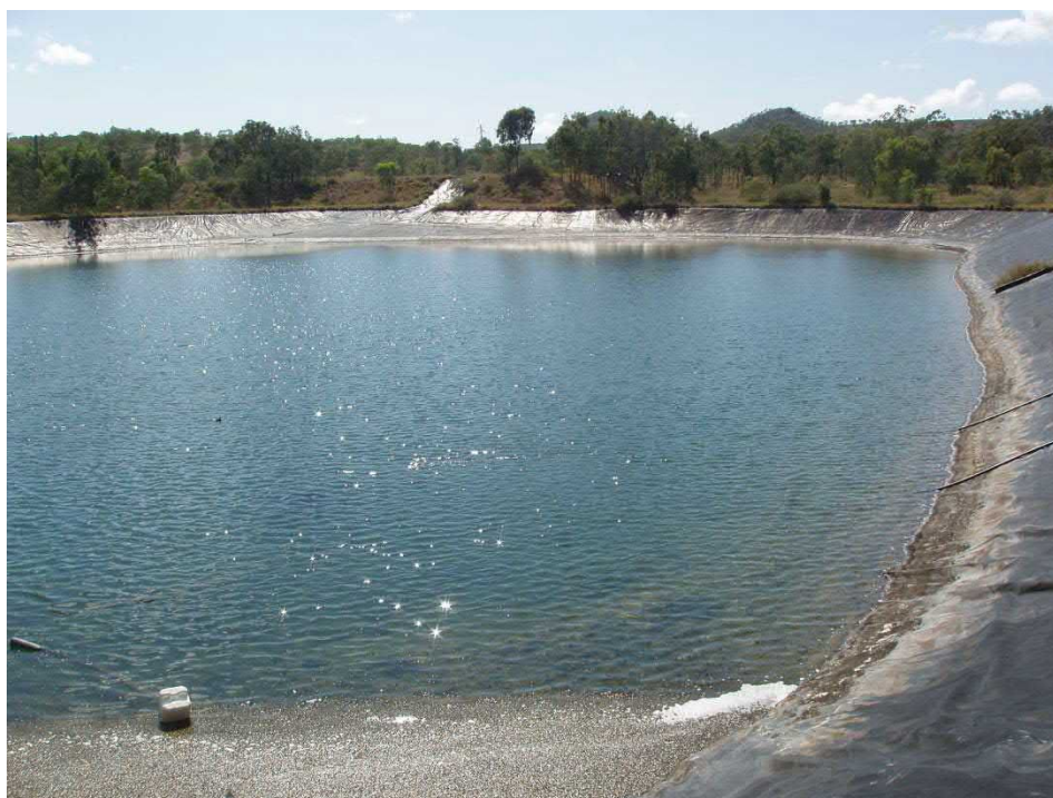
Stormwater Dam No. 2
