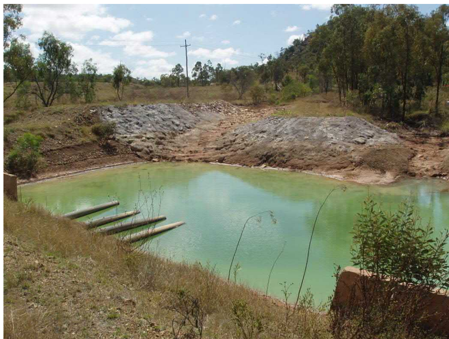
Settlement Dam high flow bypass facility
