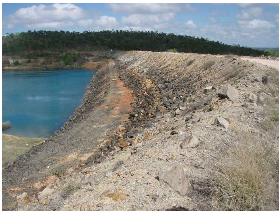
Raw Water Dam
