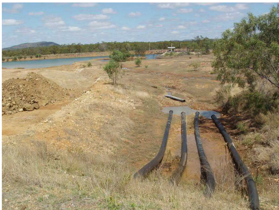
Settlement Dam high flow bypass facility
