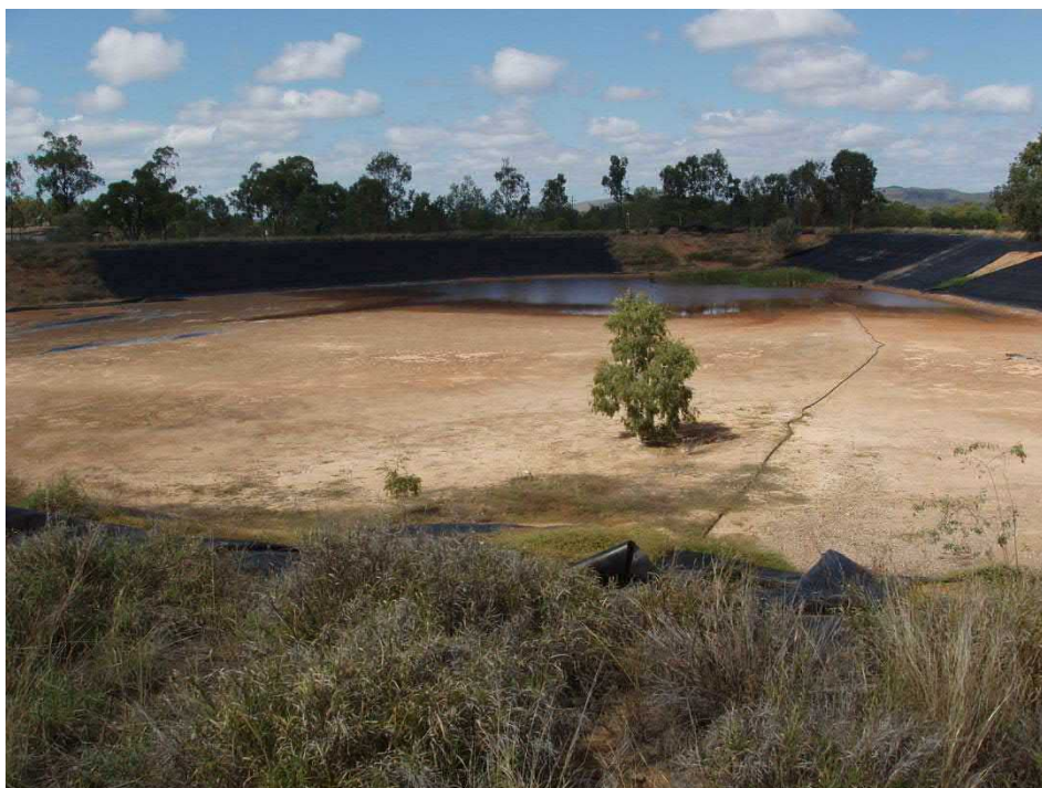
Stormwater Dam No. 1
