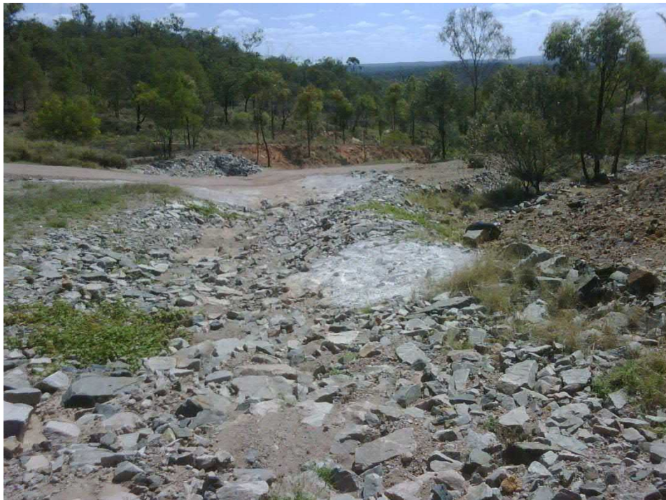
Drain on Roche Hill
