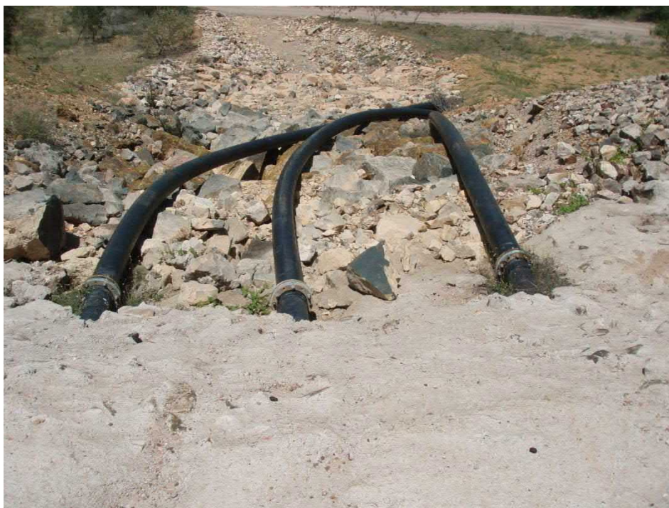
Supergene Stormwater Dam low flow bypass facility
