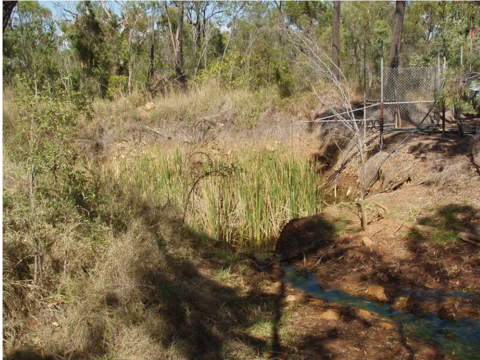
Settlement Dam Sump
