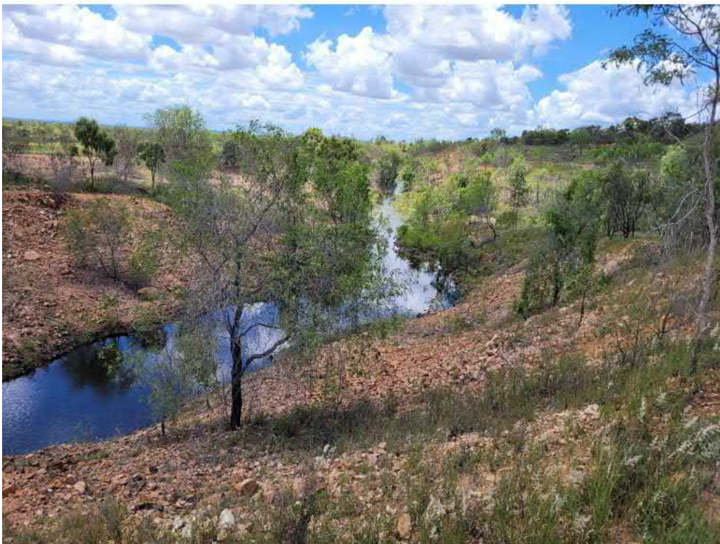
Figure 1.70: NNTSF Closure Spillway – Southern Side of Landform
