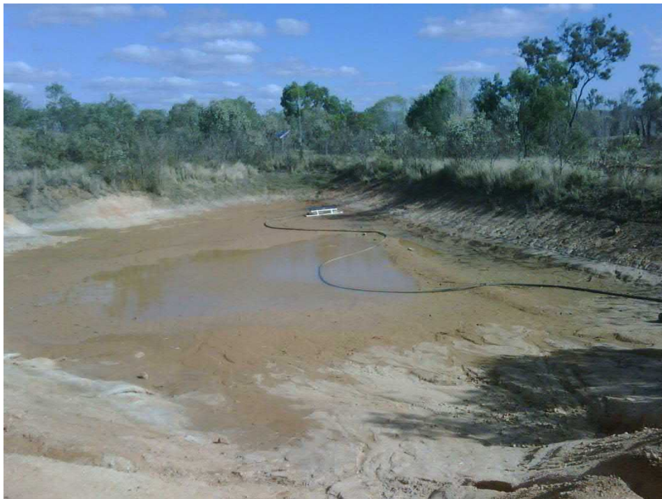
Western Scats Sump
