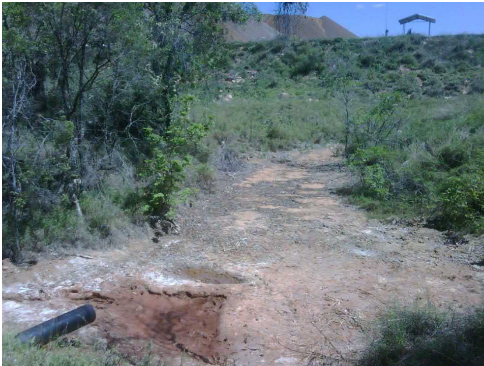
Plum Tree Creek Dam Sump
