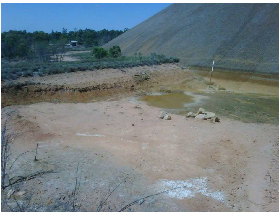
Upper Plum Tree Creek Dam
