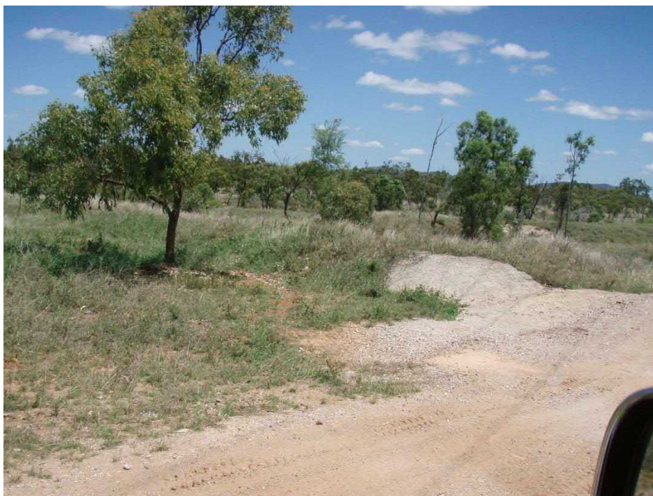
Diversion bund around eastern side of Mt Hope Extension Dam
