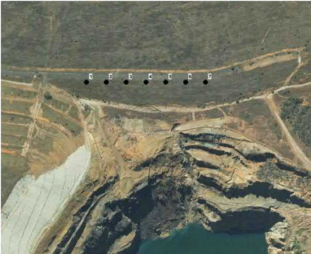
Figure 5.5: Movement Detection Survey Monuments for Open Pit North Wall Slope Failure Area
