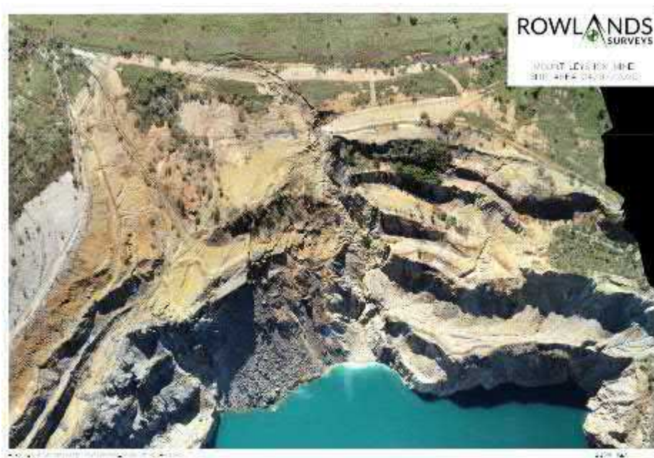
Figure 1.76: Slip Failure of Pit Void North Wall
