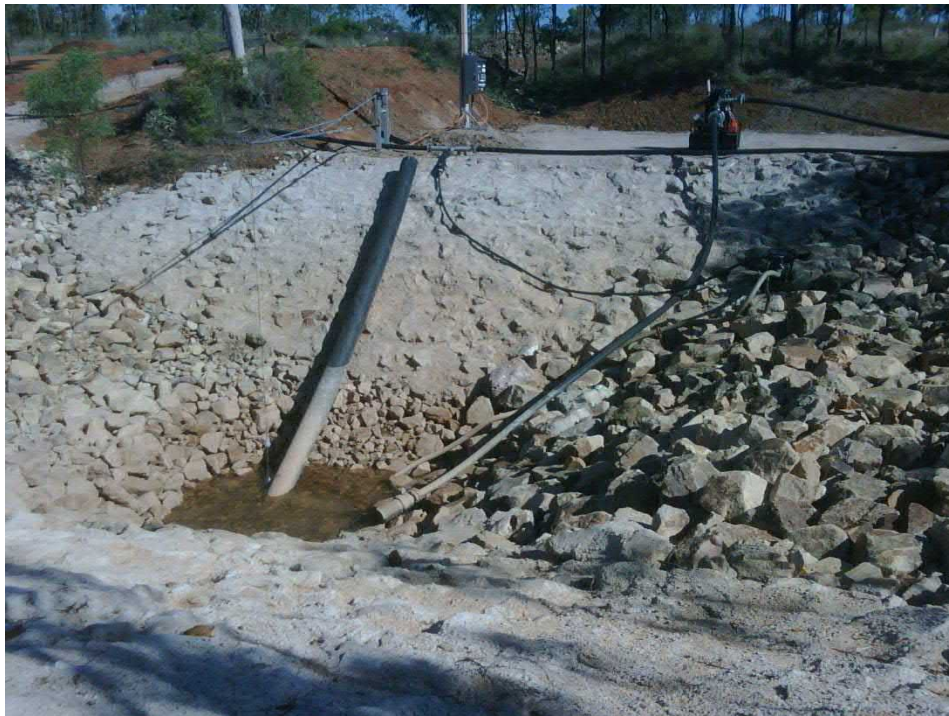
Mt Mawe Dam Sump
