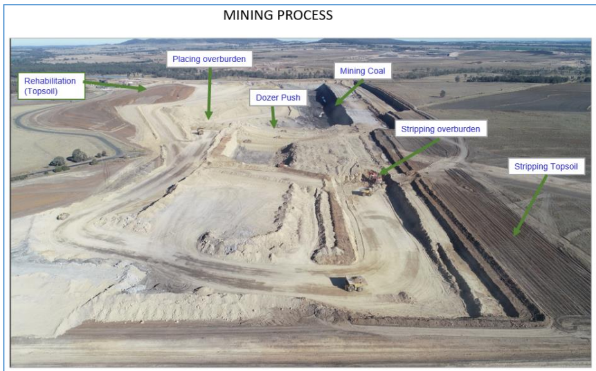
Figure 21 - Mining process from topsoil stripping to replacement.
