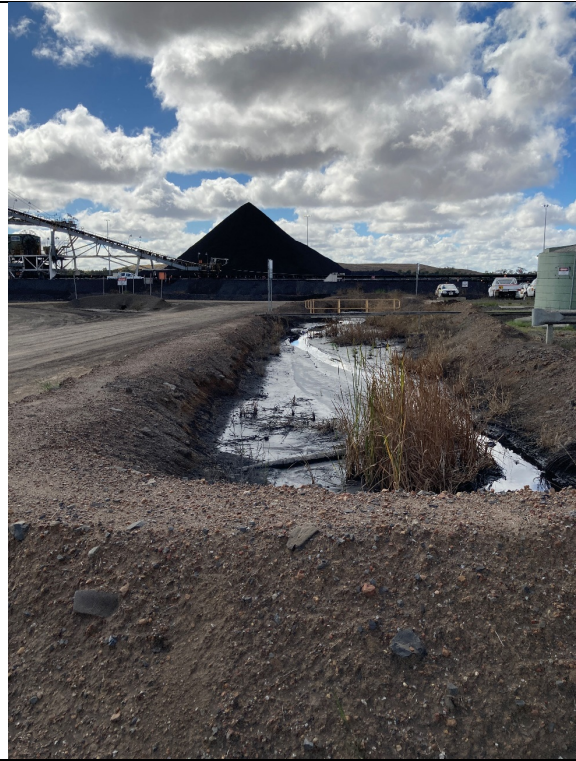
4. Stormwater drain near CHPP, large amount of coal fines visible
