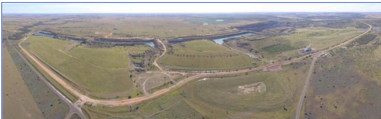
Figure 1-5 Existing rehabilitation at AB Pit (ML7459)
