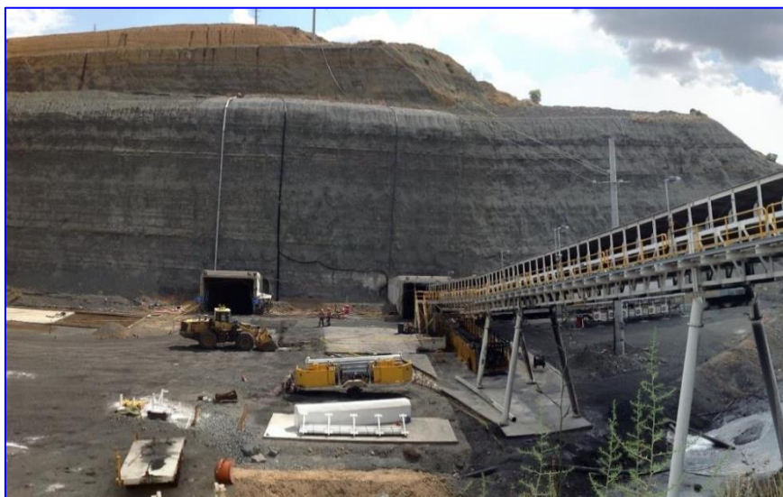
Figure 5-11 Entrances to the existing Ensham underground mine.
