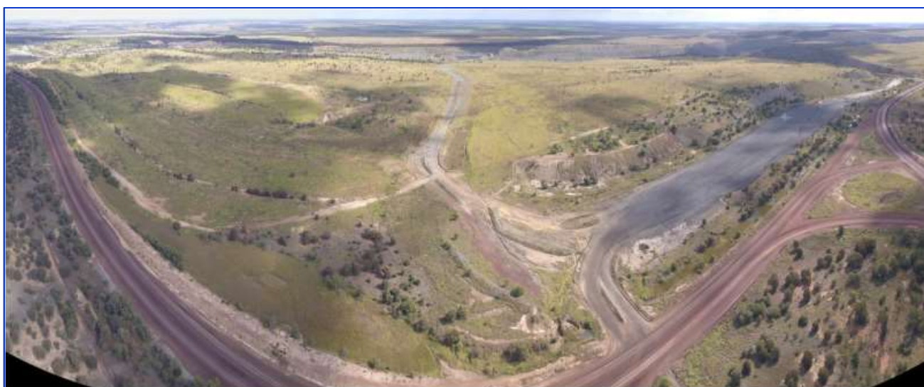
Figure 1-6 Existing rehabilitation at CDE Pit (ML7459)
