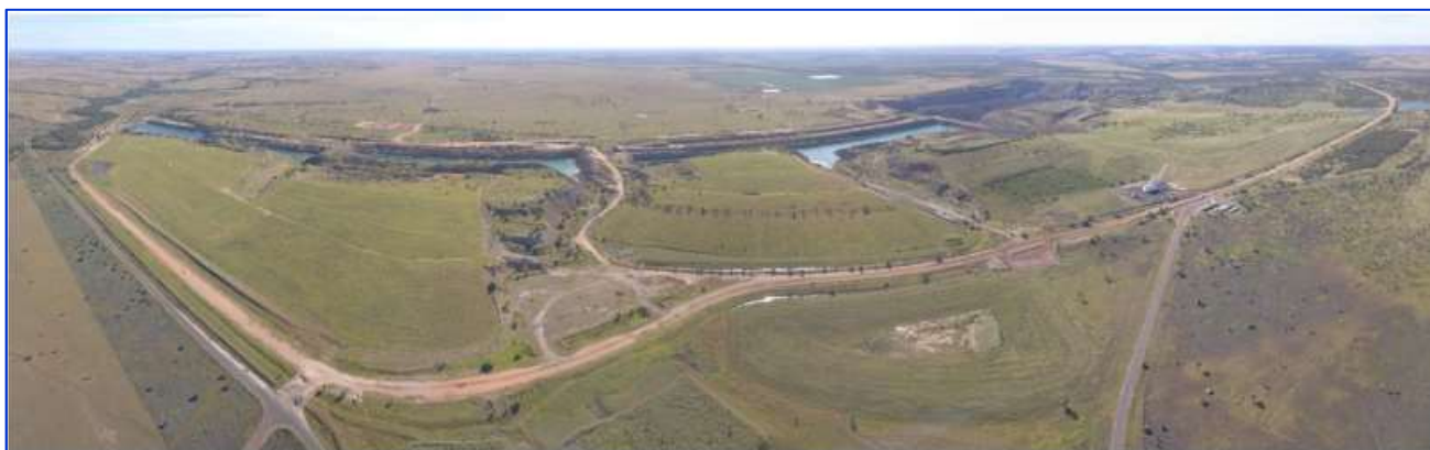
Figure 1-5 Existing rehabilitation at AB Pit (ML7459)
