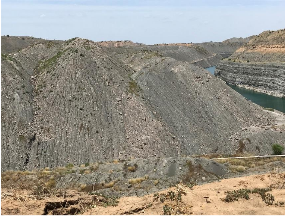
Photo 4-1: Low-wall spoil, mostly Permian materials showing signs of erosion
