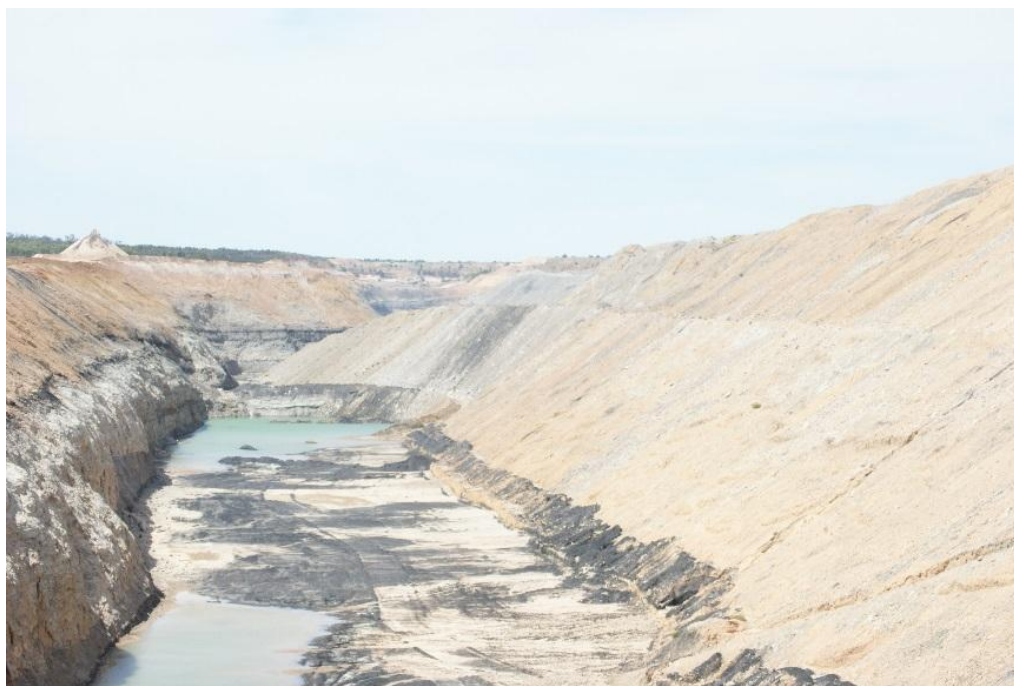
Photo 4-11: Tertiary Spoil Y-pit
