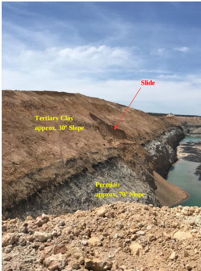
Photo 4-5: Yongala (Y-pit), weathered Permian overlain by weathered Tertiary material, with typical Tertiary failure
