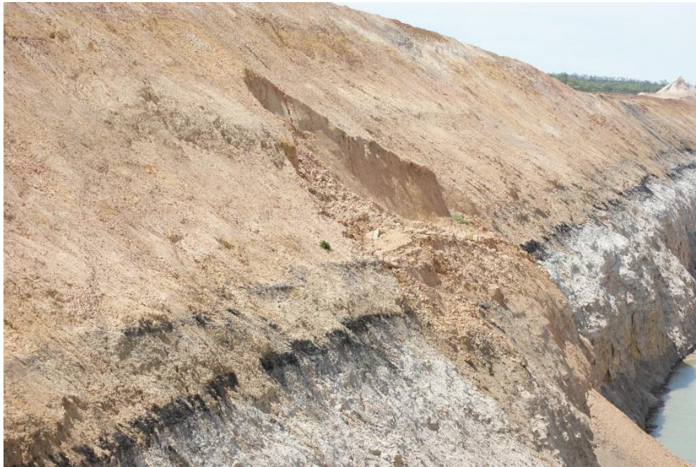
Photo 4-12: Instability in Tertiary Spoil Overlying Weathered Permian Material in Y-pit
