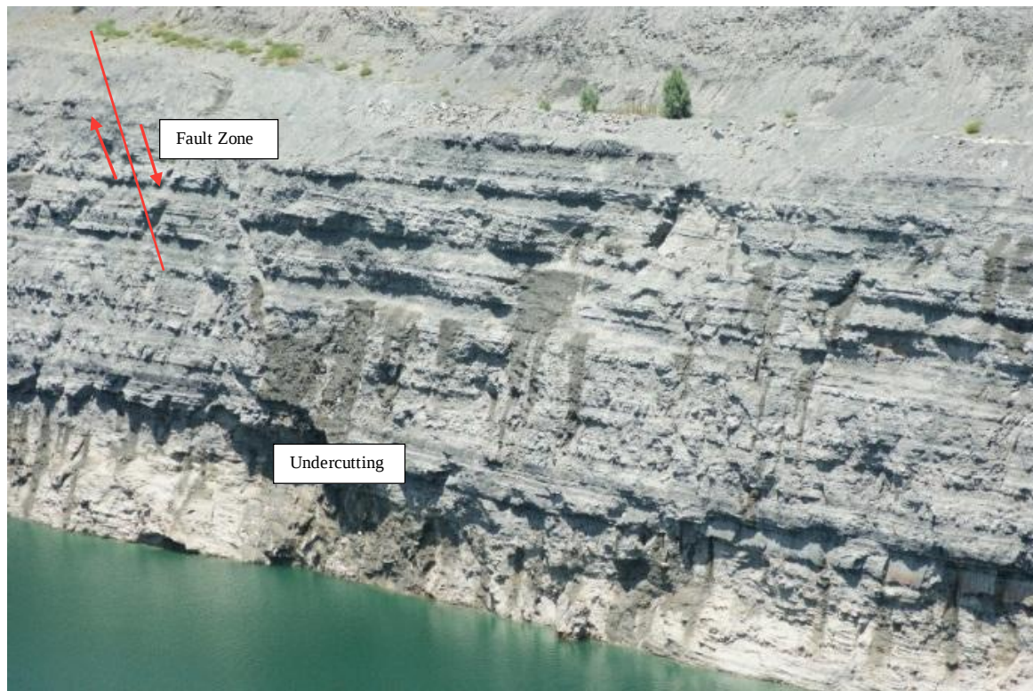
Photo 4-9: Fault in B-pit Highwall
