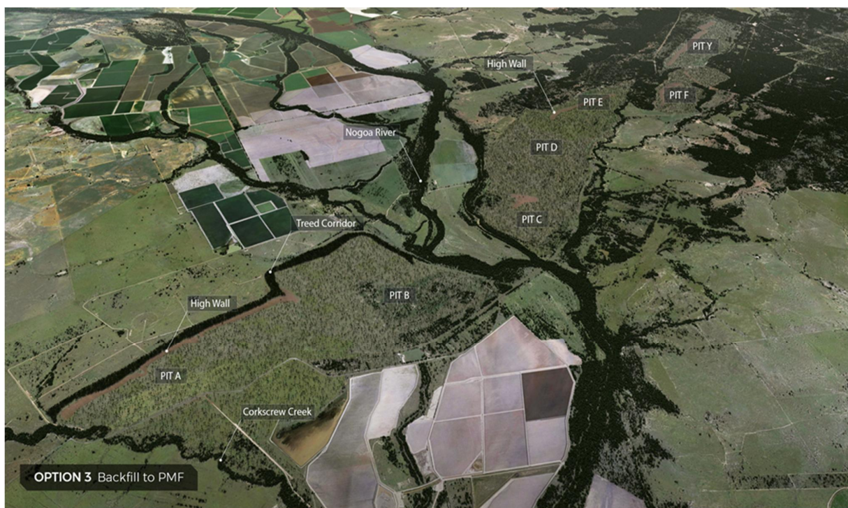
Figure 3-4: Backfill to PMF
