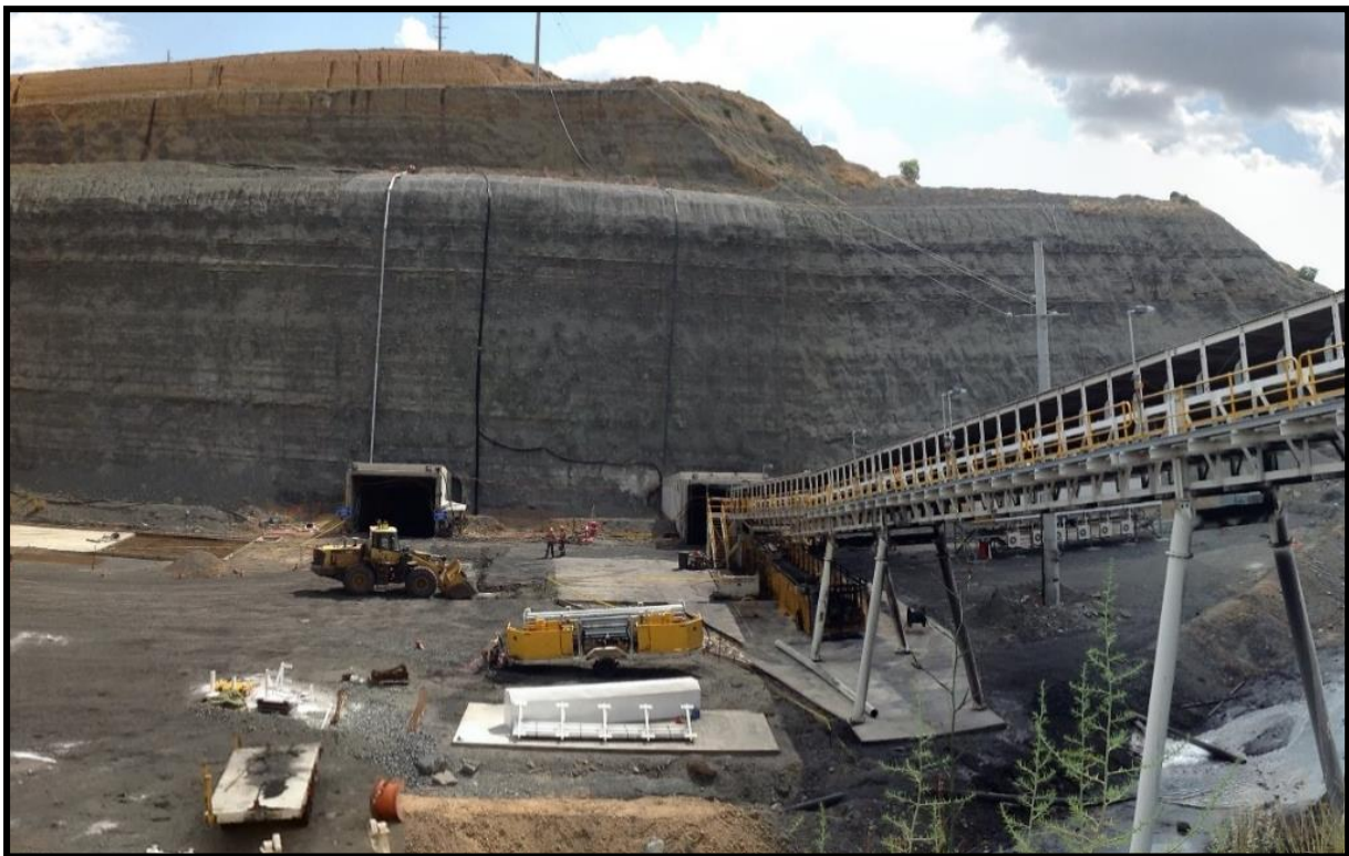
Figure 2. Access to the Underground Workings from Ramp 3
