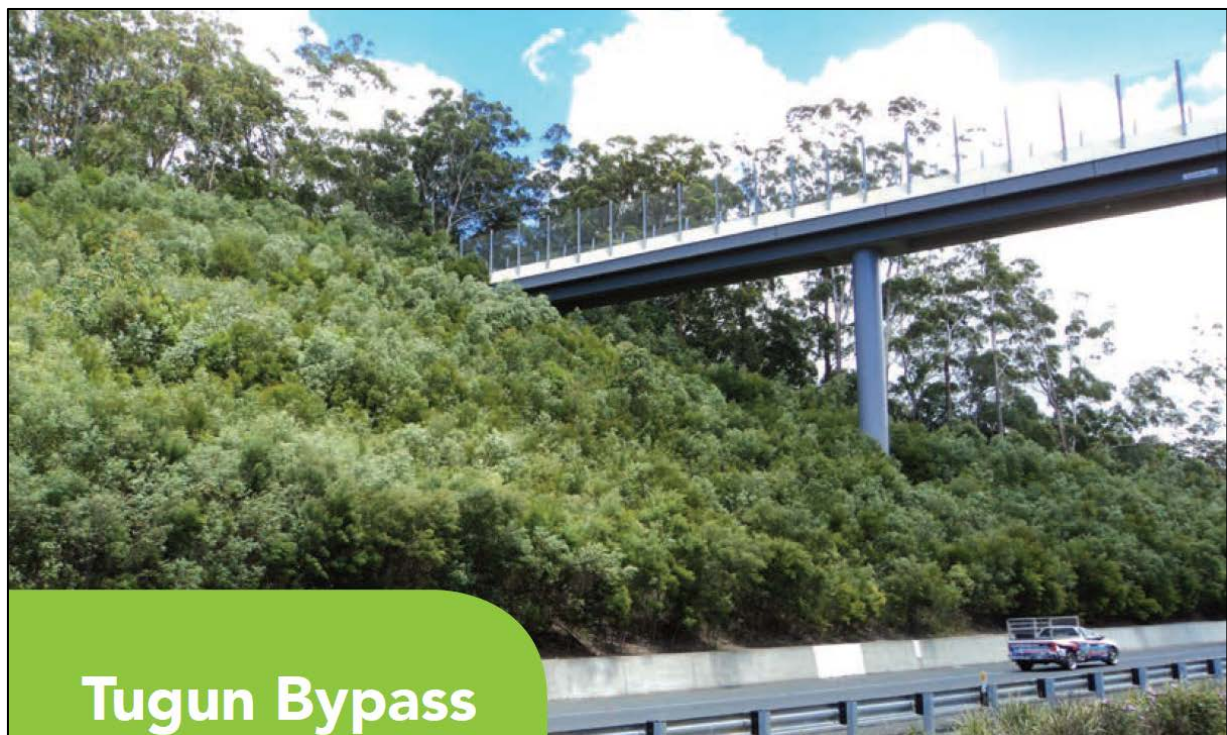
Figure 18 Tugun Bypass slope stabilisation with hydro mulching (February 2012)
