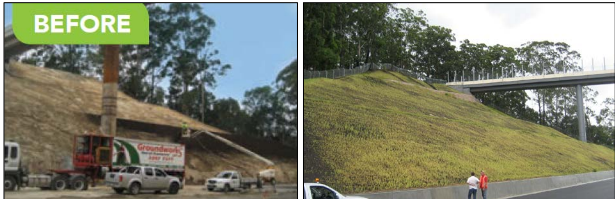
Figure 17 Tugun Bypass - Amelioration of fresh rock slope and post application (April 2008)
