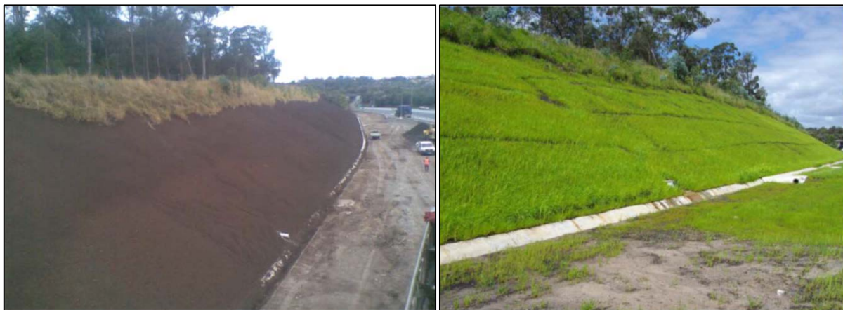
Figure 15 Centennial Motorway - Amelioration of fresh rock slope and two months post application
