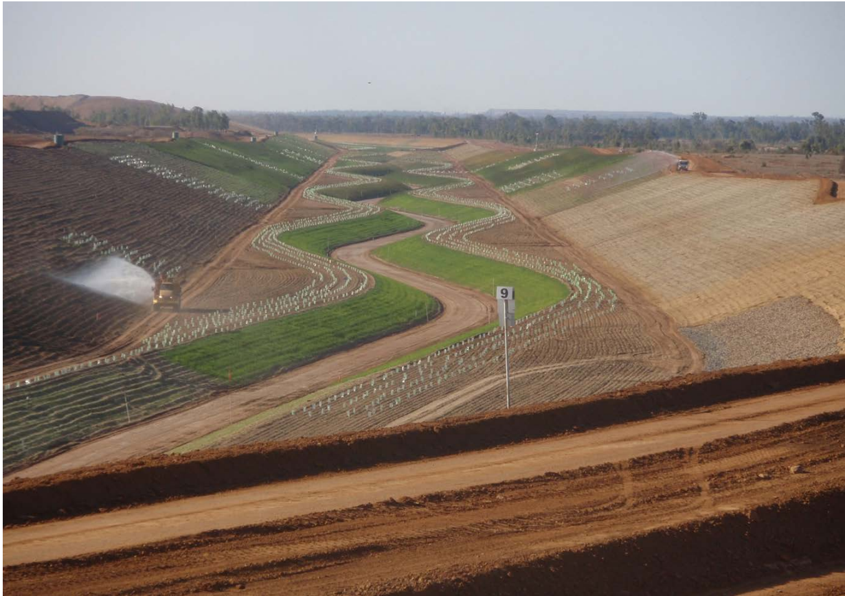
Figure 14 Slope preparation and application of hydro mulching at Blackwater Creek
