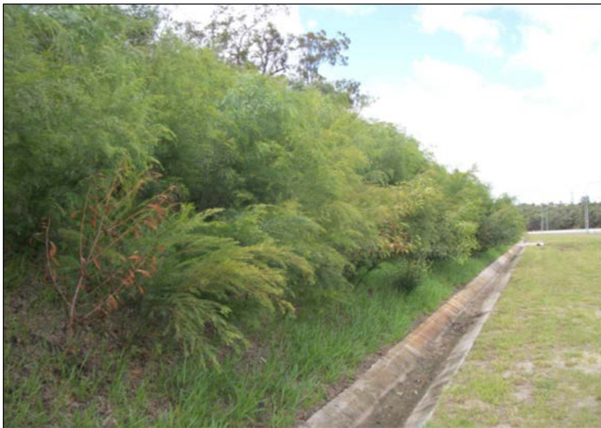
Figure 16 The same Centennial Motorway fresh rock slope after 3yrs
