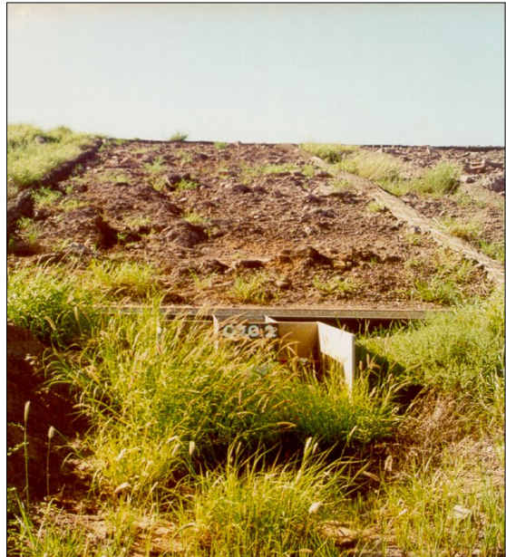
Figure 9: Topsoil bare plot
