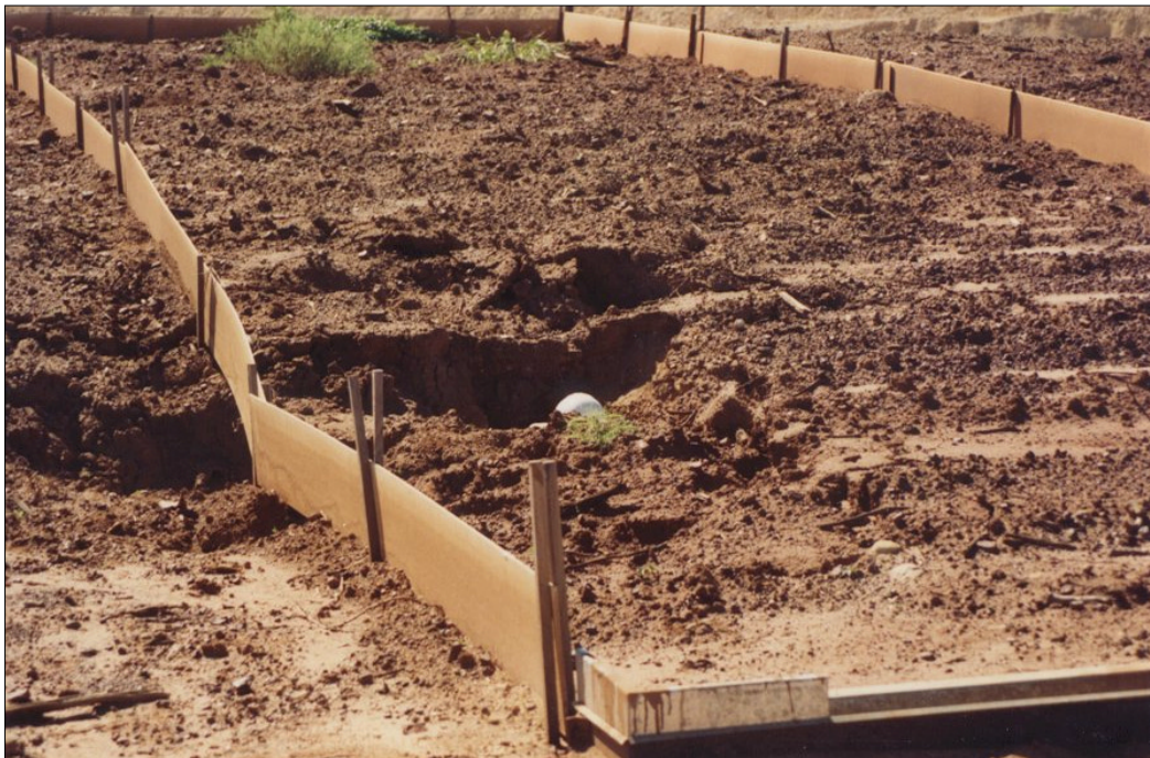
Photo 11: Slumping on the 10% topsoil plot, 1994.
