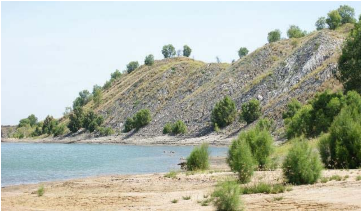
Figure 5-1: A Pit Low wall – Permian dominated side cast spoil
