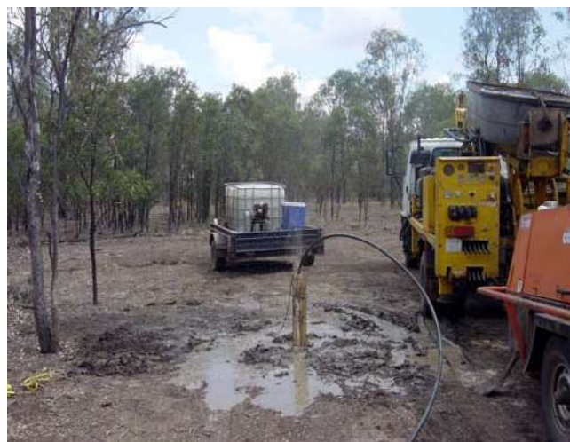
Plate 1: Drilling with foam and airlift development of monitoring bore
