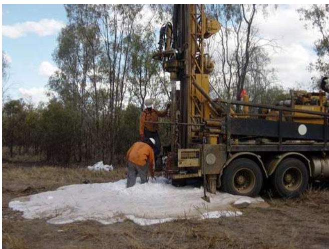
Plate 1: Drilling with foam and airlift development of monitoring bore
