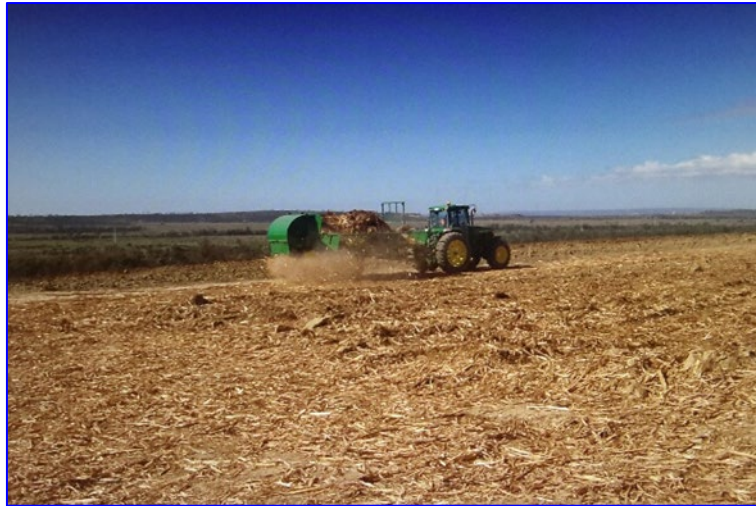
Figure 5-12 Spreading hay mulch for erosion control in rehabilitation at Ensham
