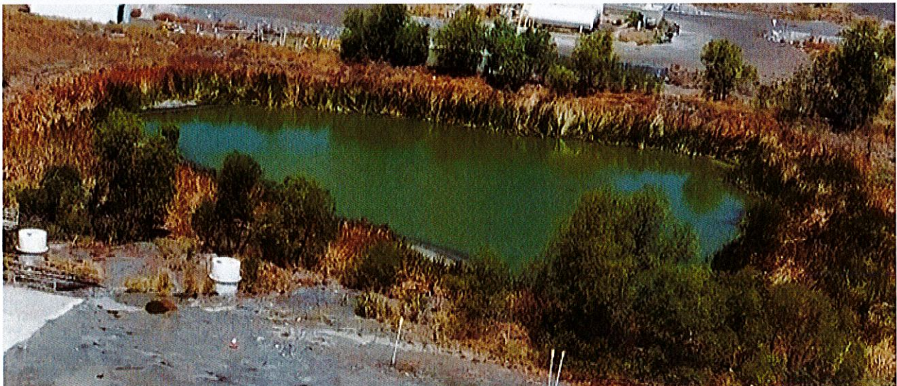
Workshop Area Dam
