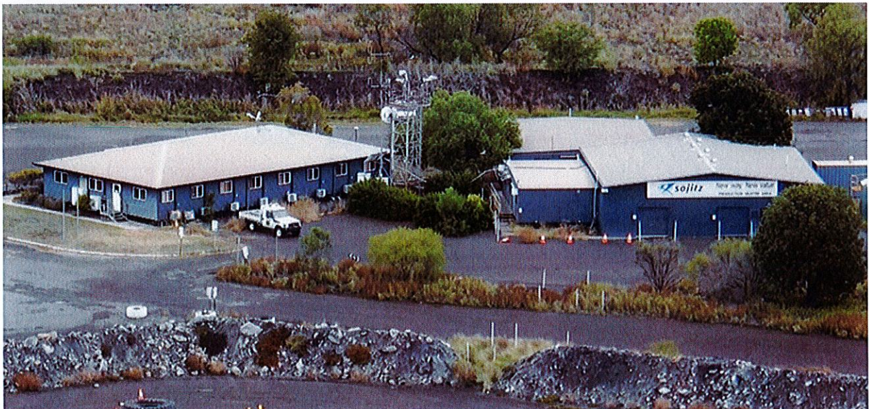
Site Administration and Muster Shed
