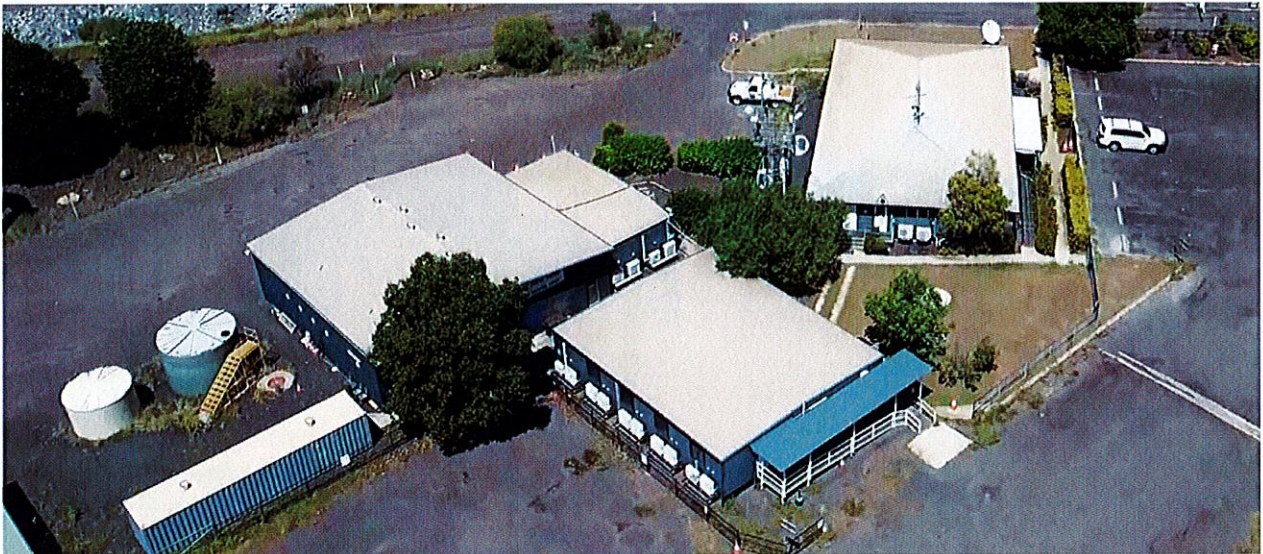
Site Administration and Muster Shed
