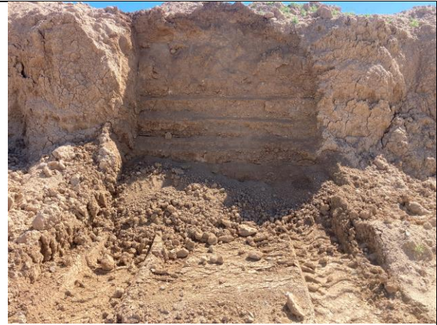
Figure 8: Dry Tails Vertical Face
