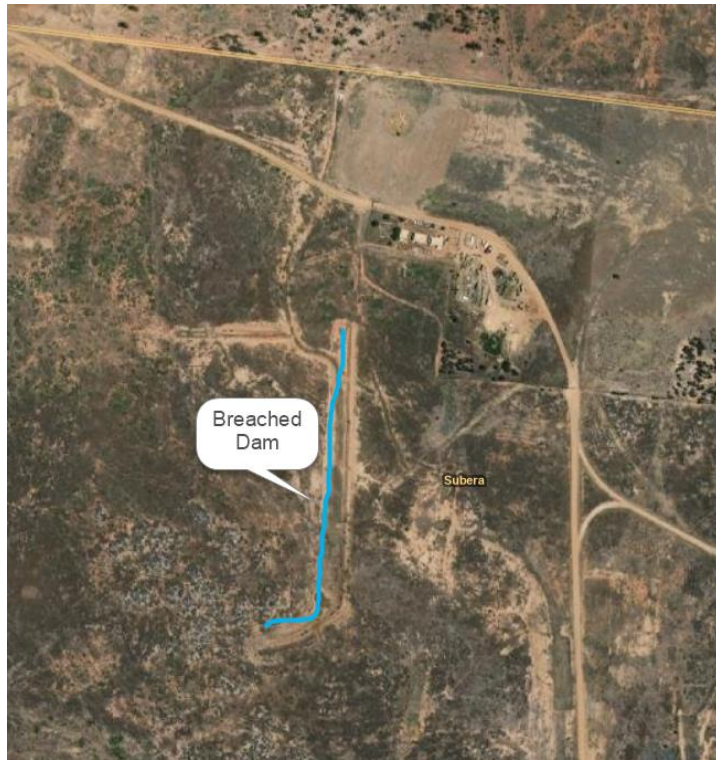
Figure 10: Breached Dam – Others
