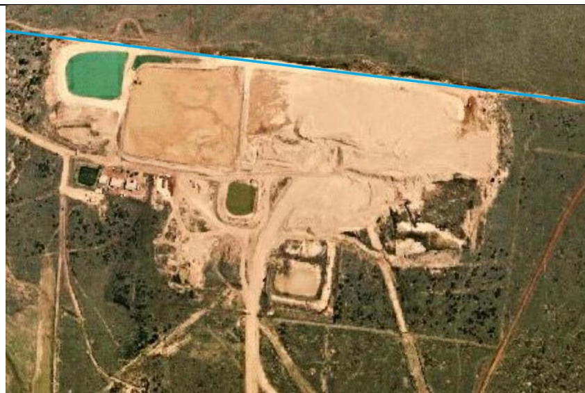
Figure 14: Main Dam Site/Rejects Hill 2001 – note absence of topsoil stockpiles
