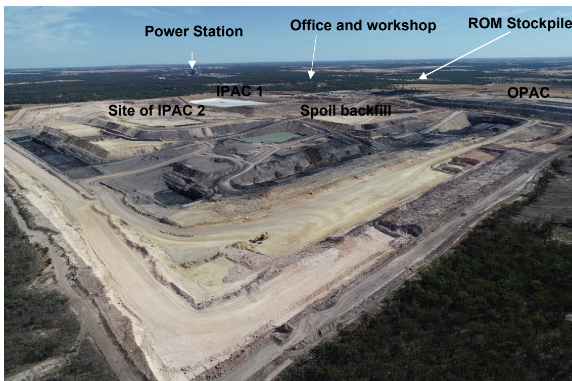
Figure 1 Mine Pit Looking Northwest to Kogan Creek PS March 2019
