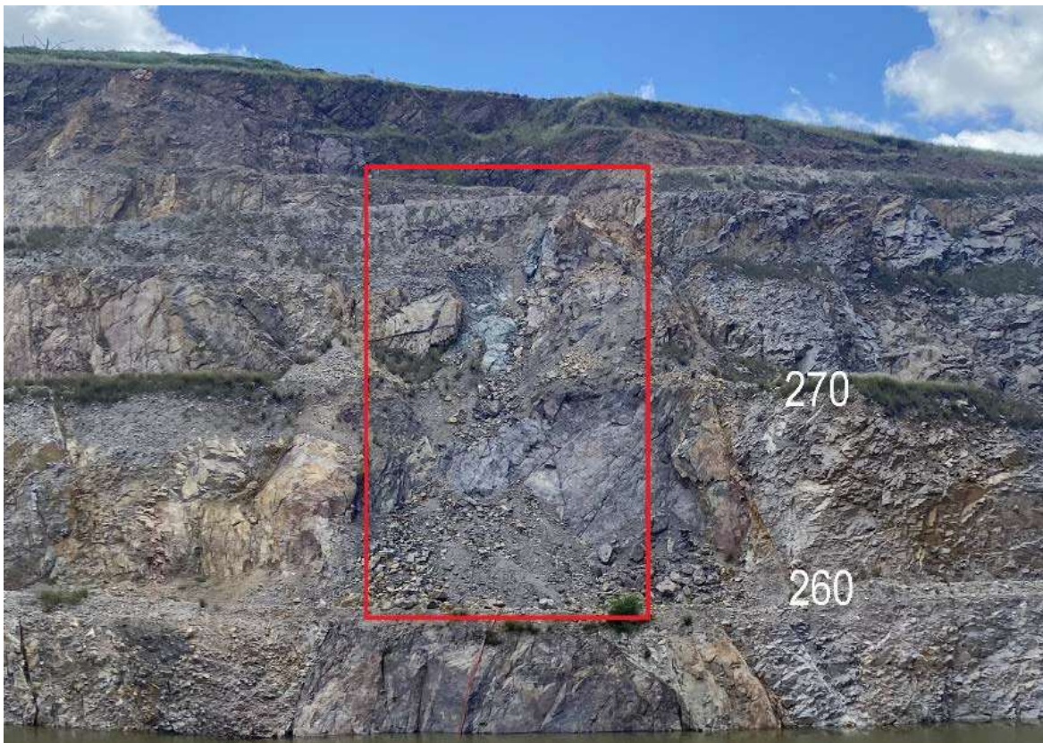
(b) Wedge sliding of unweathered limestone along two discontinuities dipping out of the east wall.
