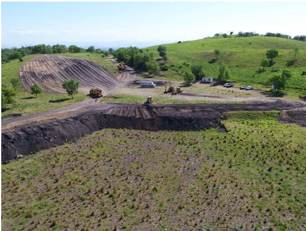
Oakleigh East – Tailings Dam Capping Operations
