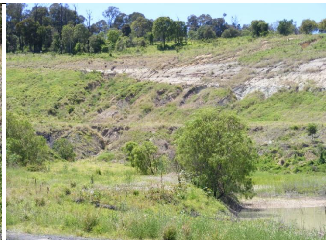
Figure 3 South-west batter of Oakleigh North void. Vegetation has not been able to establish and severe gullies have formed.
