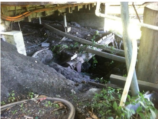
Photograph 81 – Old underground tunnel entrance (15/11/11).
