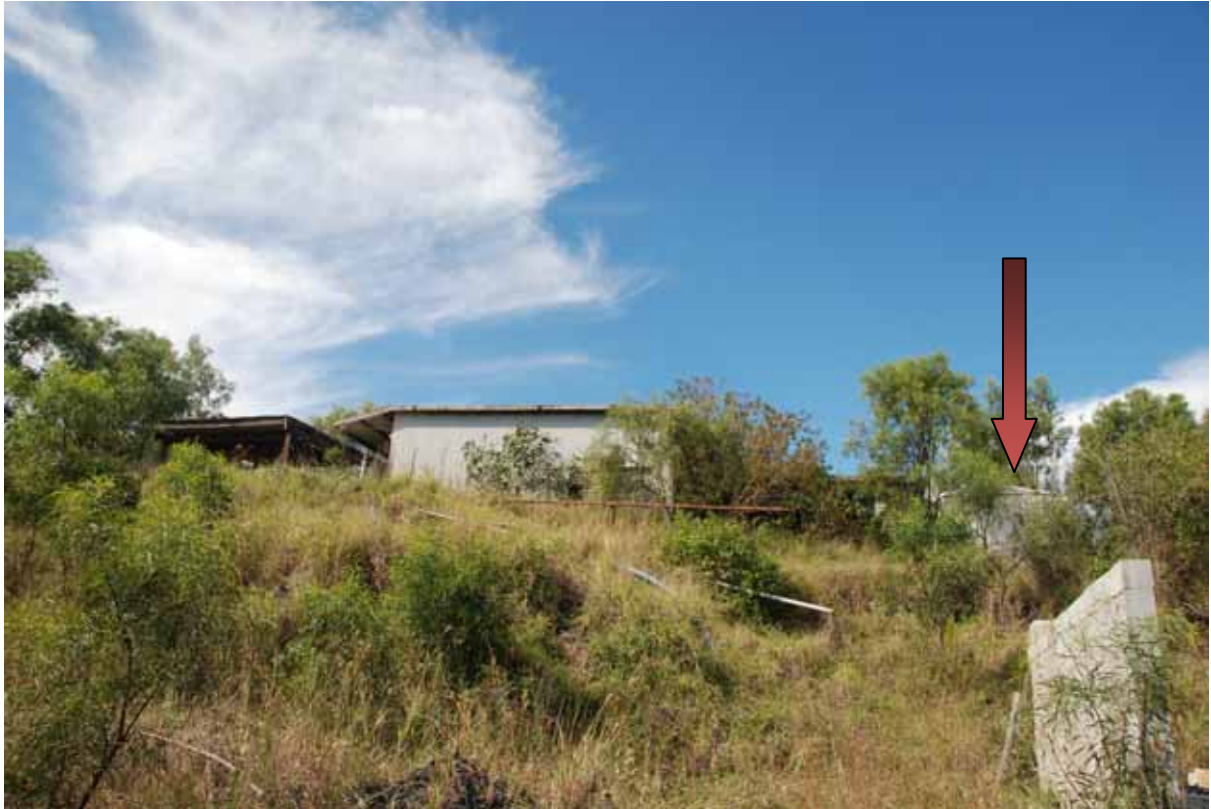
B8-5 Shed behind Repair Room
