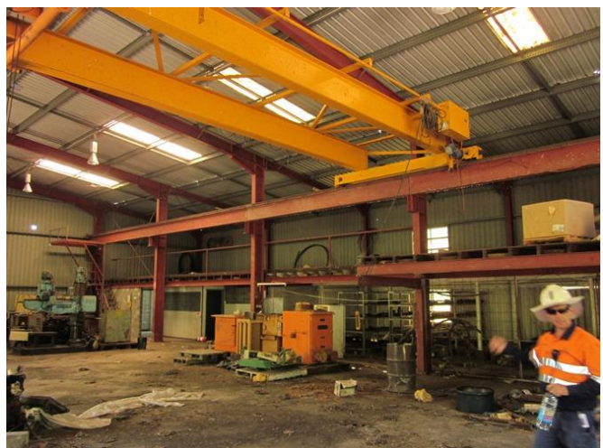
Photograph 64 – Operations workshop view from north to south (15/11/11).
