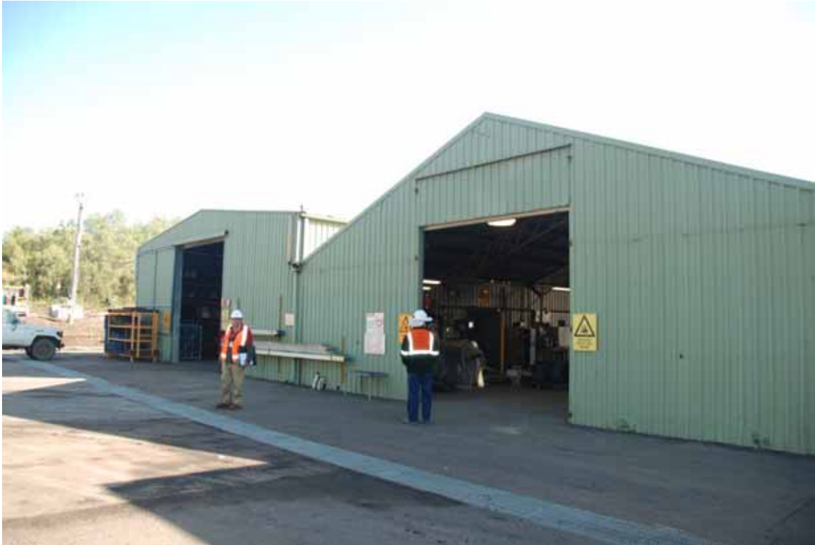
1910 Store Shed/1920 Workshop
