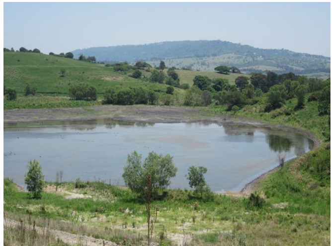
Photograph 60 – Zoomed in shot of the tailings dam (15/11/11).
