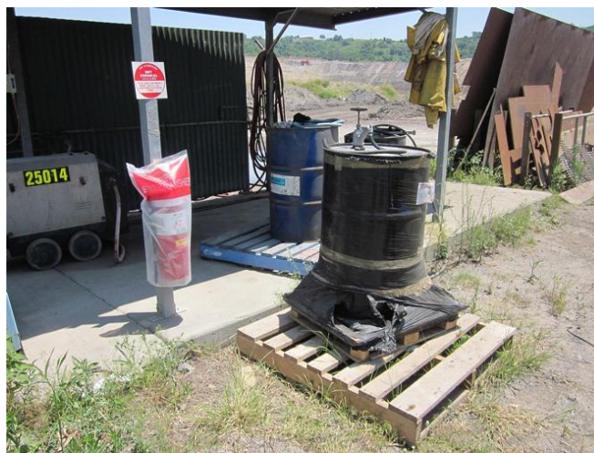
Photograph 14 – Fuel drums stored on wooden pallets, and storage of materials near to the wash down bay area (15/11/11).
