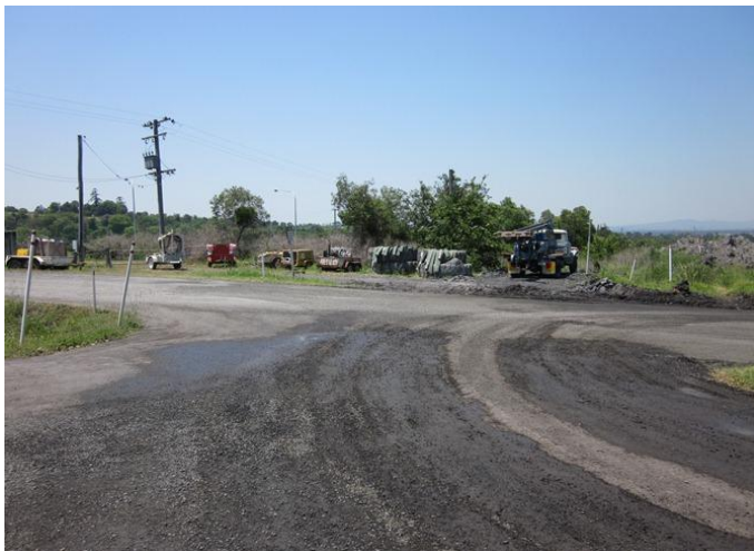
Photograph 1 – Site entrance road showing machinery storage area (15/11/11).
