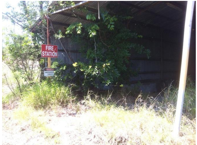
Photograph 78 – Fire station building from the underground era (15/11/11).
