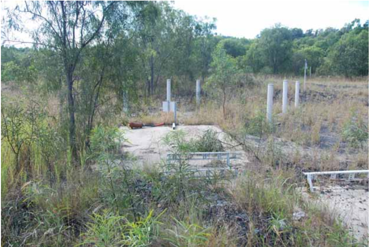
B5 – Concrete Block NO.2
