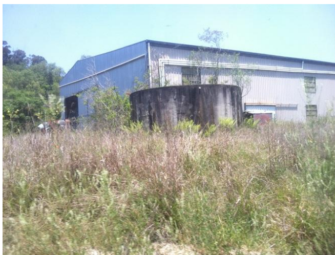
Photograph 74 – View from eastern side of the Operations workshop with guttering and concrete water tank collecting rainwater (15/11/11).
