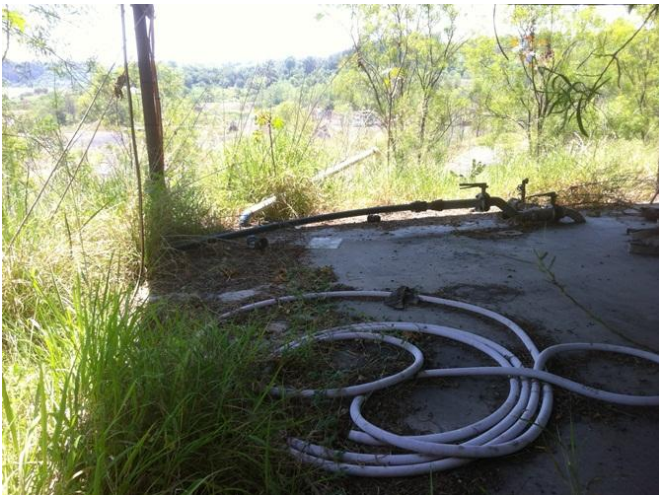
Photograph 79 – Pipe work and hosing related to the fire fighting water supply onsite (15/11/11).
