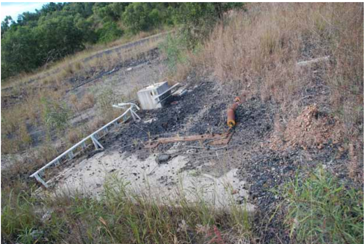
B5 – Concrete Block NO.3
