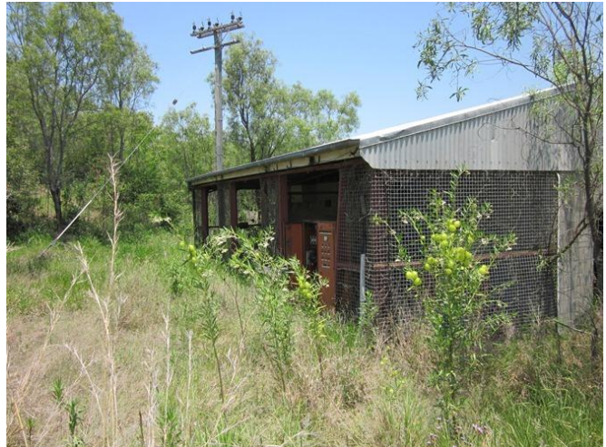
Photograph 50 – Old garage / workshop area (15/11/11).
