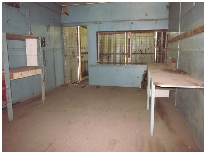
Photograph 52 – Inside the old house with walls constructed of potential asbestos containing materials (15/11/11).
