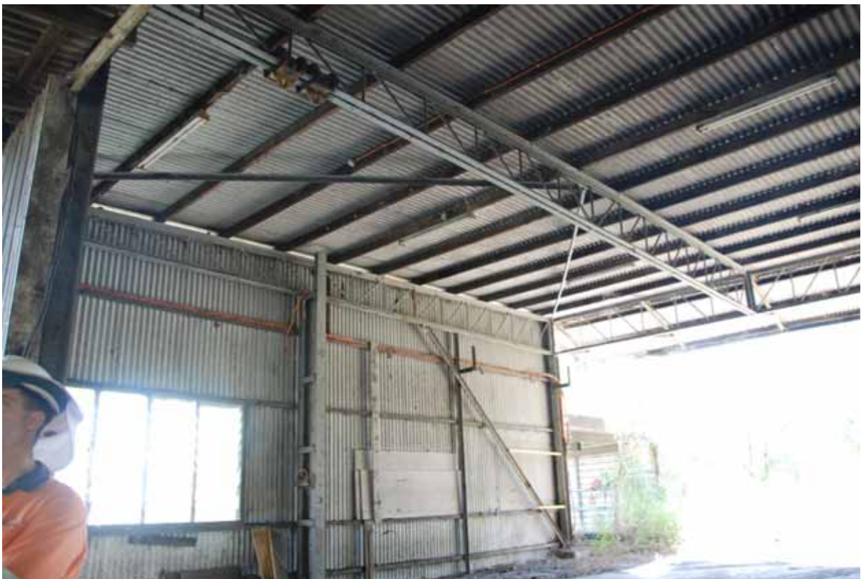
B8 - 1 Repair Room
