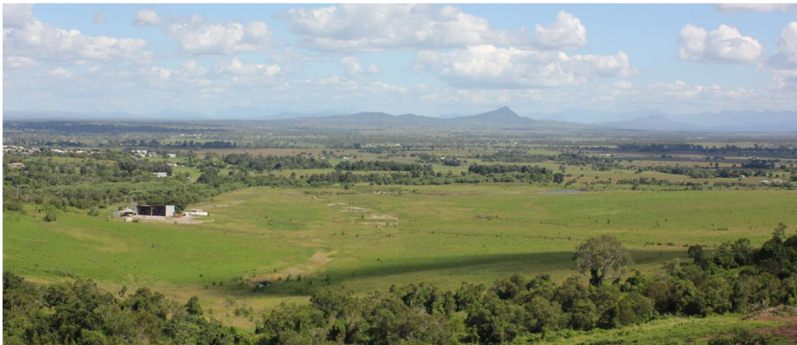
Figure 16: Oakleigh West: Post-rehabilitation—established grazing PMLU (2017; note retained infrastructure)
