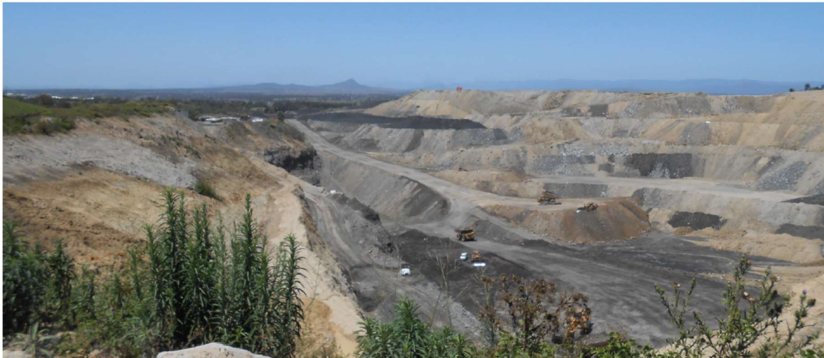
Figure 15: Oakleigh West: pre-rehabilitation—pit depth of approximately 90 m (2012)
