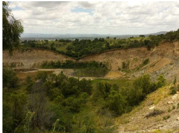
Figure 2.9 Unstable highwalls in north-western corner of site
