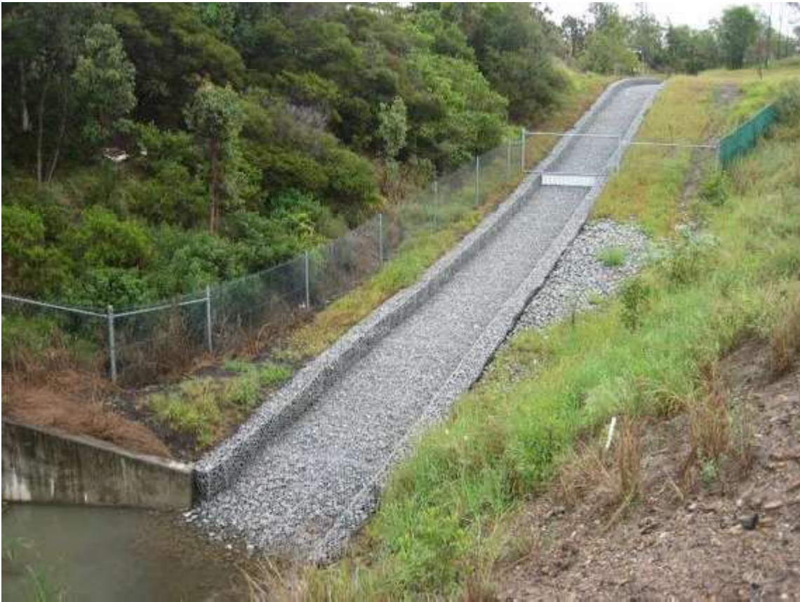
Example of gabion (Reno) mattress for discharging water safely down long steep slopes such as the internal channel
