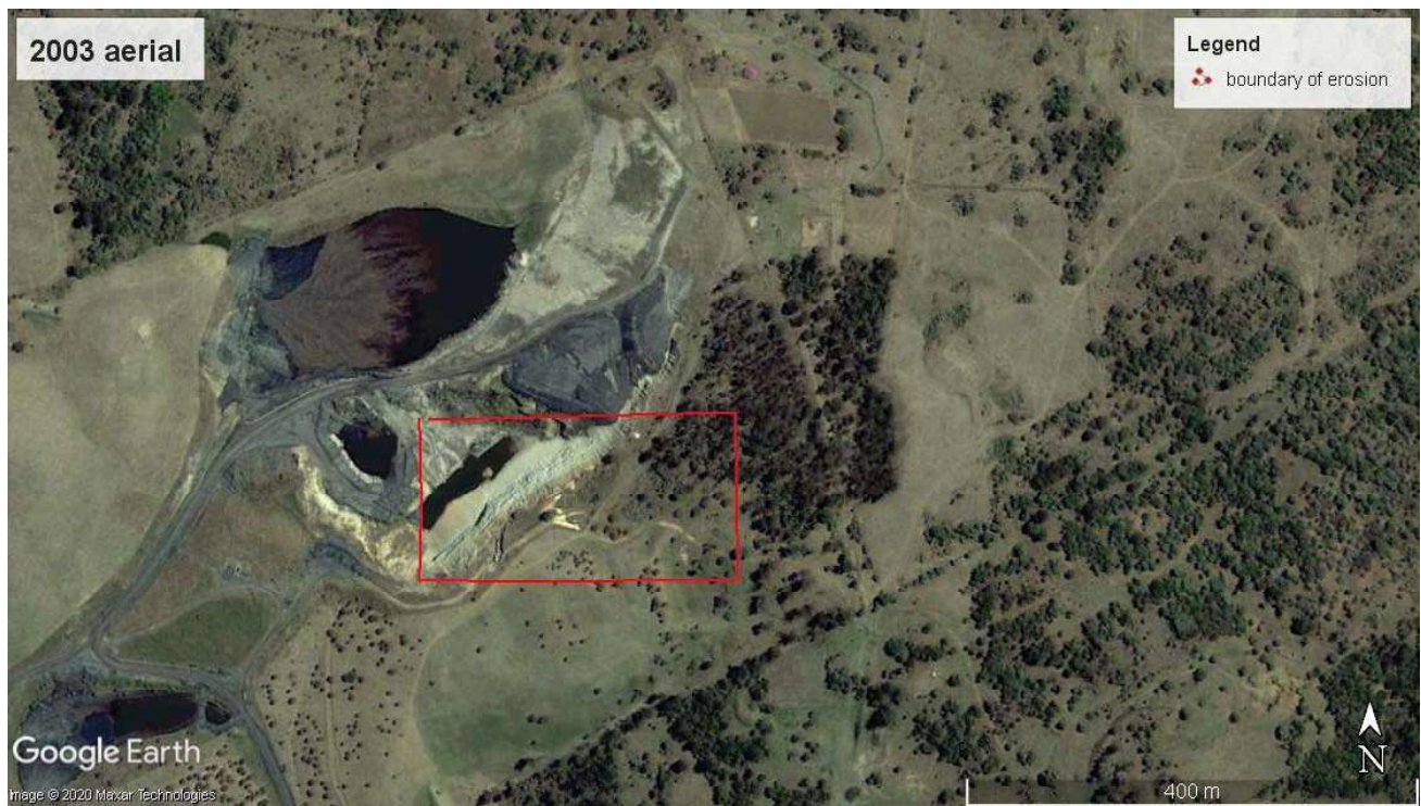
Figure 3.4 (a to d) Aerial sequence of changes to rehabilitation and erosion (2003-2020)
