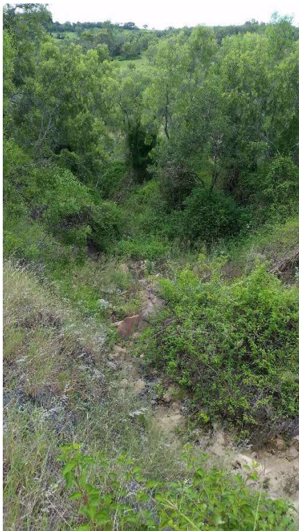
Oakleigh East - Washdown Dam Outlet
