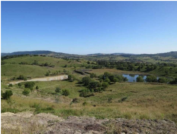
Figure 2.3 Reshaped landform looking north-east with tailings dam to the right and reshaped spoil to the left
