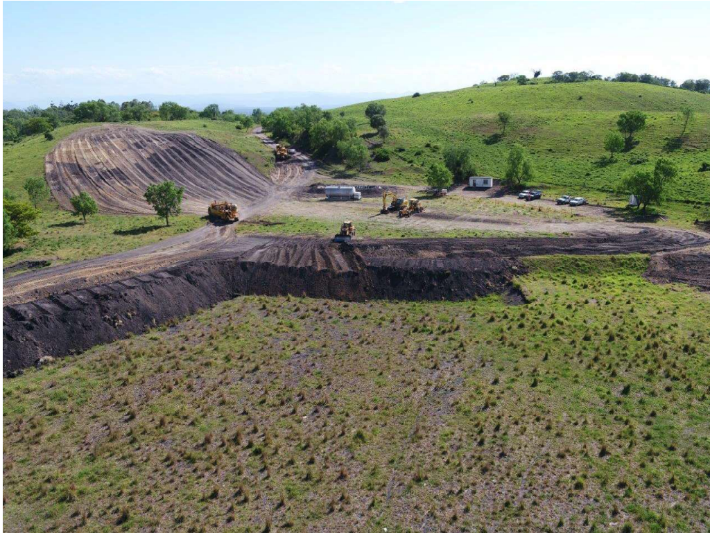
Oakleigh East – Tailings Dam Capping Operations
