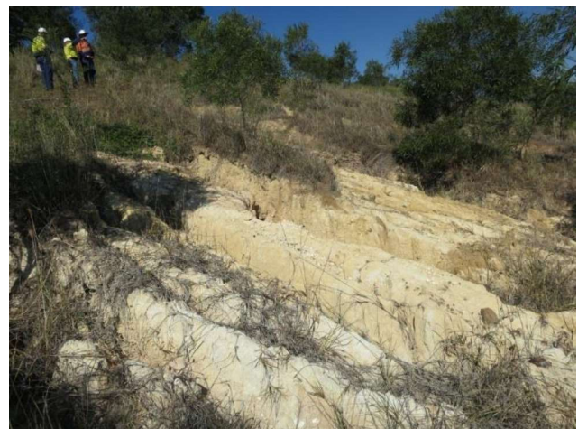
Figure 2.6 Gullying in sodic subsoil material exposed above highwall during reshaping
