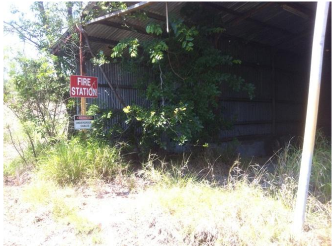
Photograph 78 – Fire station building from the underground era (15/11/11).
