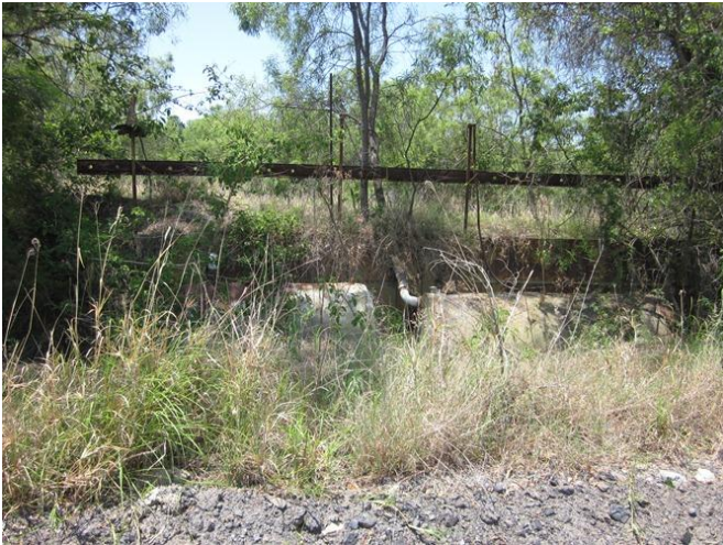
Photograph 41 – Above ground fuel tanks and refuelling infrastructure adjacent to the access road north of the Admin building (15/11/11).
