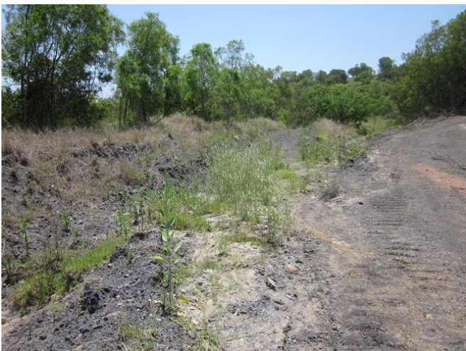
Photograph 57 – Road edges and drainage lines for surface water (15/11/11).
