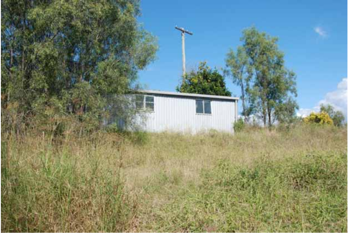
B8 – 7 Shed On The Top of Hill Behind Repair Room
