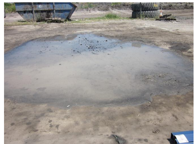
Photograph 12 – Wash down bay hardstand area with fine sediments observed on the surface (15/11/11).
