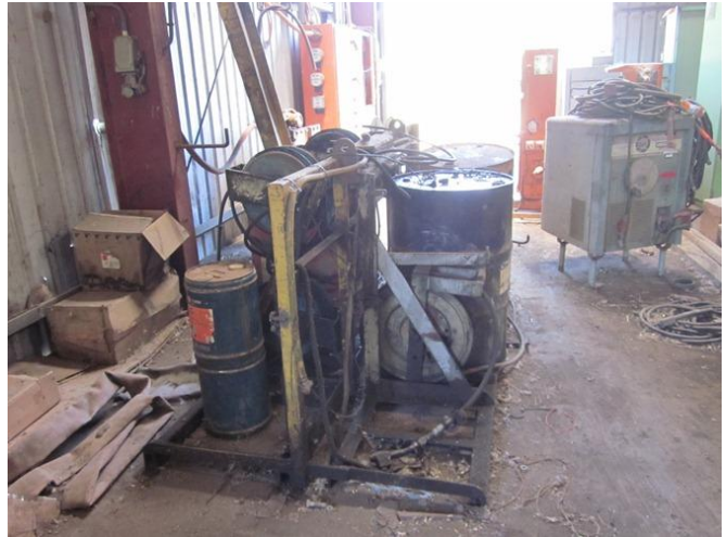
Photograph 66 – Equipment and fuel storage in the Operations workshop (15/11/11).
