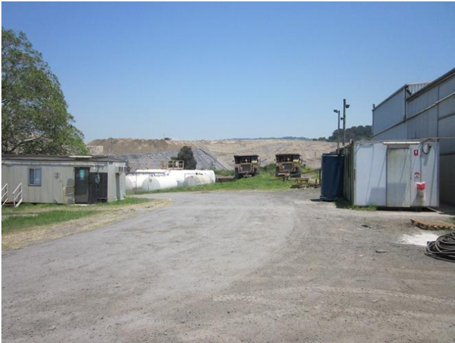
Photograph 29 – West Pit infrastructure: workshop ( right), refuelling area(at the back in the middle) and office buildings (left) (15/11/11).
