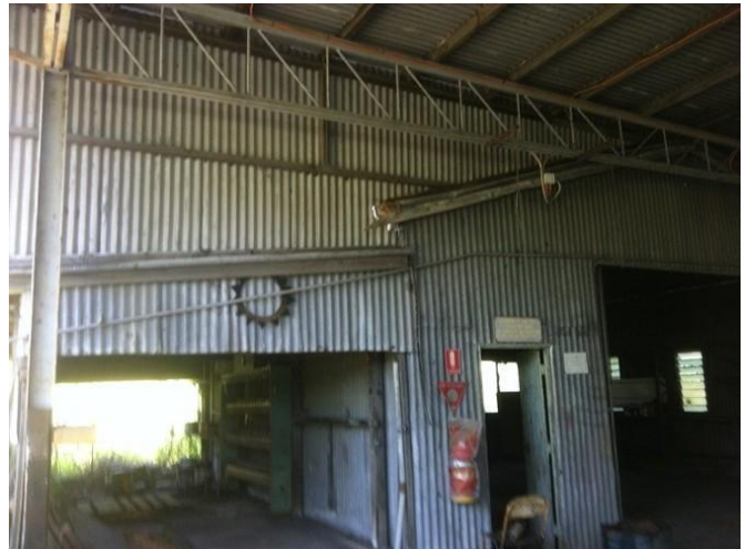
Photograph 84 – Workshop for underground area constructed of corrugated sheeting (15/11/11).
