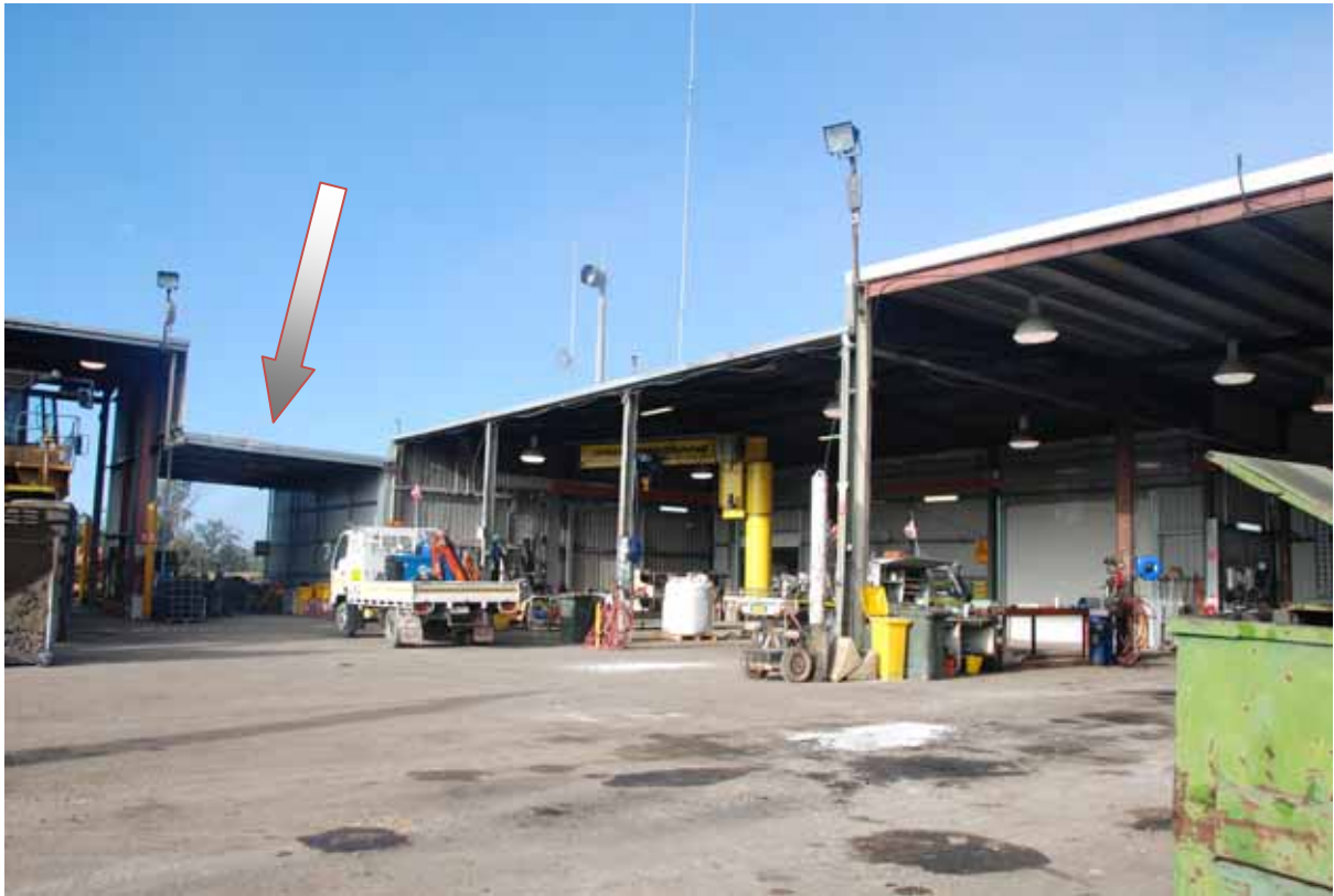
A2 – LV Work shed L-Form
