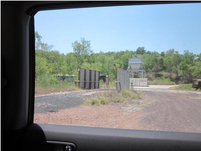
Photograph 31 – Eastern side of the site, view of disused wheel wash and coal loading hopper (15/11/11).
