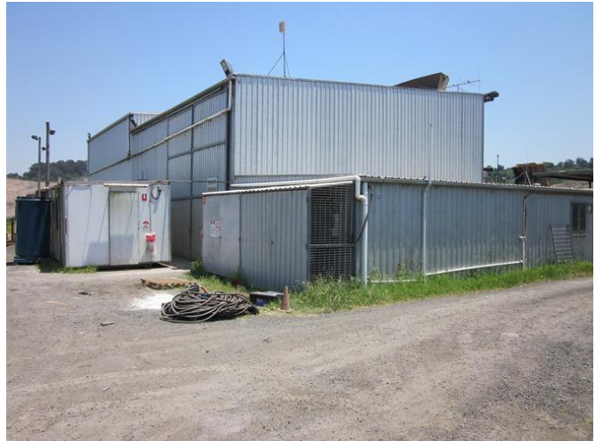
Photograph 30 – View of the shed structures comprising the workshop building (15/11/11).
