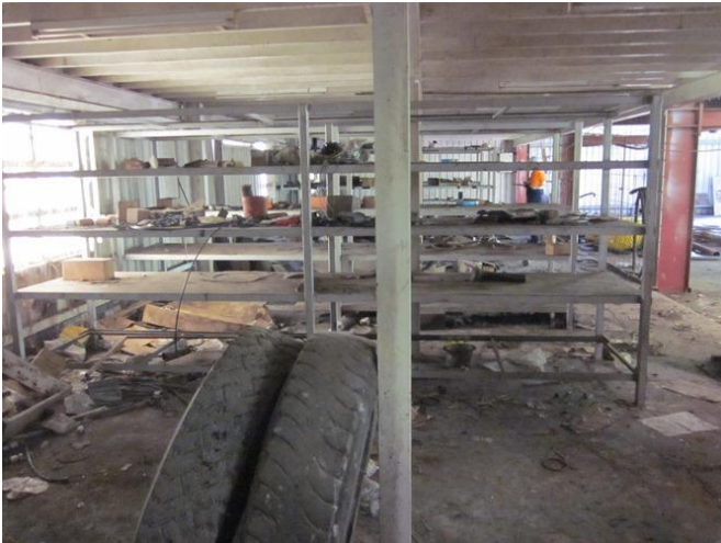
Photograph 71 – Storage area for spare parts located in north west portion of Operations workshop (15/11/11).
