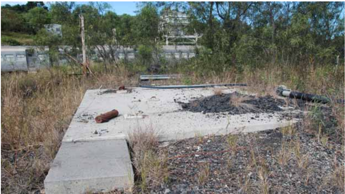
B5 – Concrete Block NO.1
