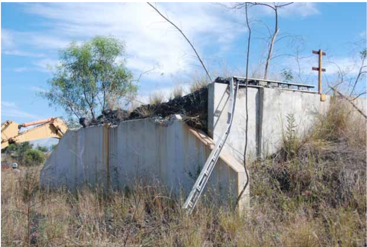
B5- Concrete Wall
