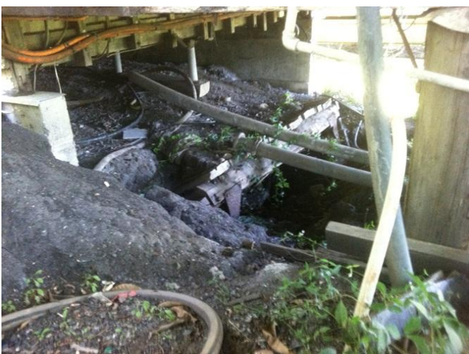
Photograph 81 – Old underground tunnel entrance (15/11/11).
