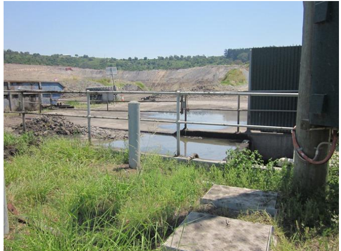
Photograph 10 – Wash down bay for with oil water separator and sediment trap (15/11/11).
