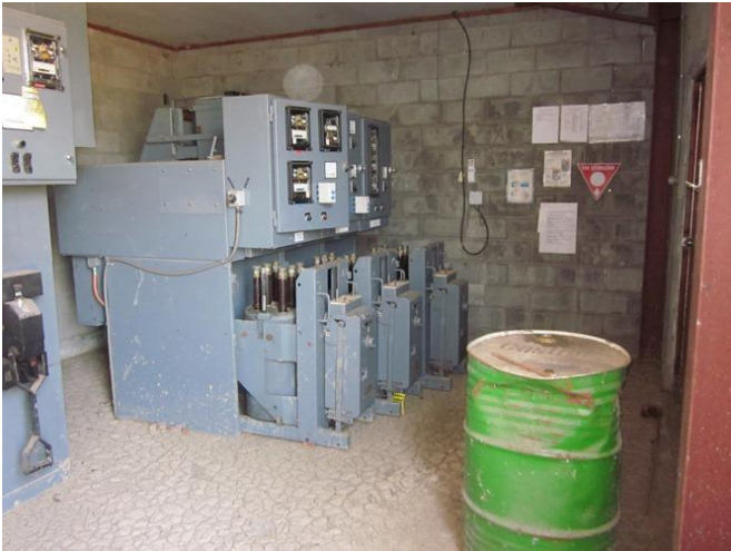
Photograph 47 – Inside the old electrical substation building (15/11/11).
