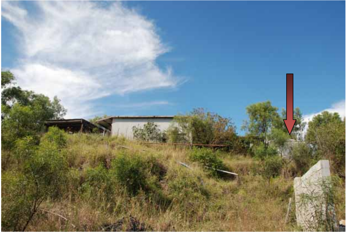
B8-5 Shed behind Repair Room
