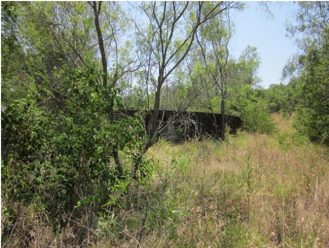
Photograph 53 – Old concrete water tank located to the north of old open cut buildings (15/11/11).
