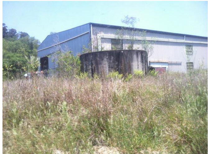
Photograph 74 – View from eastern side of the Operations workshop with guttering and concrete water tank collecting rainwater (15/11/11).
