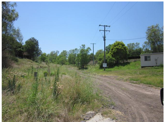
Photograph 40 – Site access road leading north from the Admin building to the north of the site.
