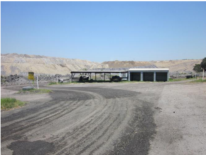
Photograph 3 – View west to the West Pit mining operations adjacent to the office and workshop buildings area (15/11/11).
