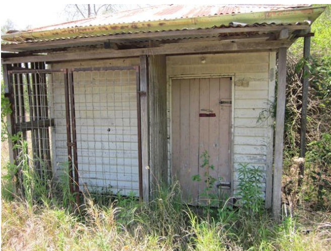
Photograph 51 – Old house, part of the old open cut buildings (15/11/11).
