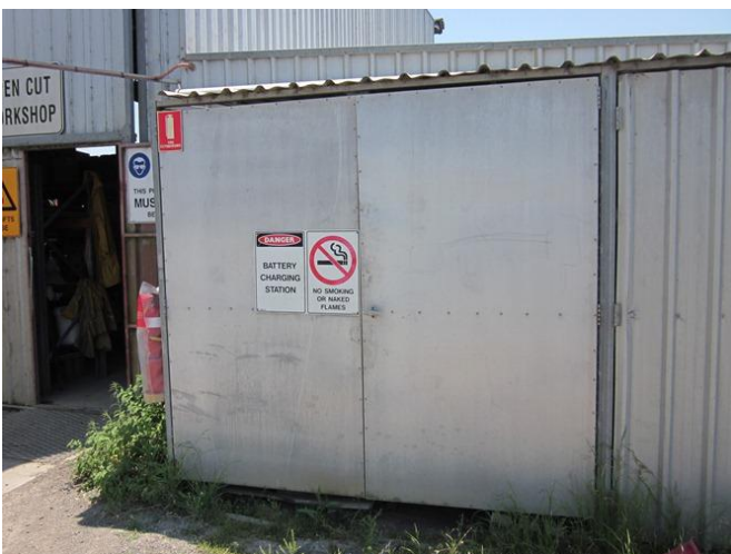
Photograph 27 – Battery charging area located to the south of the workshop building (15/11/11).
