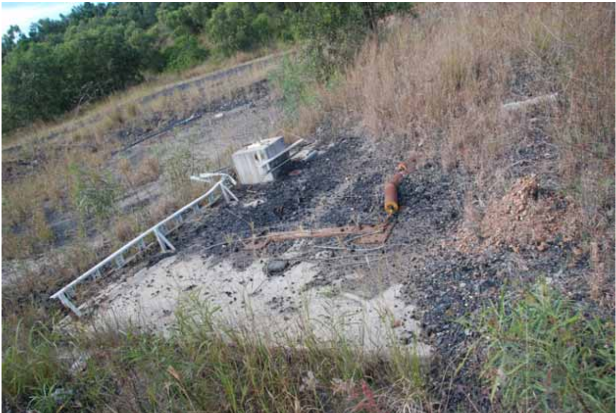
B5 – Concrete Block NO.3
