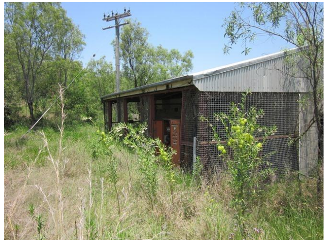
Photograph 50 – Old garage / workshop area (15/11/11).
