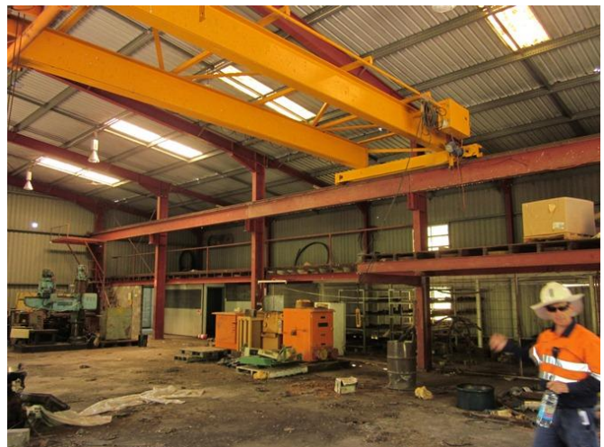
Photograph 64 – Operations workshop view from north to south (15/11/11).
