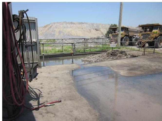
Photograph 11 – Wash down bay area with sediment collection sump (15/11/11).
