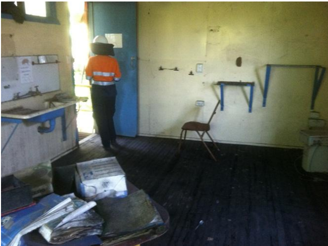
Photograph 83 – Office from underground operations located vertically above the tunnel entrance shaft (15/11/11).
