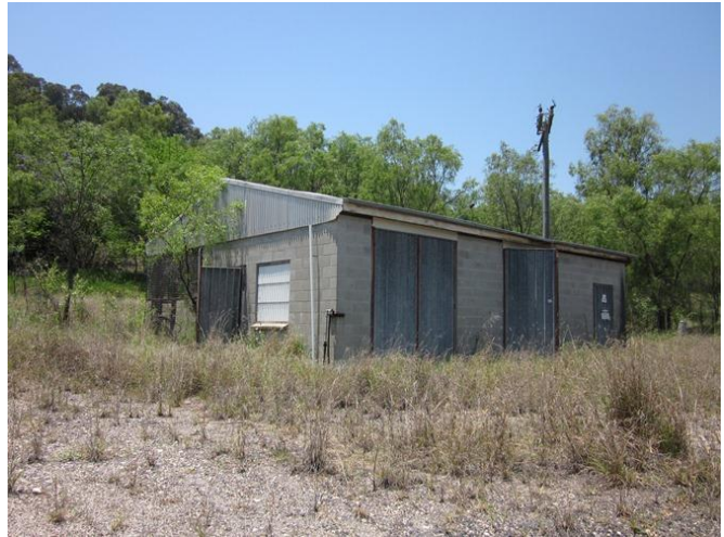
Photograph 42 – Electrical substation building and decommissioned power lines located east of the North Pit (15/11/11).
