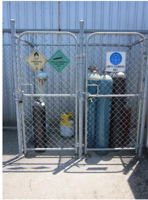
Photograph 20 – Designated gas cylinder storage area on the southern side of the workshop building (15/11/11).
