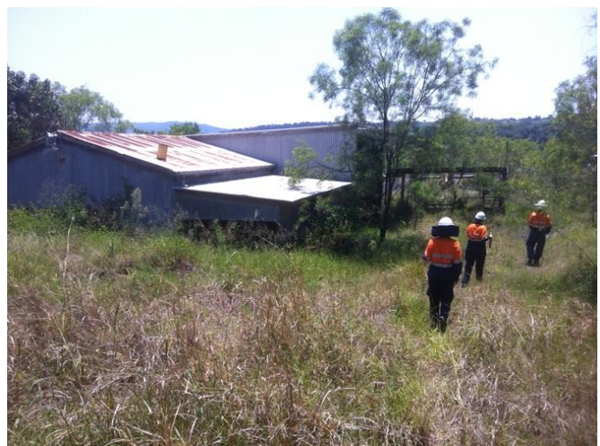
Photograph 76 – Collection of buildings comprising the surface buildings from the underground mining operations (15/11/11).
