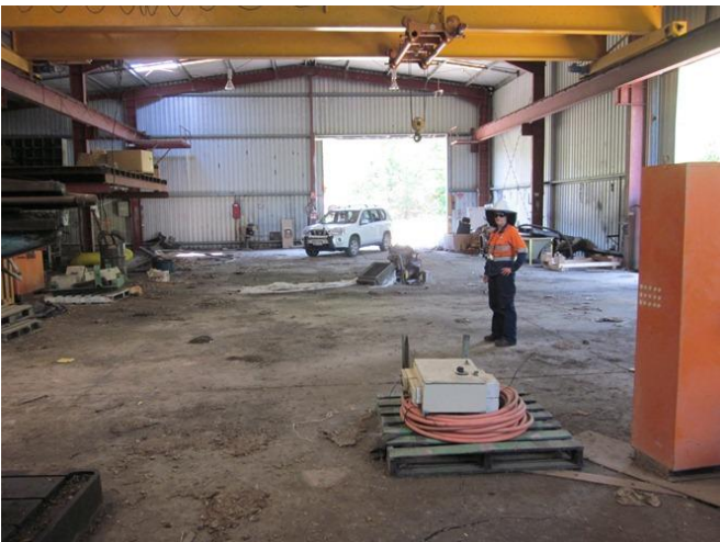
Photograph 69 – View of Operations workshop taken from south to north (15/11/11).
