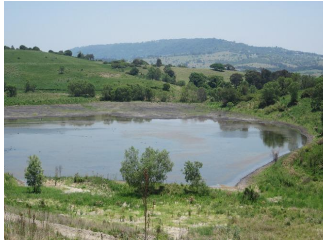
Photograph 60 – Zoomed in shot of the tailings dam (15/11/11).
