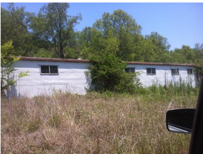
Photograph 75 - Old building located south west of the Operations workshop (15/11/11).
