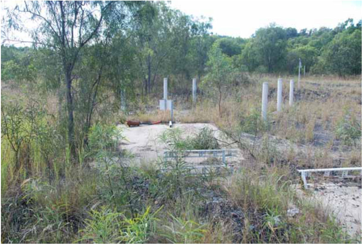
B5 – Concrete Block NO.2
