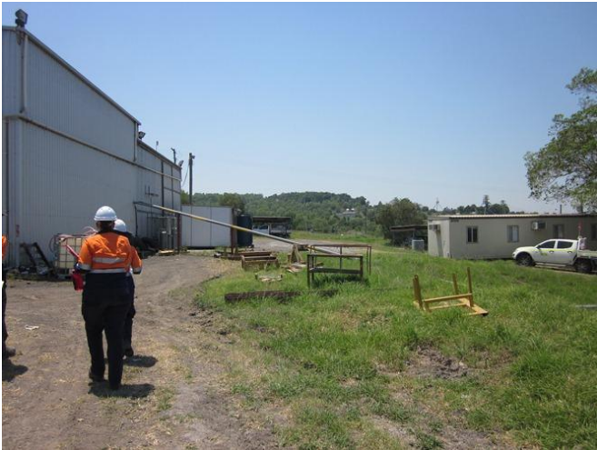
Photograph 15 – View to the east showing office buildings on the right and workshop building on the left of image (15/11/11).
