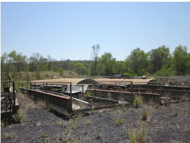
Photograph 33 – Storage of disused metal structures (15/11/11).
