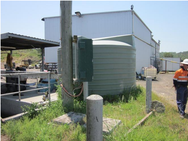
Photograph 13 – View of wash bay water tank, and workshop building in the background (14/12/11).
