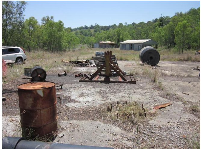
Photograph 44 – View north of the old open cut buildings showing the electrical substation, house, and garage / workshop area (15/11/11)
