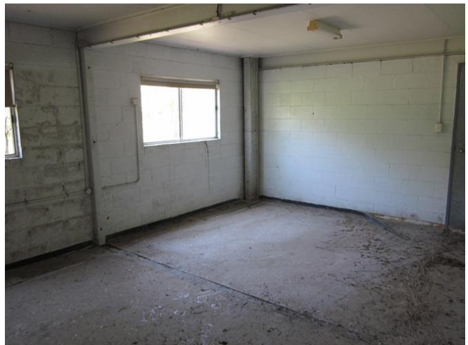
Photograph 70 – Typical construction of the series of rooms adjoining the Operations workshop (15/11/11).
