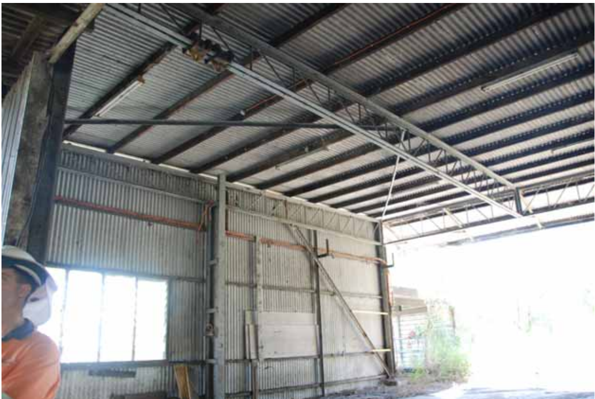
B8 - 1 Repair Room
