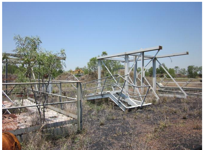
Photograph 34 – Storage of disused metal structures previously used for coal loading (15/11/11).
