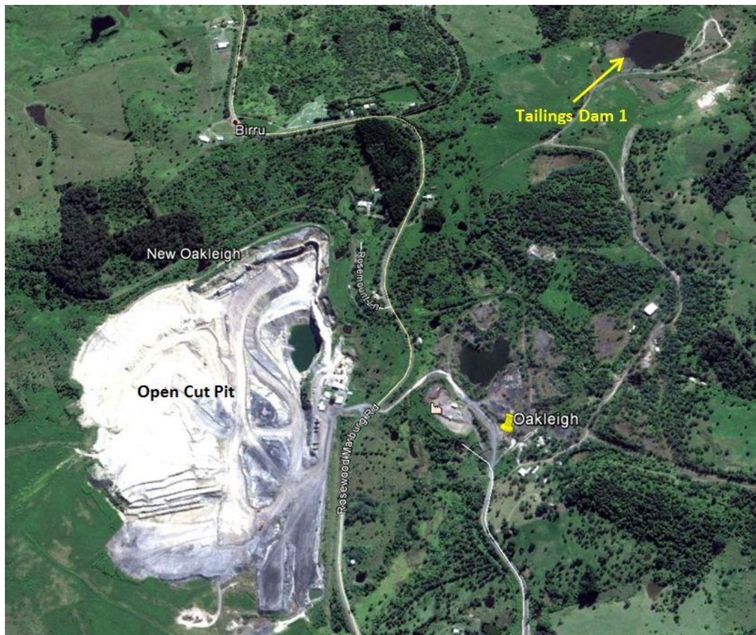
Plate 1 General Location of Tailings Dam 1
