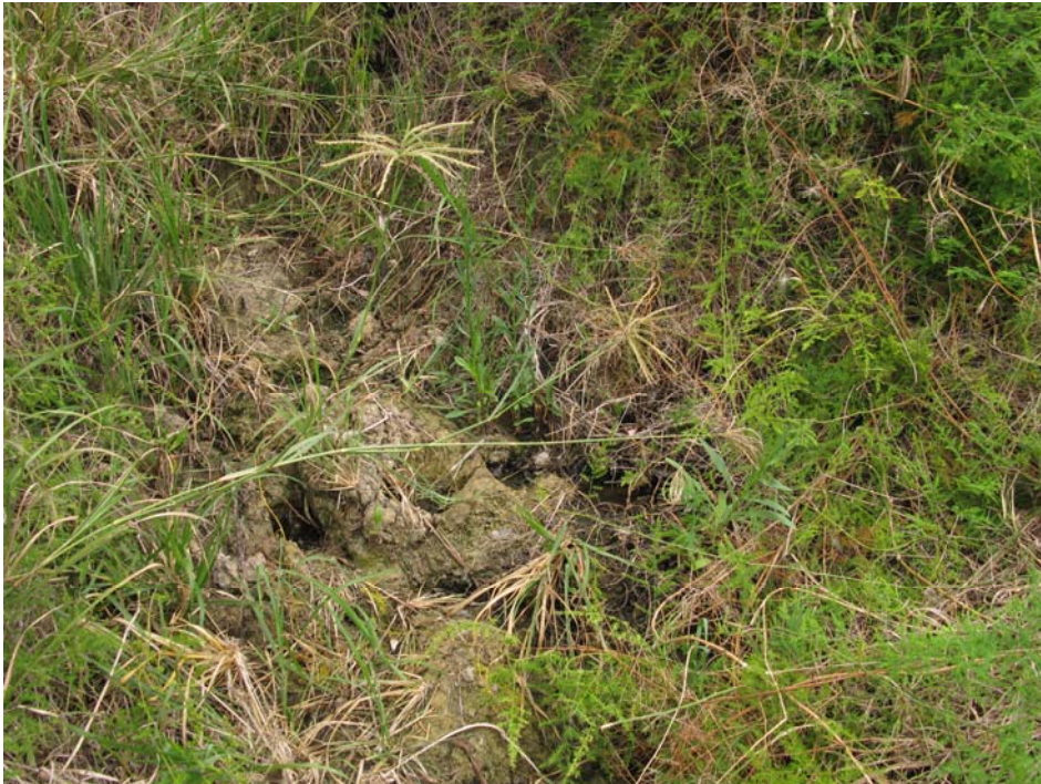
Figure 1: First seepage area in gully embankment in southern portion of Lot 2; note slight vegetation dieback and white desiccation crystals
