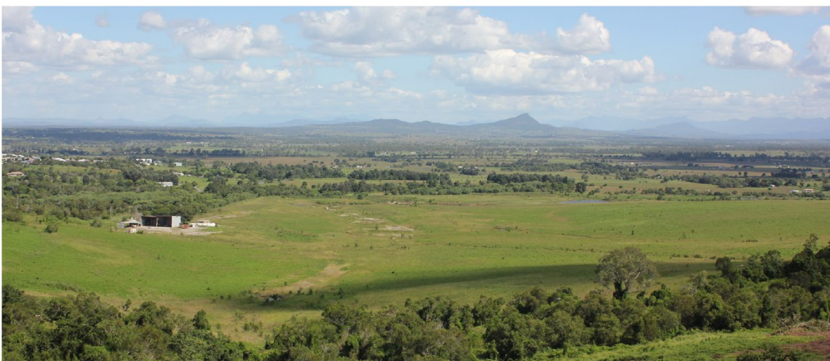
Figure 15: Oakleigh West: Post-rehabilitation—established grazing PMLU (2017; note retained infrastructure)
