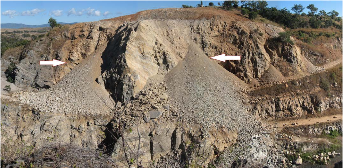
Figure 18. In 2014, a protrusion of limestone and sandstone on the west wall was excavated and the wall benched to reduce risk applicable to vehicles traversing along the haulroad during proposed mining. Some of the loose material was used to form a short section of the haul road and to cover the lower bench.
