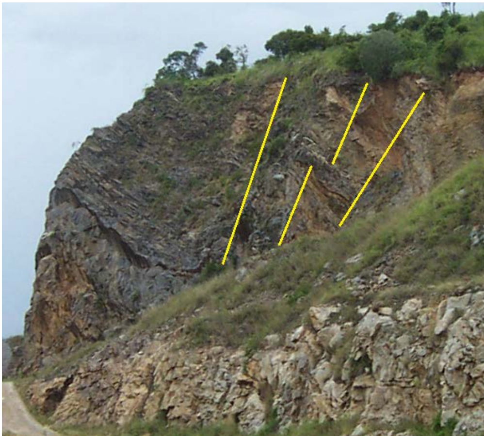
Figure 4. Examples of north-south striking faults in the west wall associated with fault F1 (refer Figure 3).
