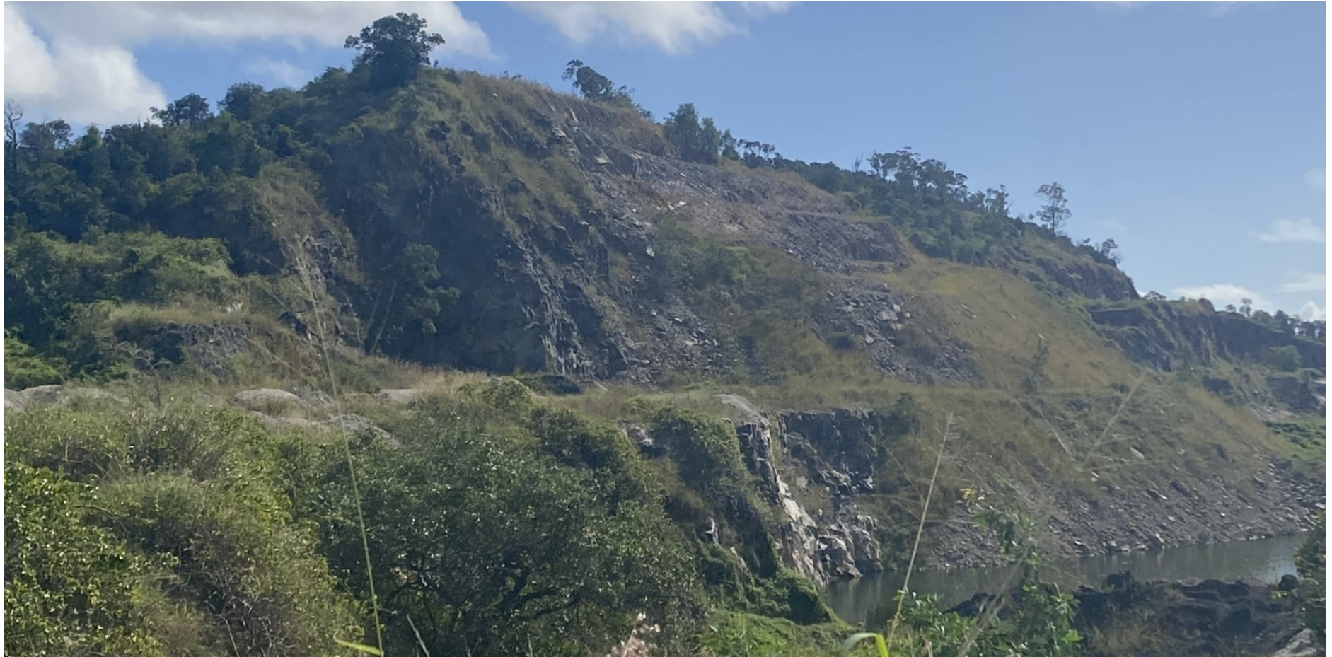
Figure 24. West wall looking north. The density of vegetation on the berms is moderate to high. It is sparse to moderate on the batters.
