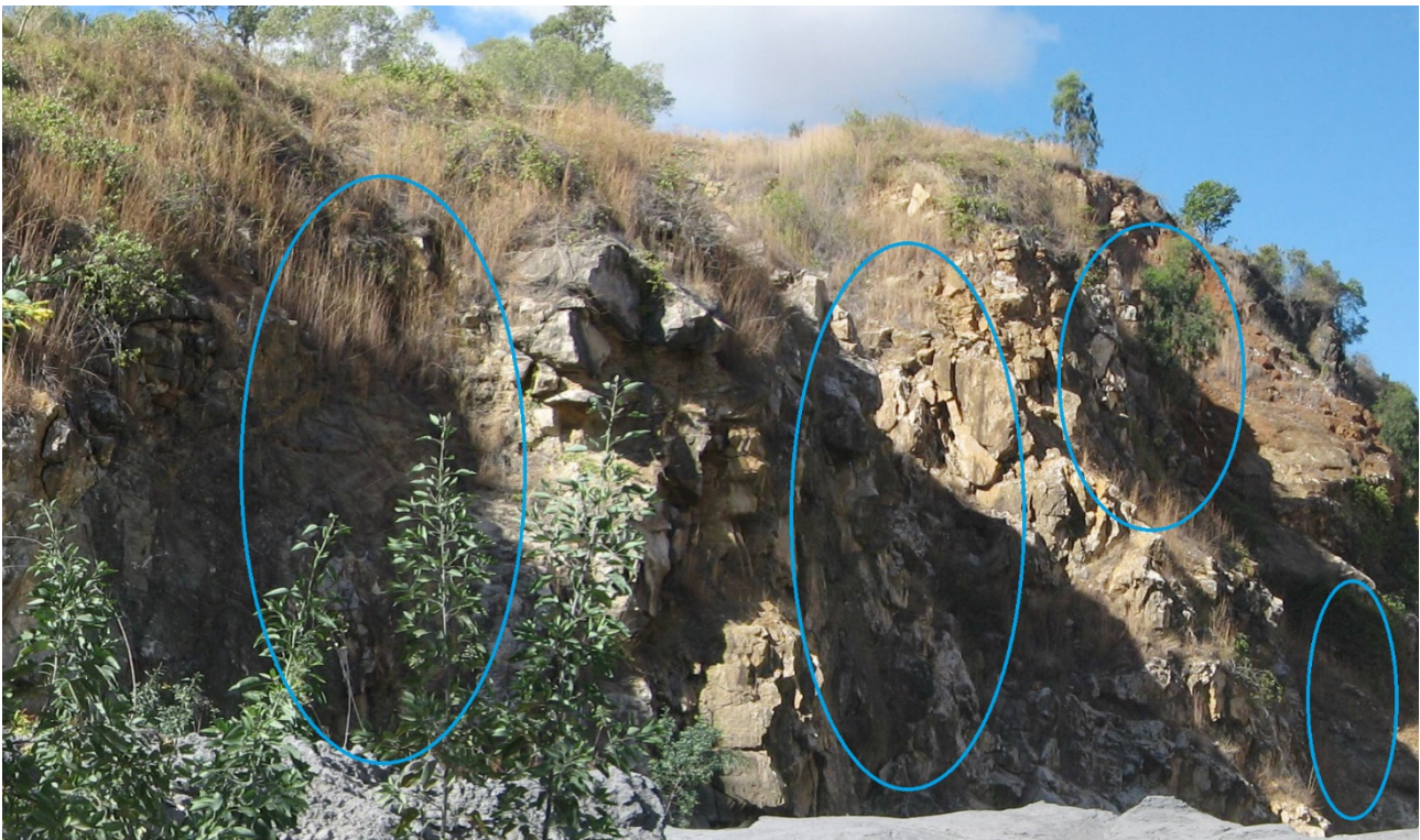
Figure 26. Highlighted midway along the east wall are examples of multi-bench (i.e., inter-ramp) and overall scale masses of rocks that have detached by toppling from, and sliding along, one or two discontinuities, predominantly from Sets 1, 4 and 5.
