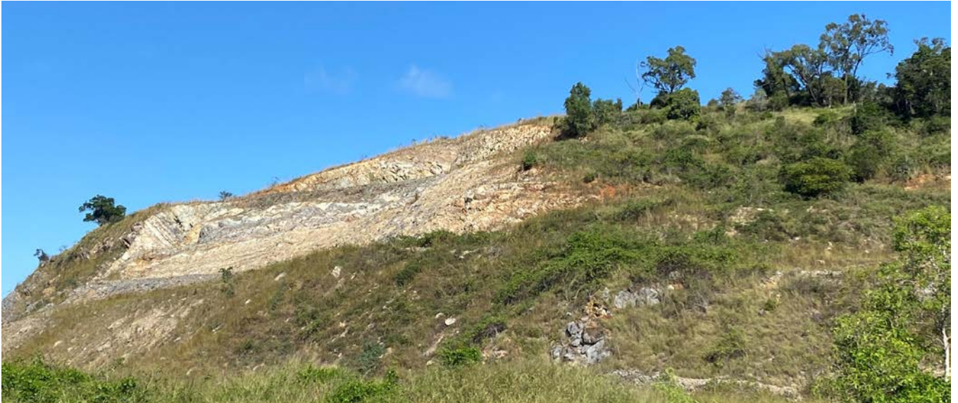
Figure 23. Vegetation is sparse below the crest of the section of the west wall where earthworks were undertaken in 2014.
