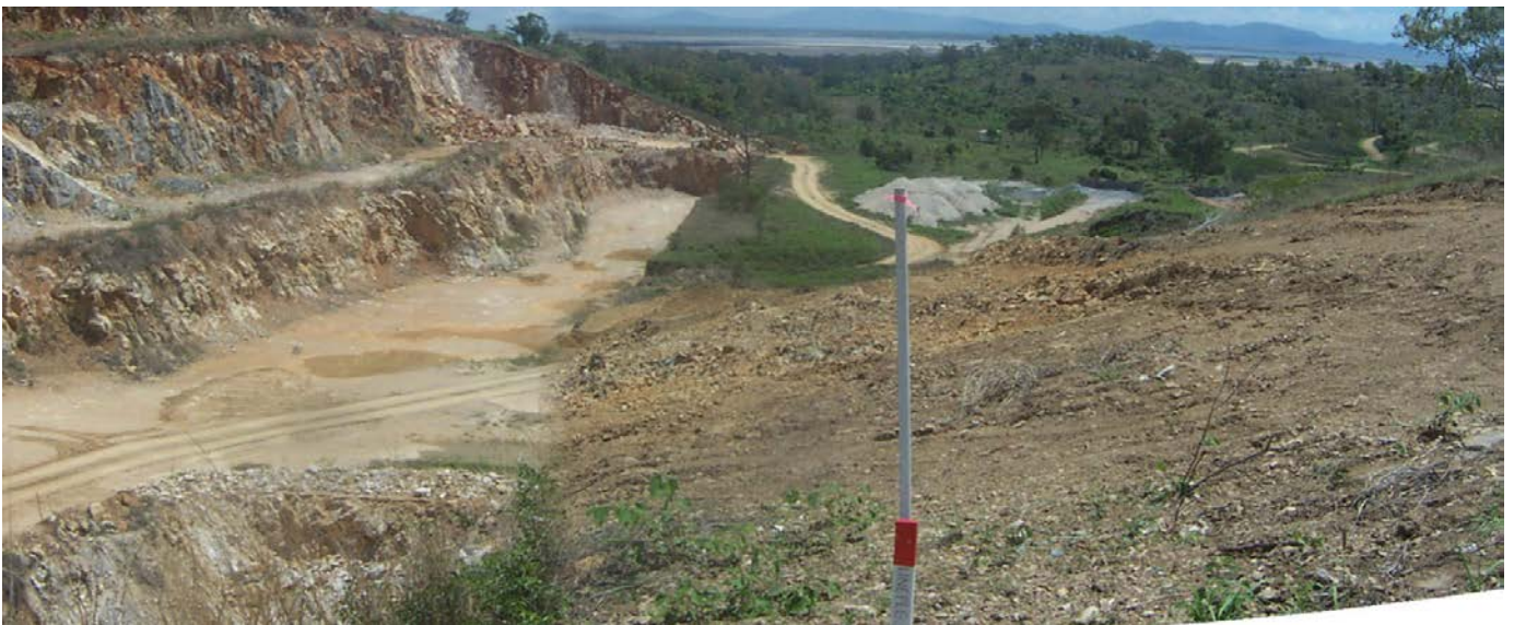
Figure 19. In 2014, the crest of the east wall was cut back to ensure the risk applicable during proposed mining on the pit floor would be acceptable.
