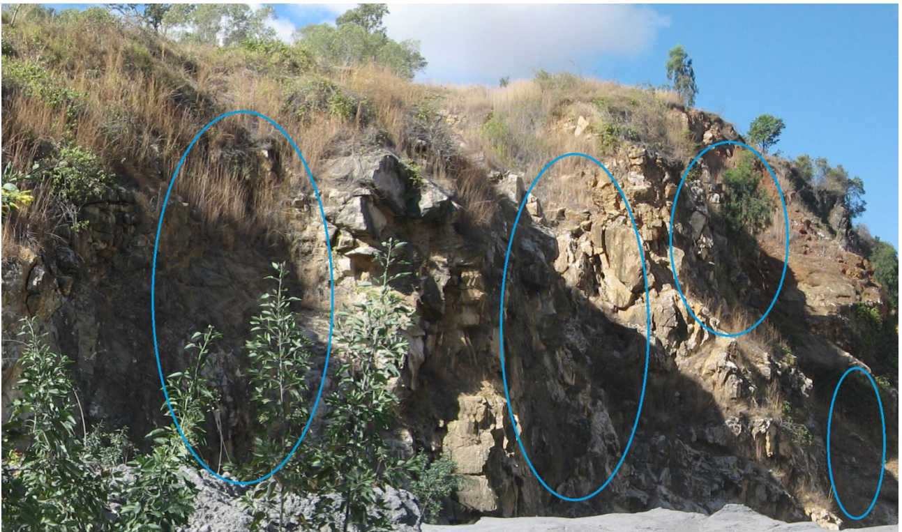
Figure 26. Highlighted midway along the east wall are examples of multi-bench (i.e., inter-ramp) and overall scale masses of rocks that have detached by toppling from, and sliding along, one or two discontinuities, predominantly from Sets 1, 4 and 5.
