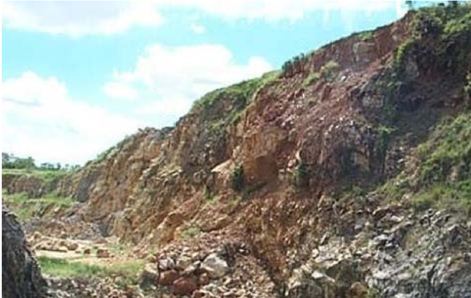
Figure 20. Rocks pushed over the crest of the east wall during the 2014 cutback triggered instabilities of individual rocks and masses of rocks on the wall that had marginal capacities. Doing so, and subsequent scaling, reduced the number of hazards.
