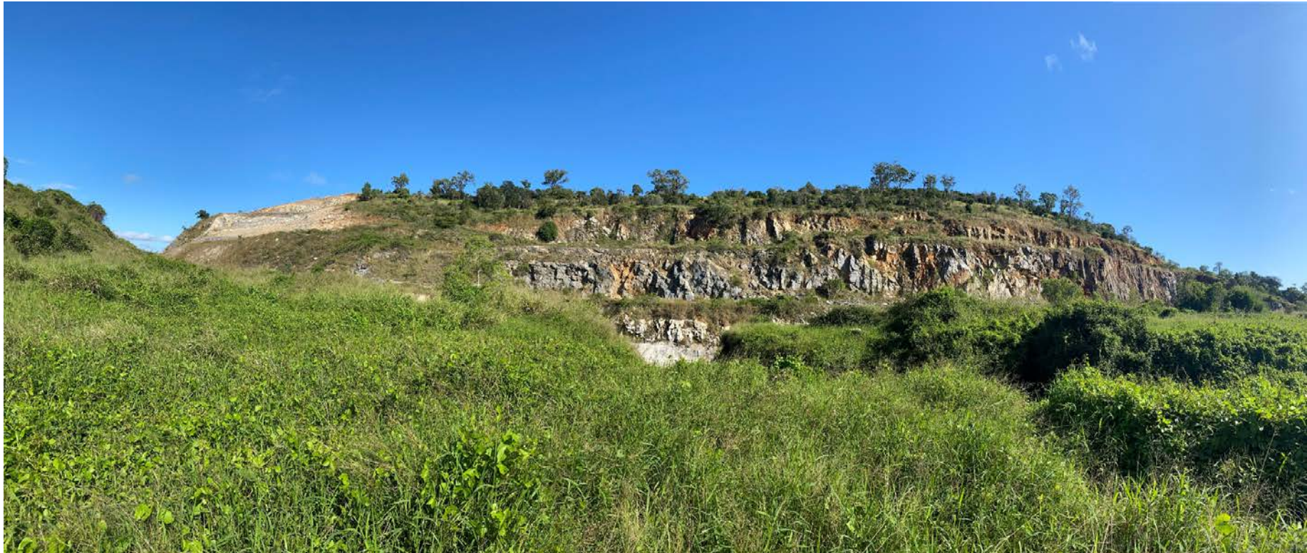
Figure 21. View from behind the crest of the east wall looking towards the west wall. The density of vegetation behind the crests of all walls is high. It is moderate to high on the berms.
