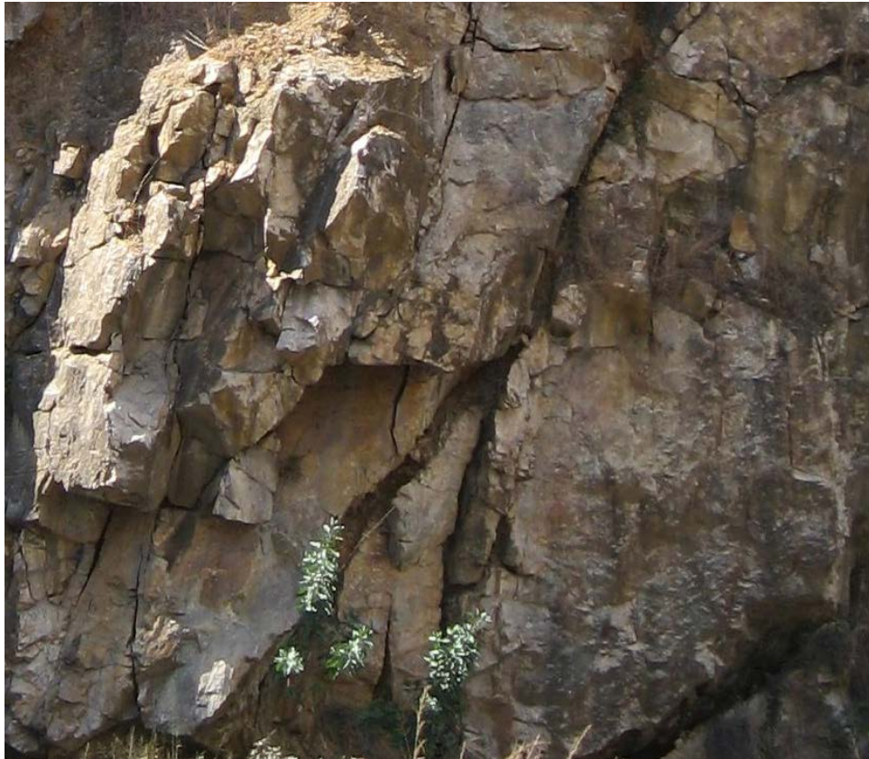
Figure 15. Most blocks of limestone are less than 50 cm in size, consistent with the results of rock size analyses in Section 2.6.5. The surfaces of the discontinuities in the direction of sliding (i.e. down) are slightly rough and undulating. These characteristics contribute positively to their shear strengths.
