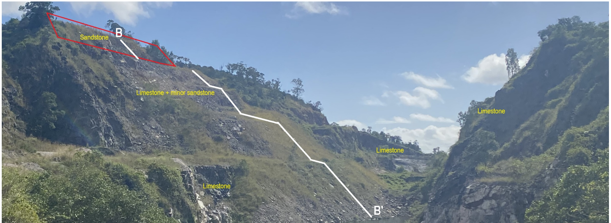
Figure 2. General rock types exposed in the pit walls. Vegetation density is high behind the crests and sparse to moderate on the walls and the pit floor. The stabilities of the east and west walls along cross-section B-B' is considered in Section 4.2.2.
