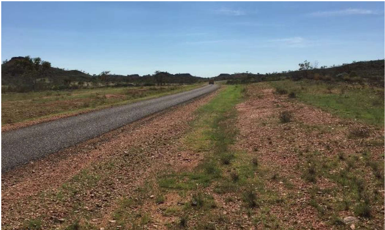
Figure 5-7 Diamantina Developmental Road looking east from the proposed site access
