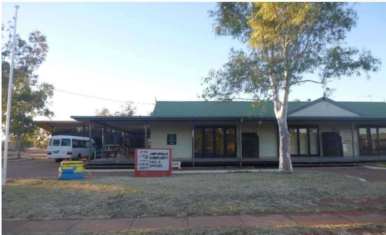
Plate 24: Jimberella Community Hall
