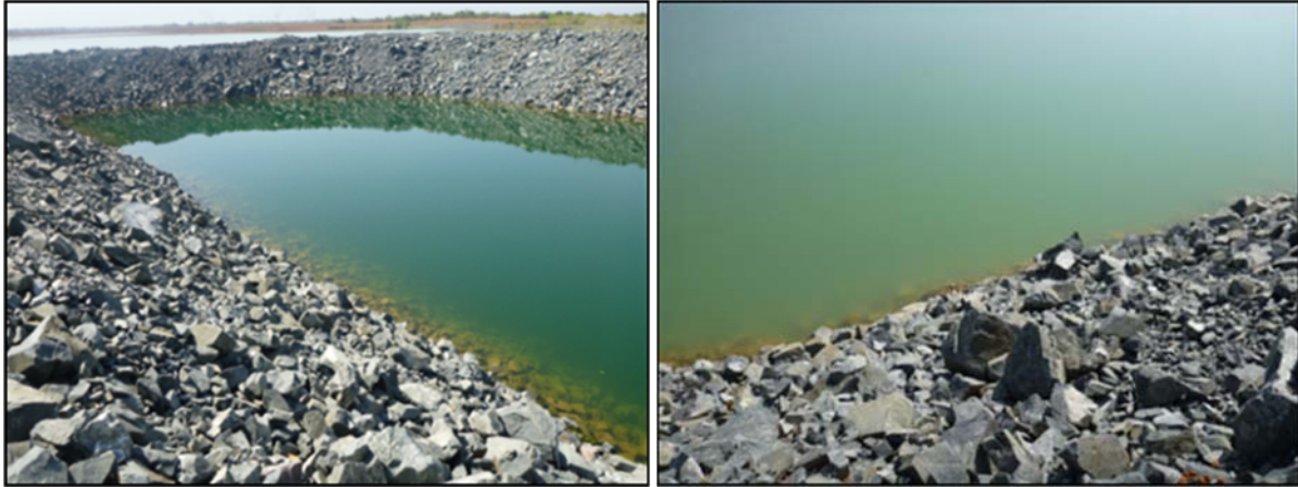
Figure 7-3 - Supernatant water inside the rock ring (left) and outside the rock ring (right)
