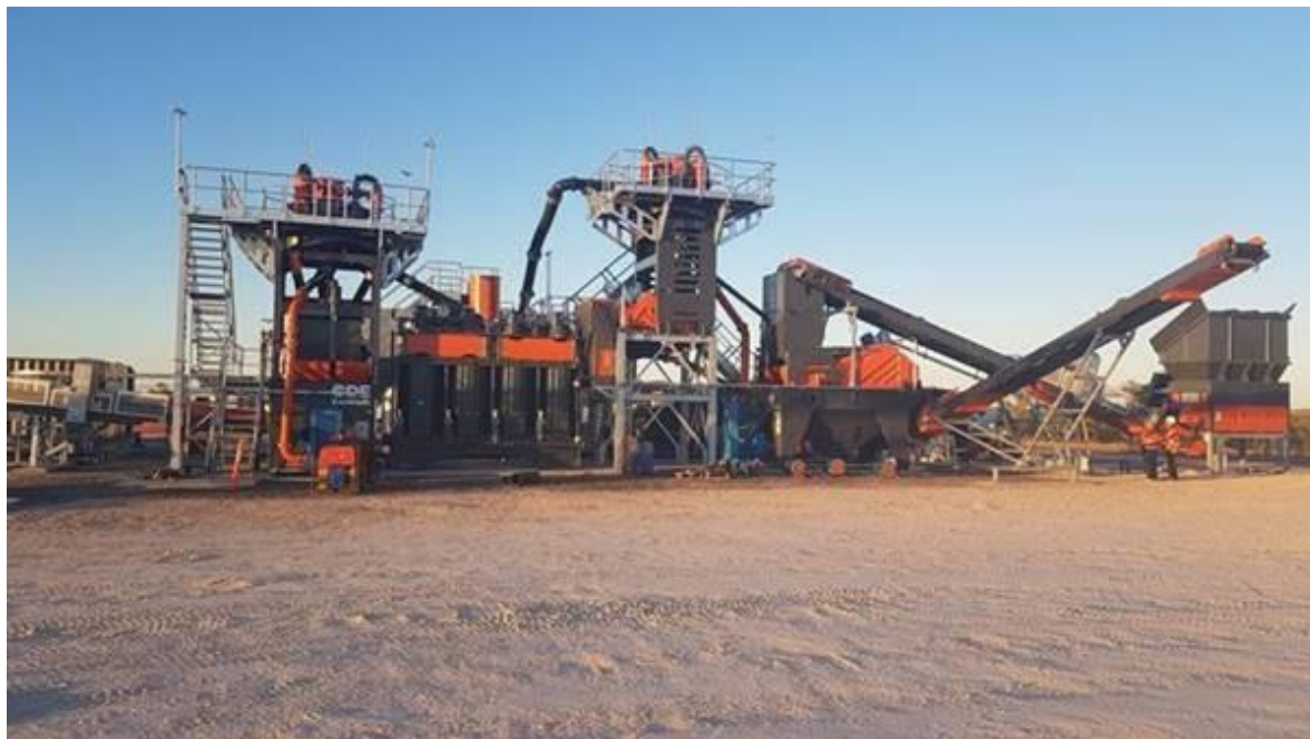
Figure 26: Processing plant area
