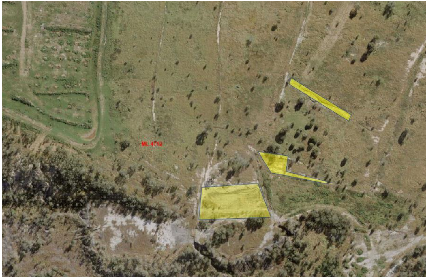
APPENDIX 2 - IMAGE 10: AREAS WITHIN LANES EASTERN EMPLACEMENT REQUIRING REHABILITATION
