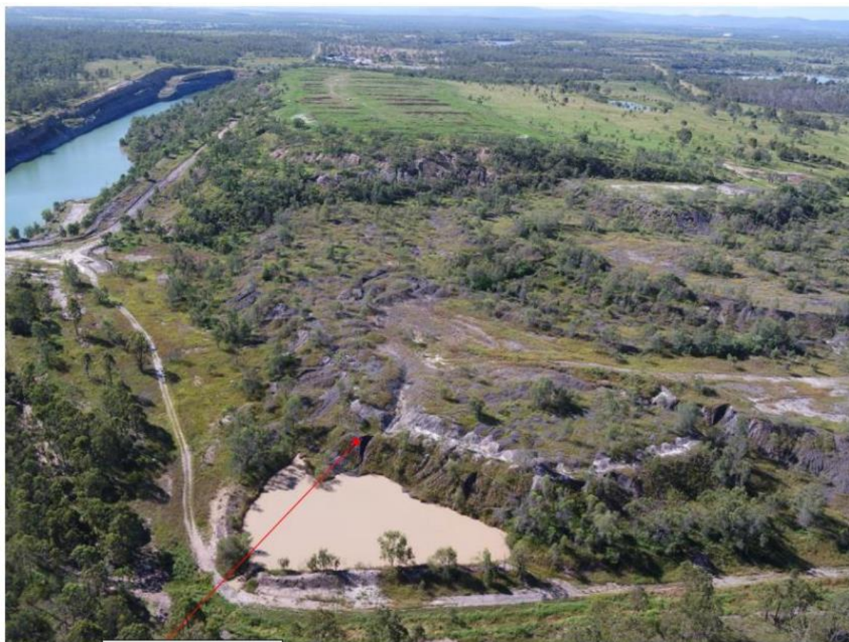
Drain to be stabilised
