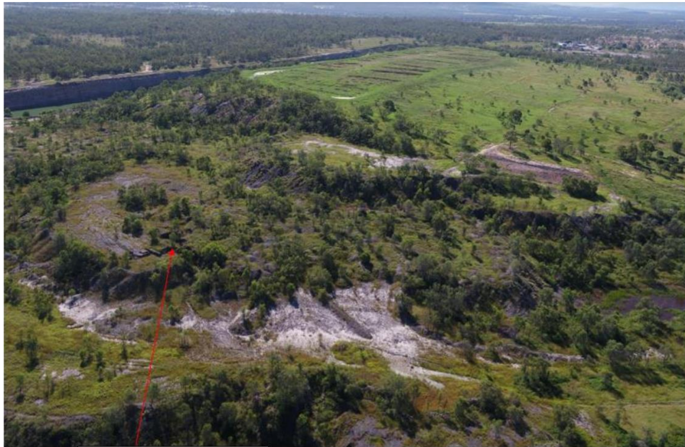
Deep Erosion Requiring Backfilling
