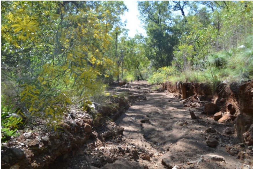
Figure 11: Bywash Dam 3 – November 2022
