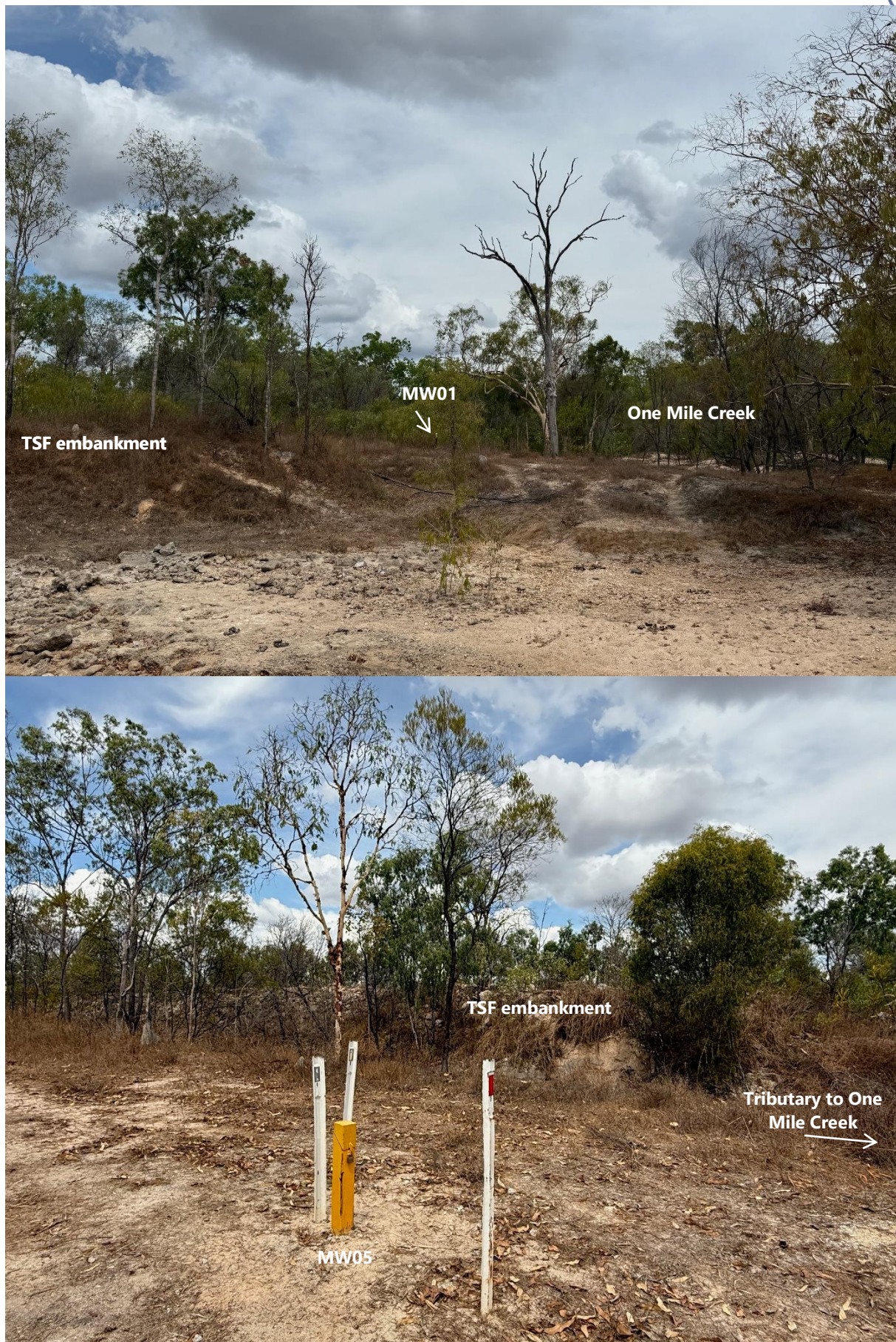
Figure 78 - View of MW01 and MW05 with other landforms
