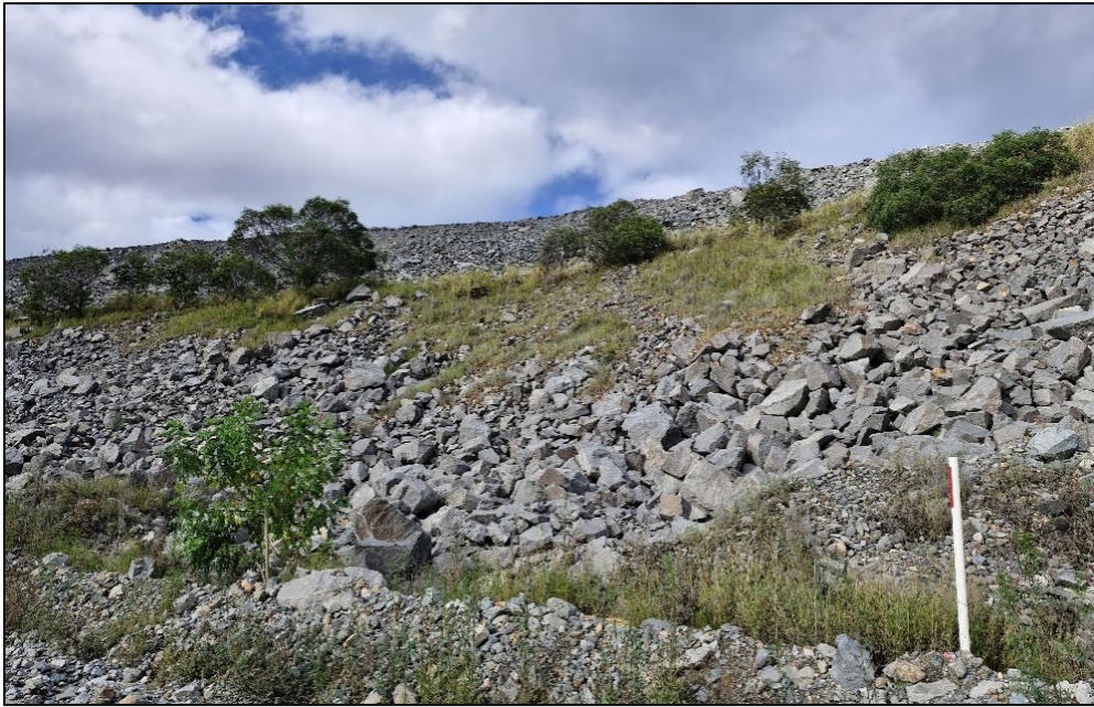
Figure 2.7: Coarse overburden material comprising the angle of repose NWRD batters adjacent to the open pit (Okane, 2024).
