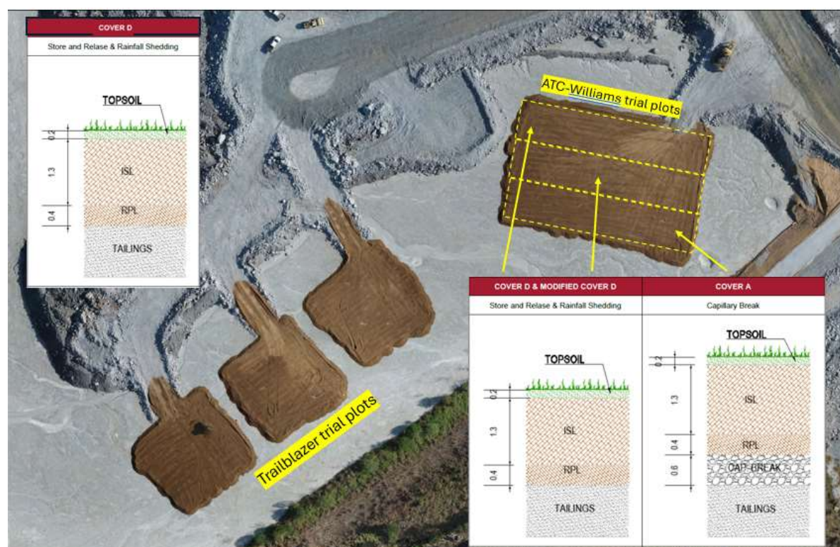
Figure 93 : ATC-Williams and Trailblazer cover trial plot locations on TSF (October 2024).
