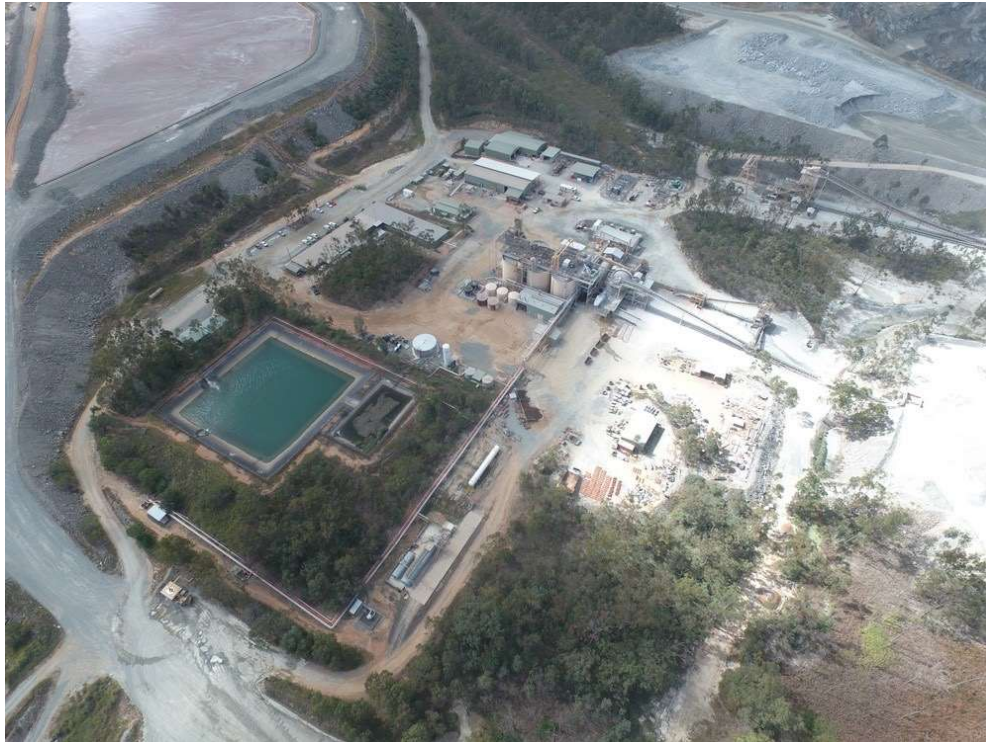
Figure 89: Main Infrastructure Area at MRO, as Viewed from the South.
