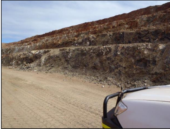
View of benching at excavation batter
