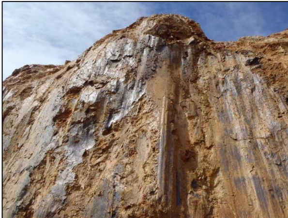
Weathered rock and clay exposed in batter
