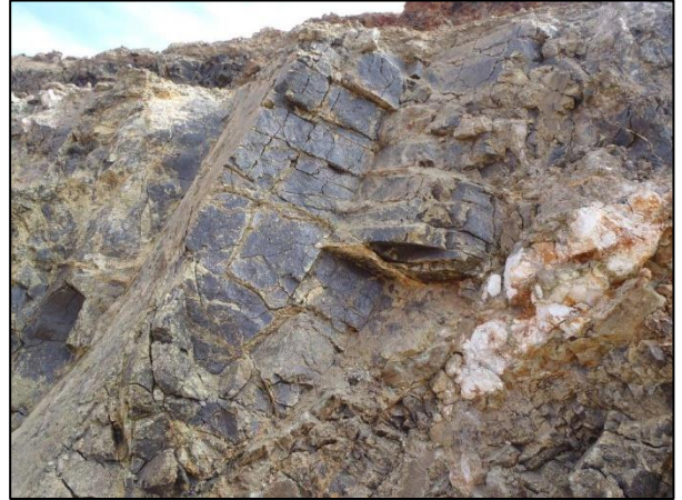
Serpentine rock exposed in batter face
