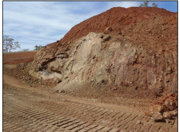
Serpentine rock exposed in batter face
