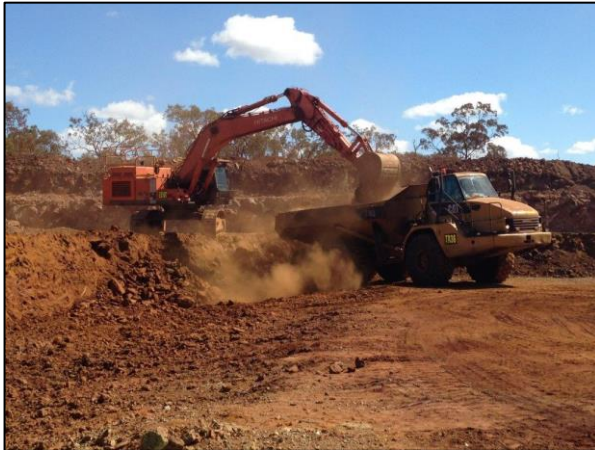
View of benching at excavation batter
