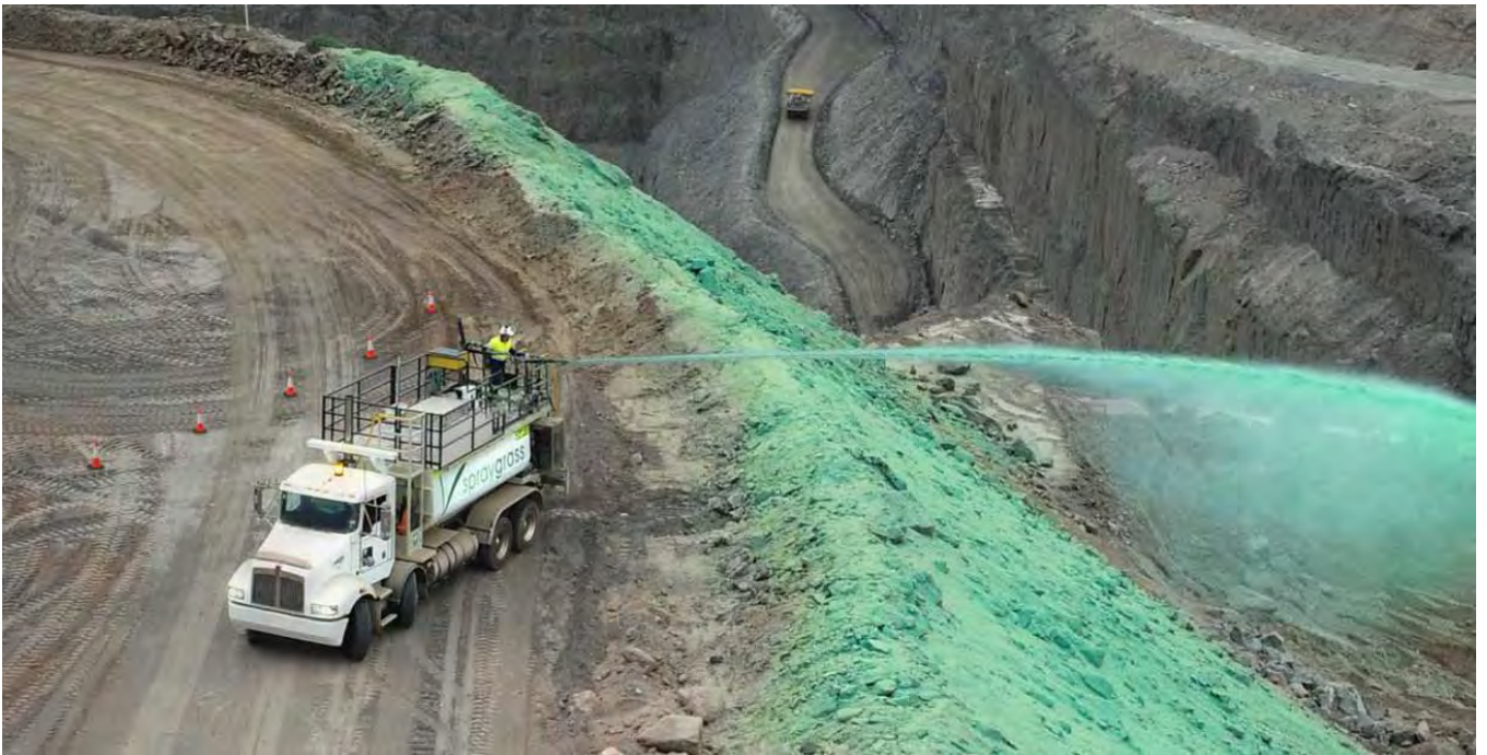
Figure 55. Hydroseeding, and desirably hydromulching, are recommended for the batter adjacent to the main ramp along the east wall of the Phoenix pit and for spraying topsoil on WRD 2.
