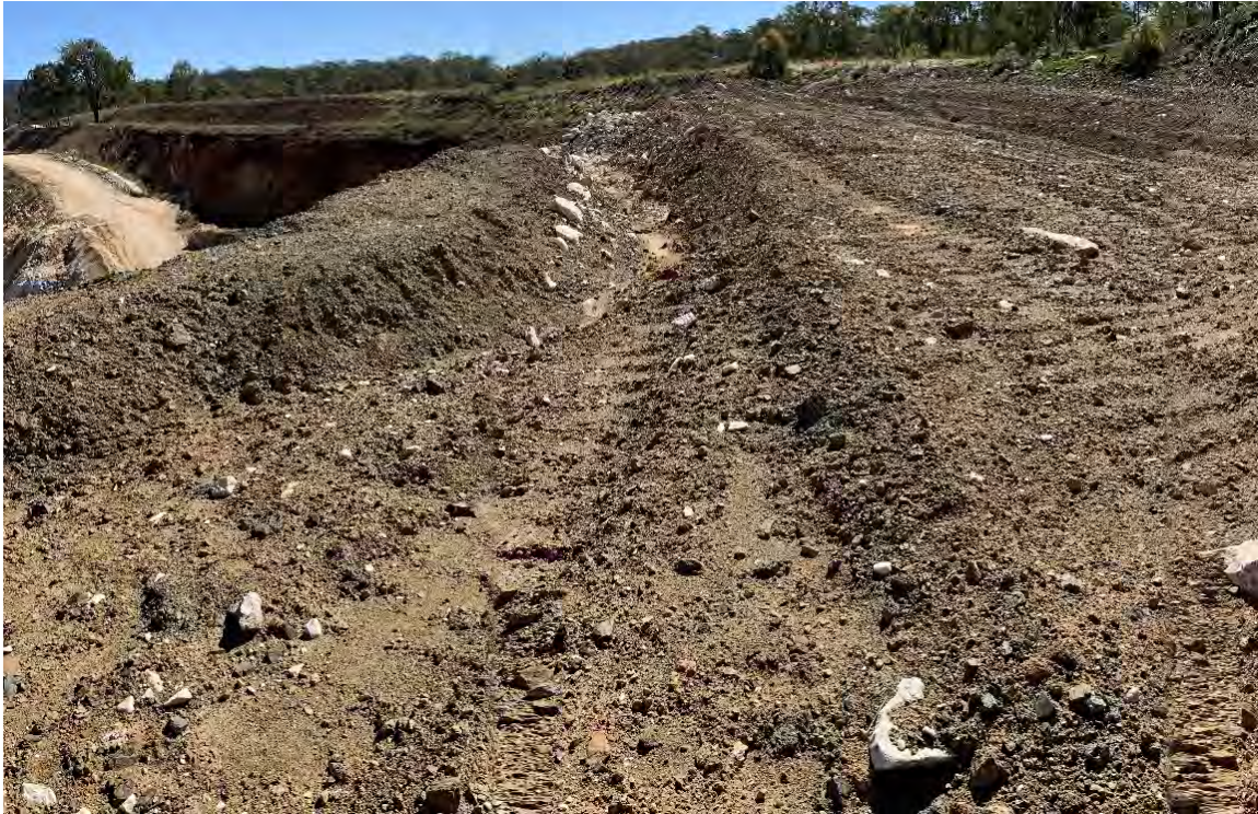
Figure 39. The haul-road along the east end of the Phoenix pit is to be graded to shed water to the east, removed by ripping and hydroseeded.
