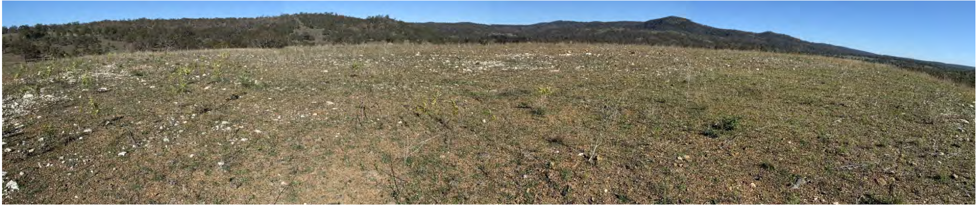
Figure 45. Upper surface of waste rock dump 1 (WRD 1) to the west of the East-West pit. The surface has been contoured and topsoil spread enabling a low to moderate density of grasses to establish.
