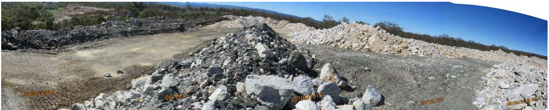
Figure 46. Upper surface of the southern section of waste rock dump 2 (WRD 2) to the southeast of Phoenix pit. The surface shaping, grading, crowning, topsoil and hydroseed.
