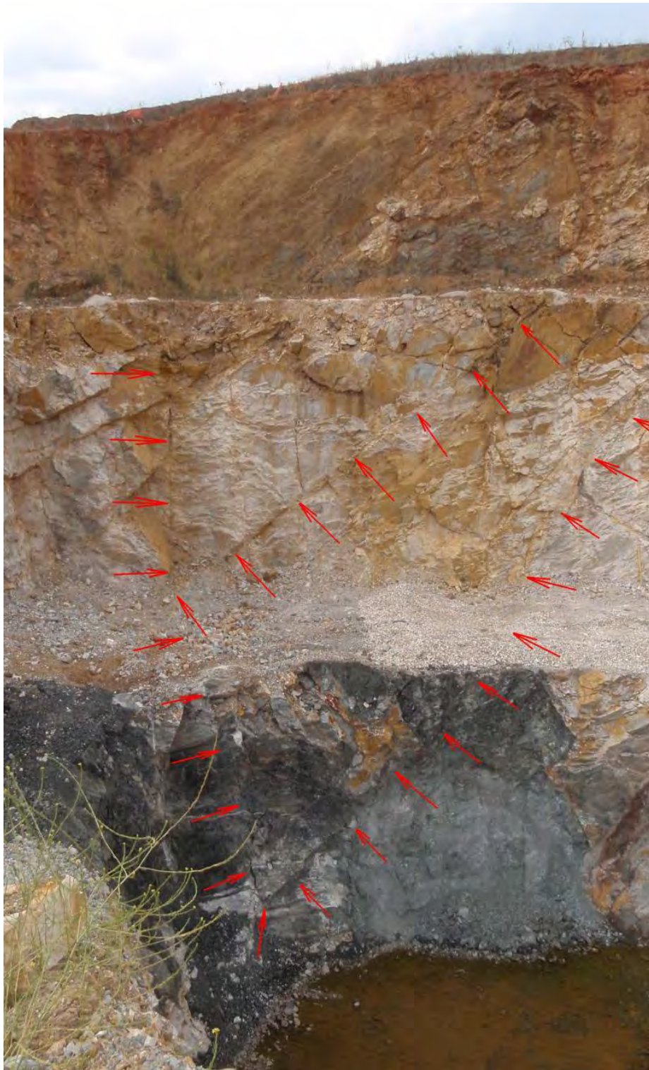
Figure 12. Examples of traces of large wedges formed by the intersections of faults and bedding.
