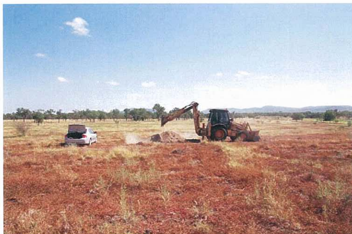
Figure 2-1: General view of SCP area from the low ridge in the south-east of the site at the proposed rail loop. Note generally flat floodplain area with stands of open woodland in the background.
