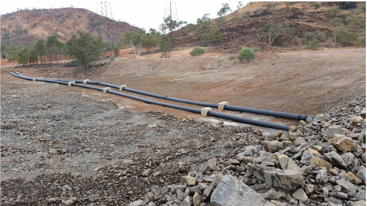
Photograph I-12: King Gully Dam, Downstream; BSOC Seepage Diversion to KSOC
