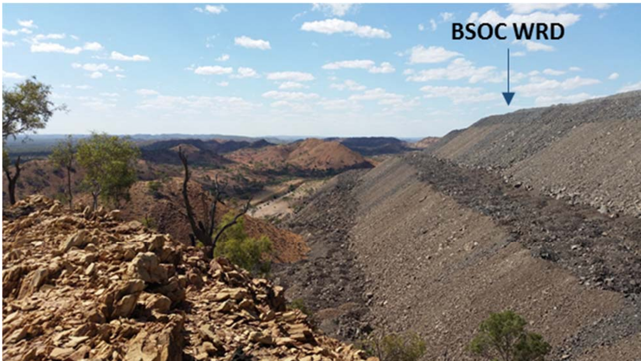
Figure 4-2: BSOC WRD, facing north (August, 2015)
