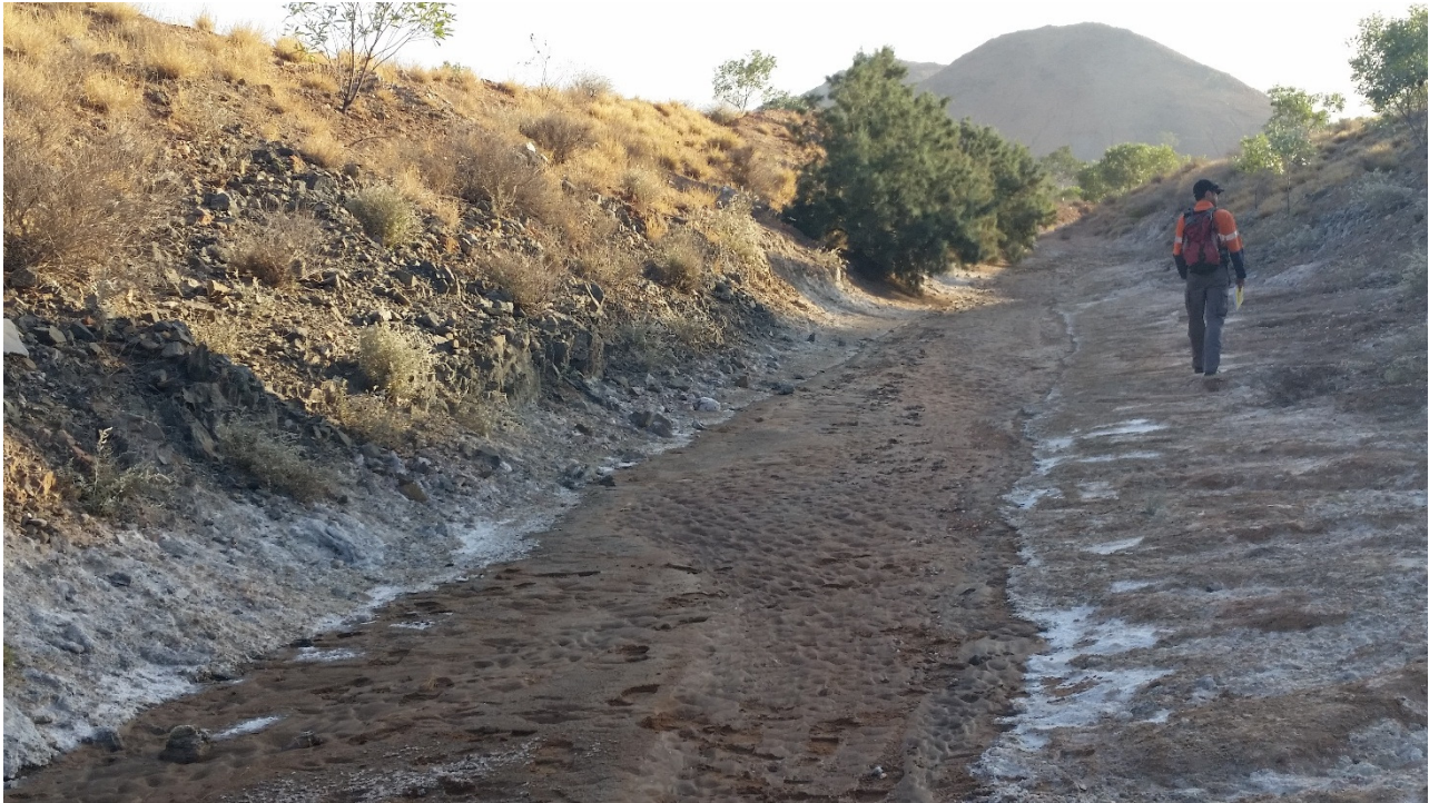
Photograph I-24: Diversion Drain, downstream of BSOC WRD South Seepage, Facing North
