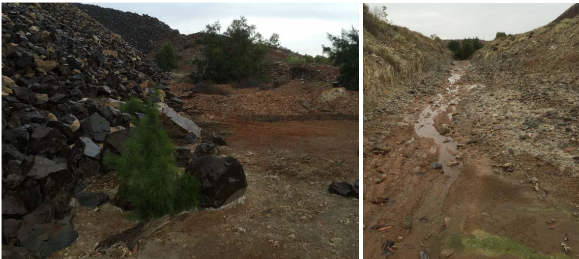
Figure 2-2 Northern Seepage Point a) Toe of BSOC WRD b) Adjacent diversion channel (looking east-northeast)
