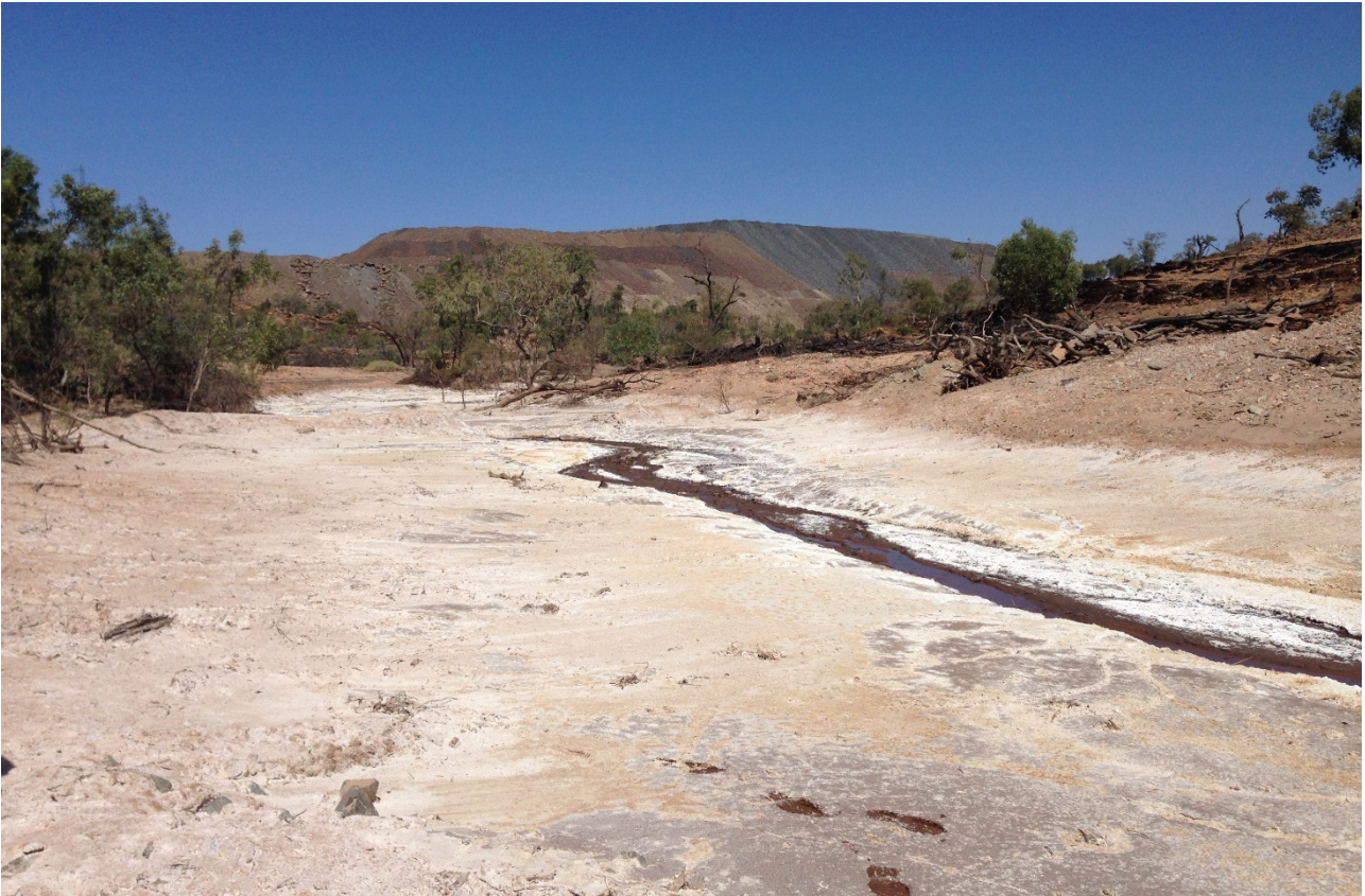
Photograph I-9: King Gully Dam, Upstream; BSOC WRD in background
