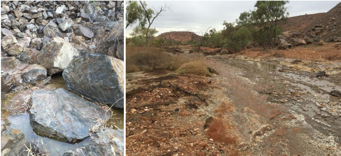
Figure 2-3 TSF3 Seepage Point a) Toe of BSOC WRD b) Adjacent King Gully (looking east-northeast)
