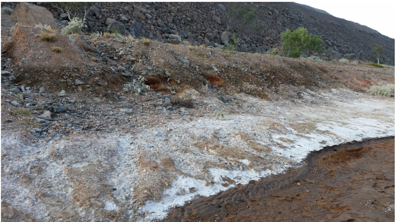
Photograph I-25: Diversion Drain, downstream of BSOC WRD South Seepage, Facing East
