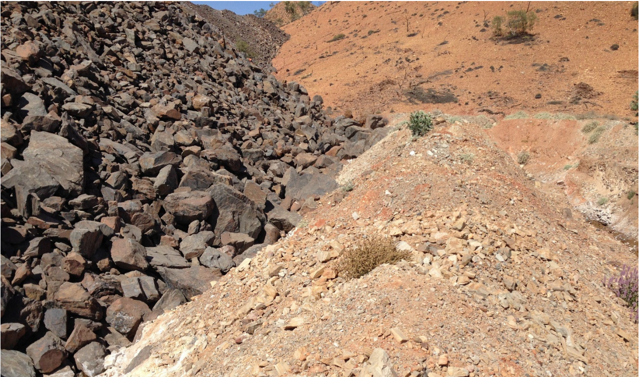
Photograph I-20: BSOC WRD South Seepage Trench, WRD Toe
