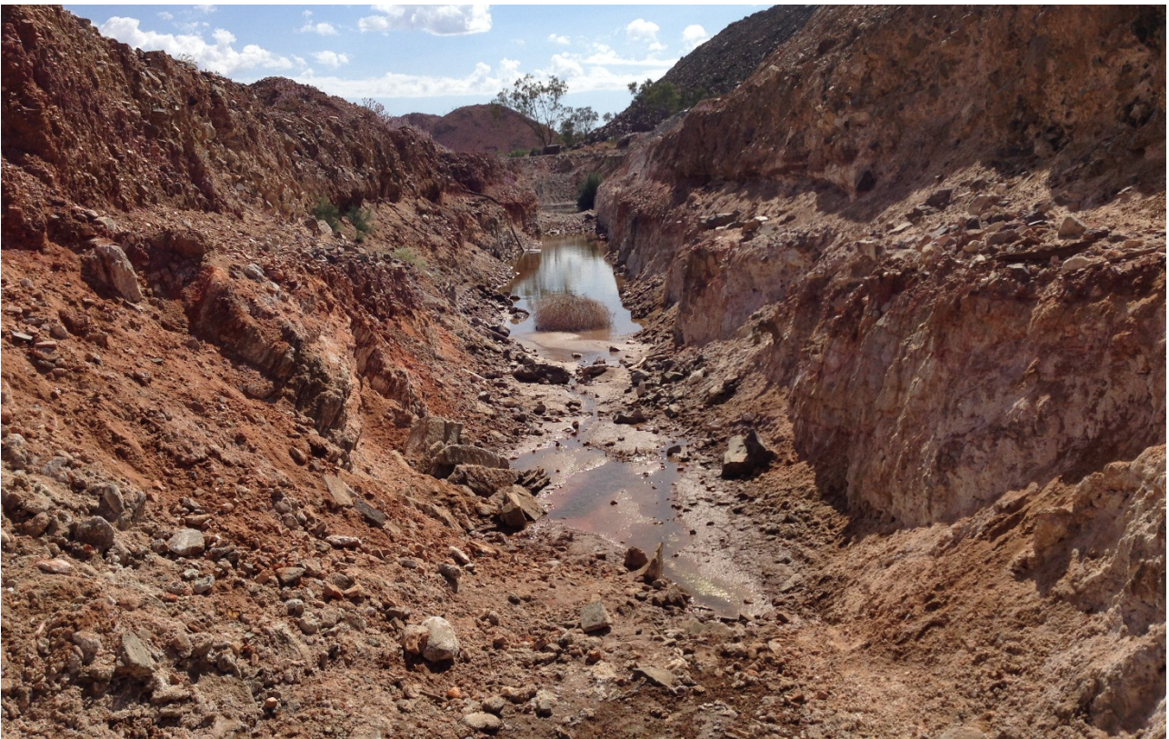
Photograph I-19: BSOC WRD South Seepage Trench, Facing North
