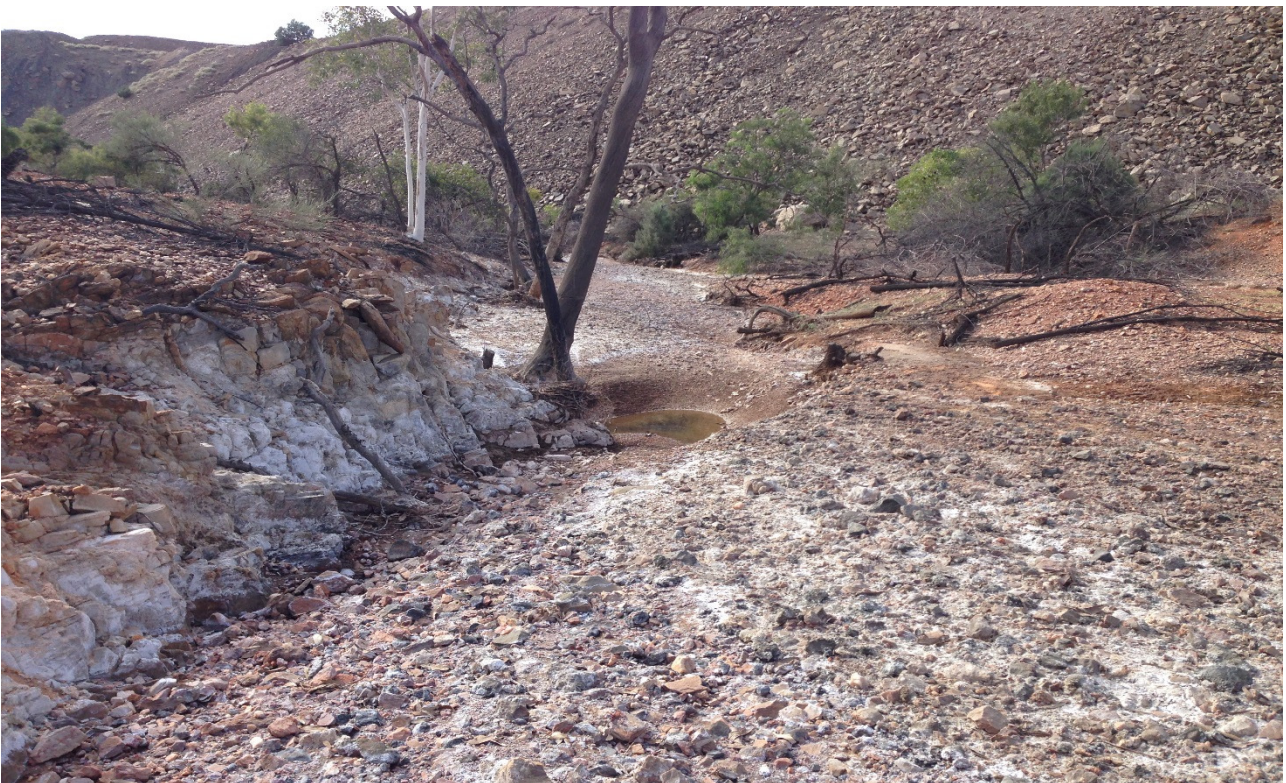
Photograph I-23: Seepage and Precipitation in Diversion Drain, Upstream of TD3 Seepage, Facing East, BSOC WRD in Background
