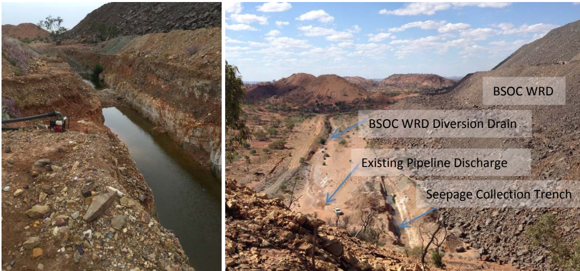
Figure 2-1 Southern Seepage Pit (looking north)
