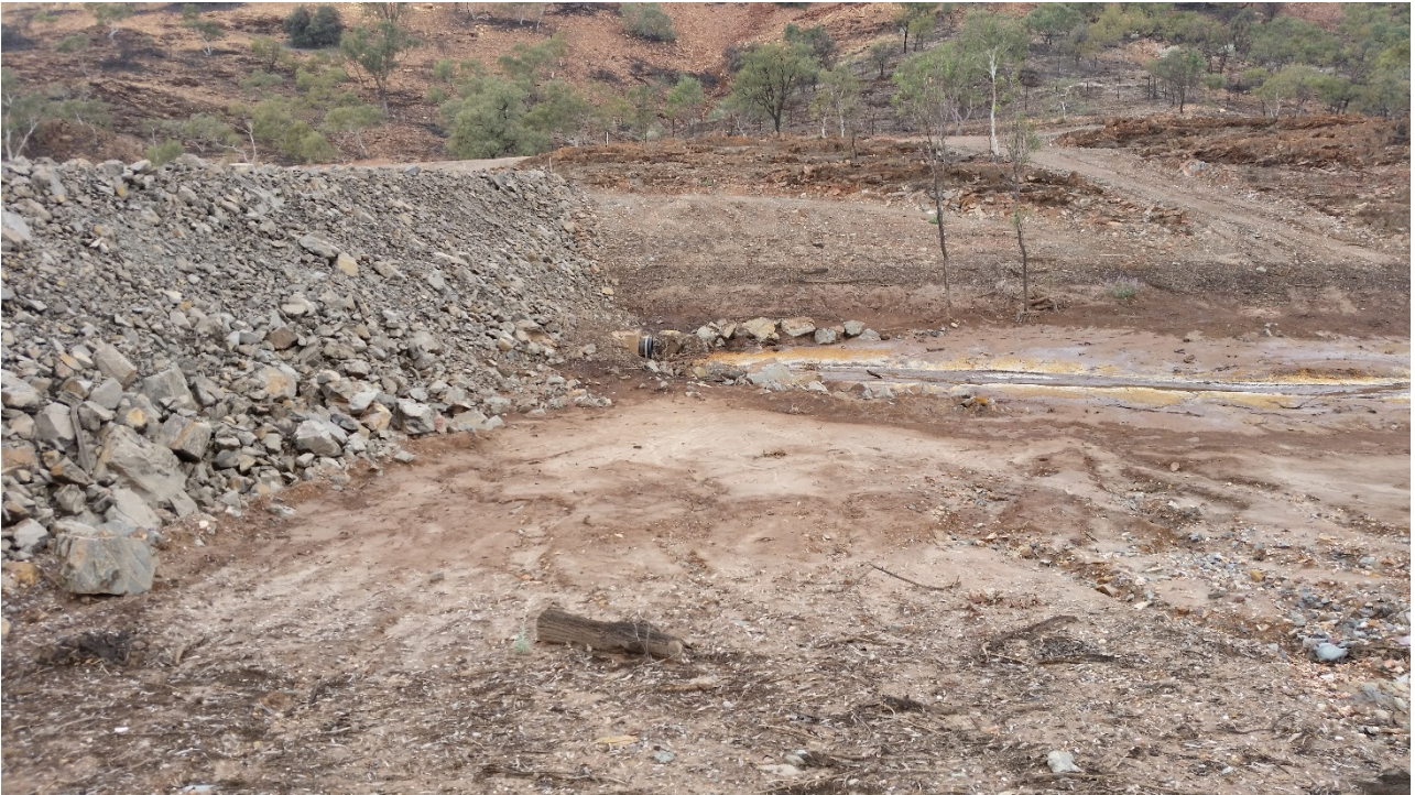
Photograph I-11: King Gully Dam, Upstream
