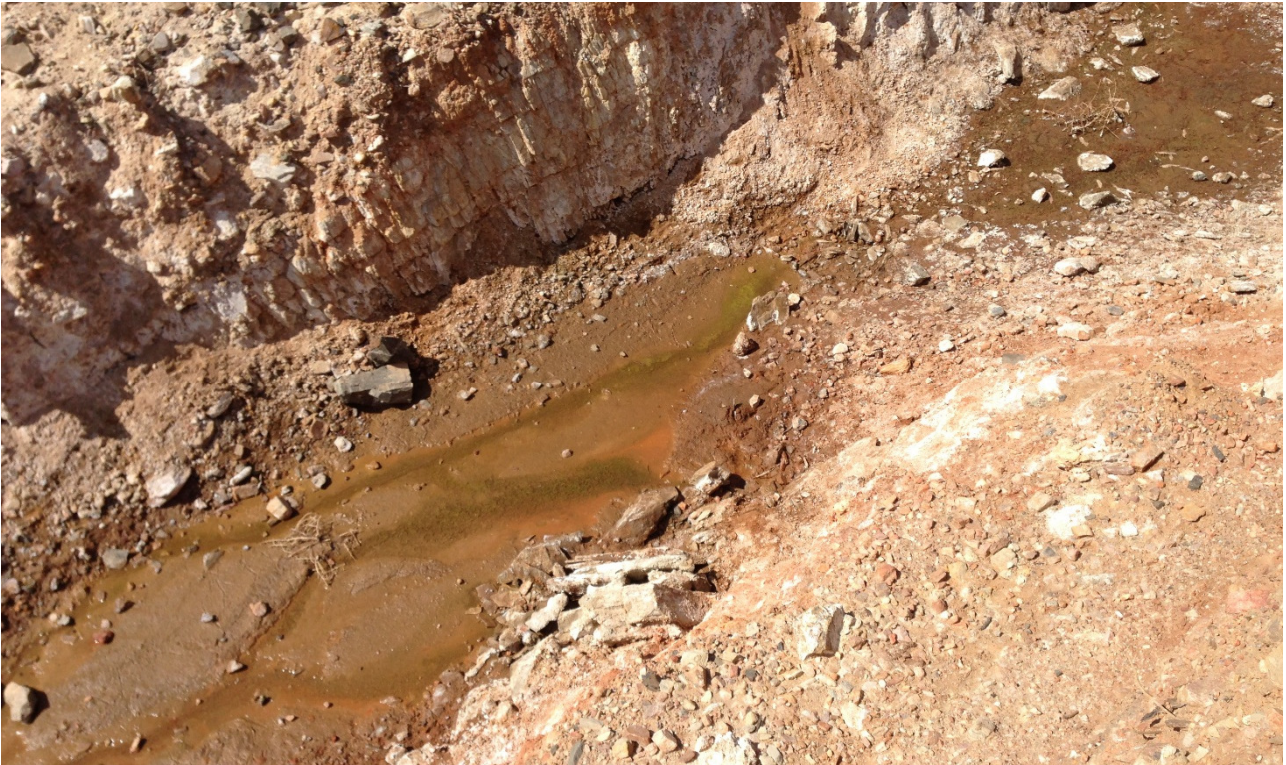
Photograph I-18: BSOC WRD South Seepage Trench
