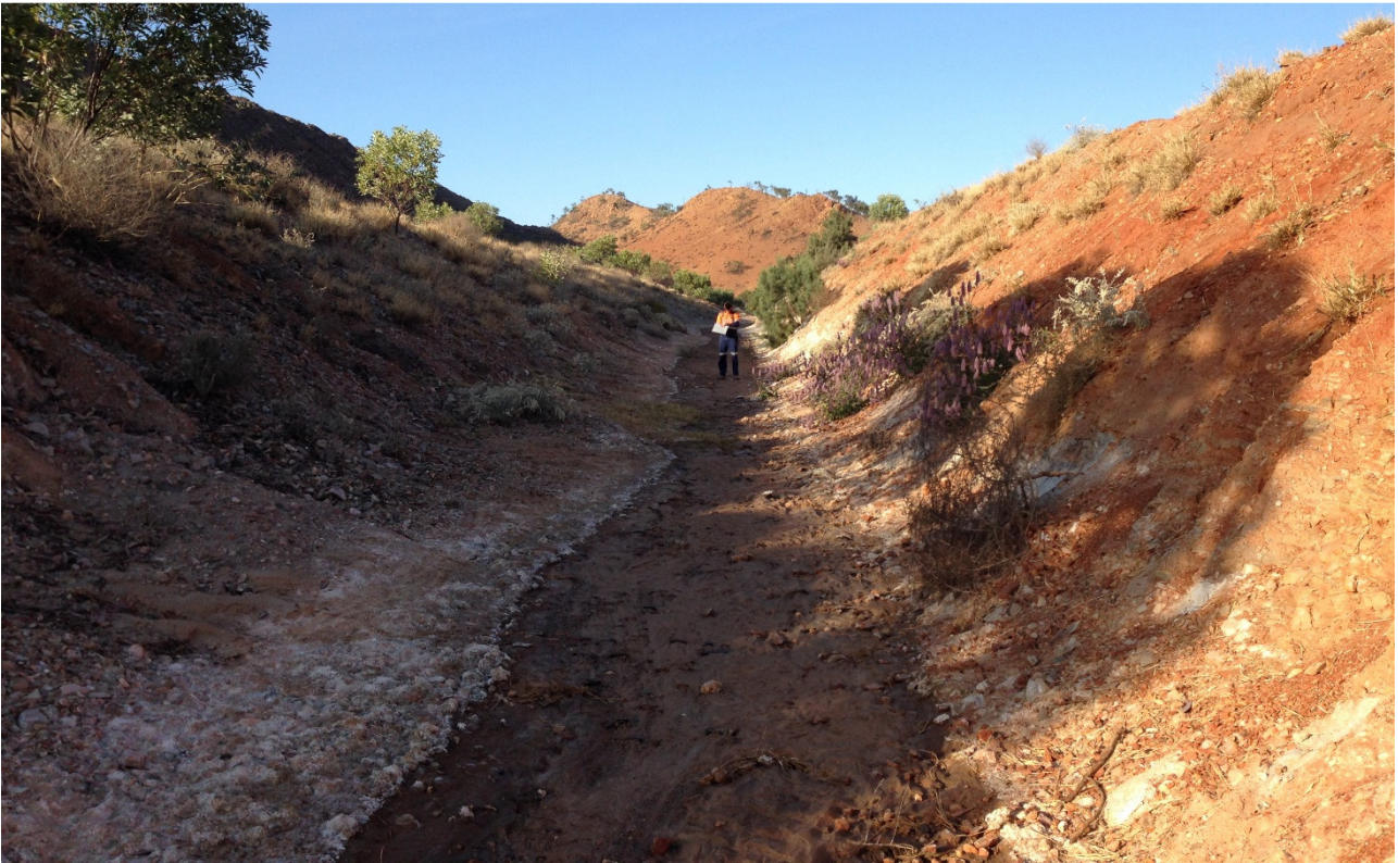
Photograph I-26: Diversion Drain, downstream of BSOC WRD South Seepage, Facing South
