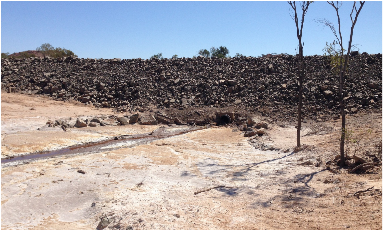
Photograph I-7: King Gully Dam, Upstream
