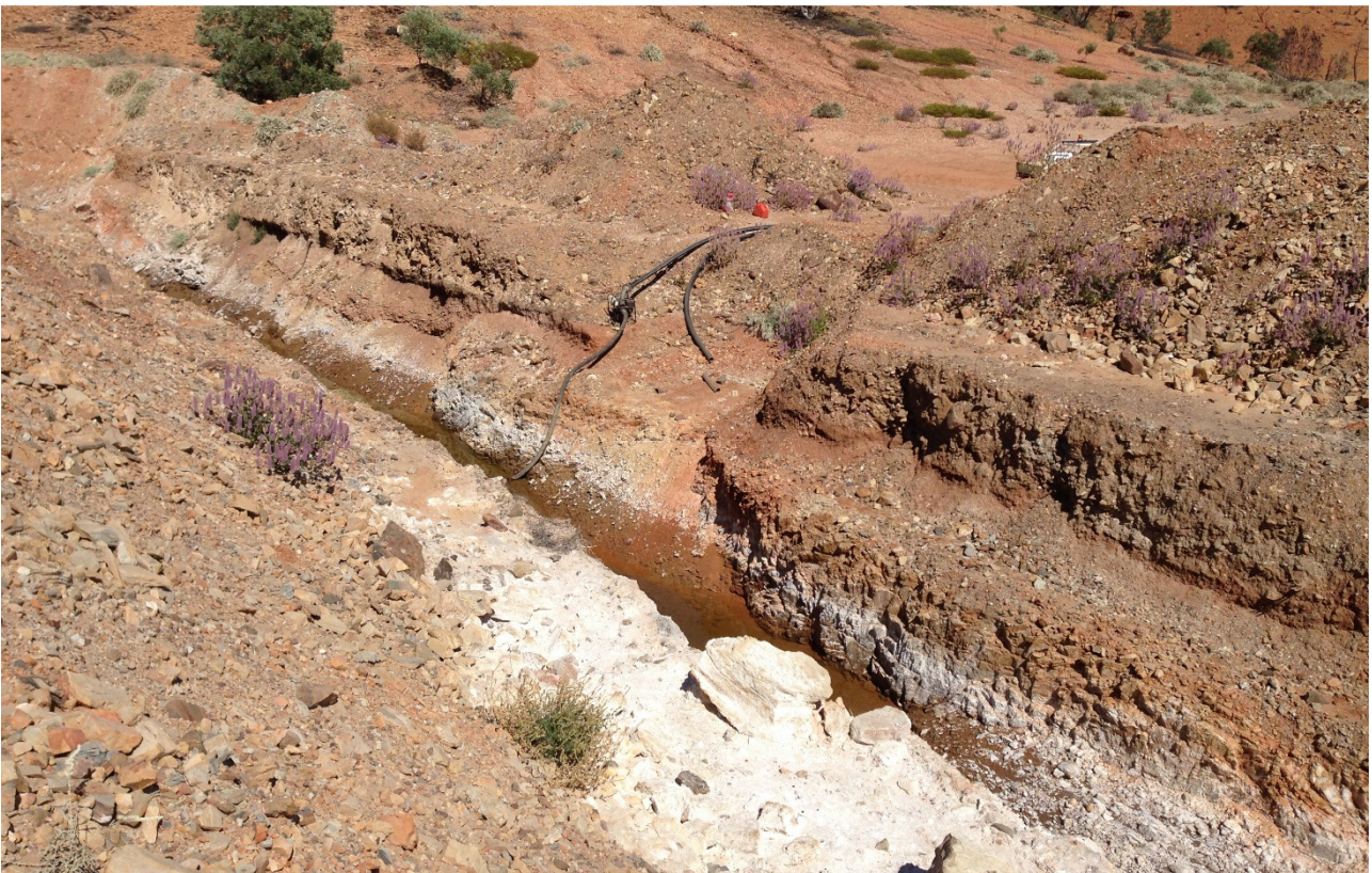
Photograph I-21: BSOC WRD South Seepage Trench, Facing Southwest
