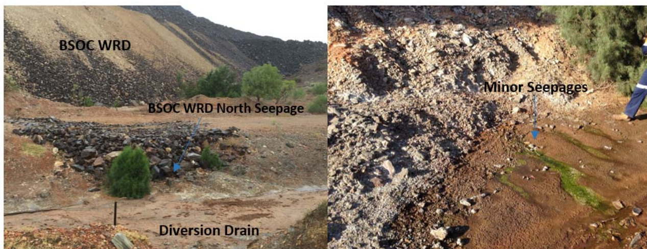
Figure 5-6: BSOC WRD North Seepage. a) Facing south, with BSOC WRD and the Diversion Drain shown, b) Minor seepages identified downstream of the main BSOC WRD North Seepage location (August, 2015)
