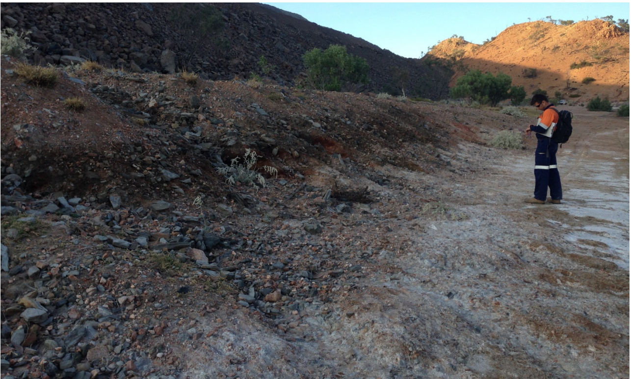
Photograph I-23: Diversion Drain, downstream of BSOC WRD South Seepage
