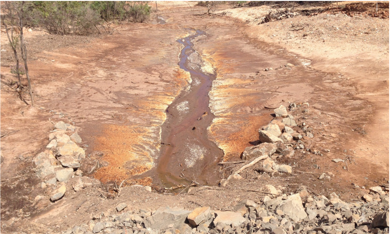
Photograph I-10: King Gully Dam, Upstream
