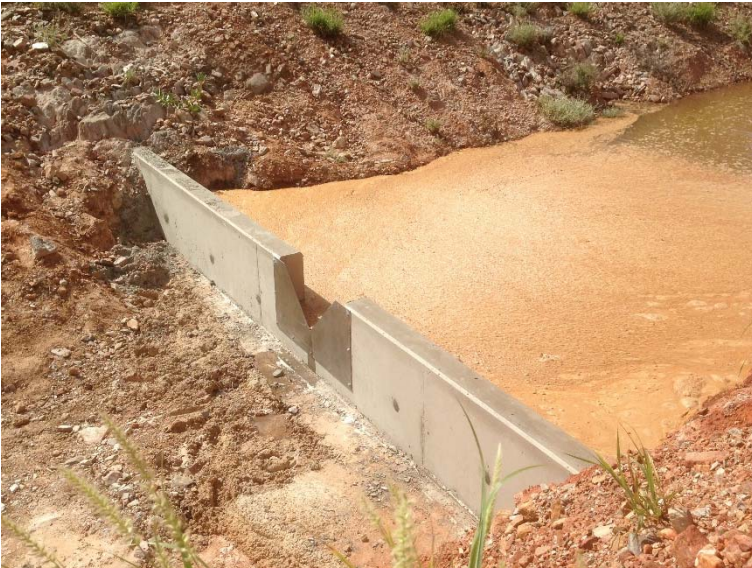
Figure 5-28: BSOC WRD Weir 3 after construction (January, 2016)
