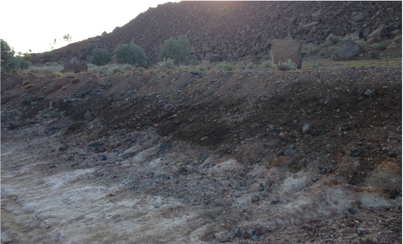
Photograph I-22: Diversion Drain, downstream of BSOC WRD South Seepage
