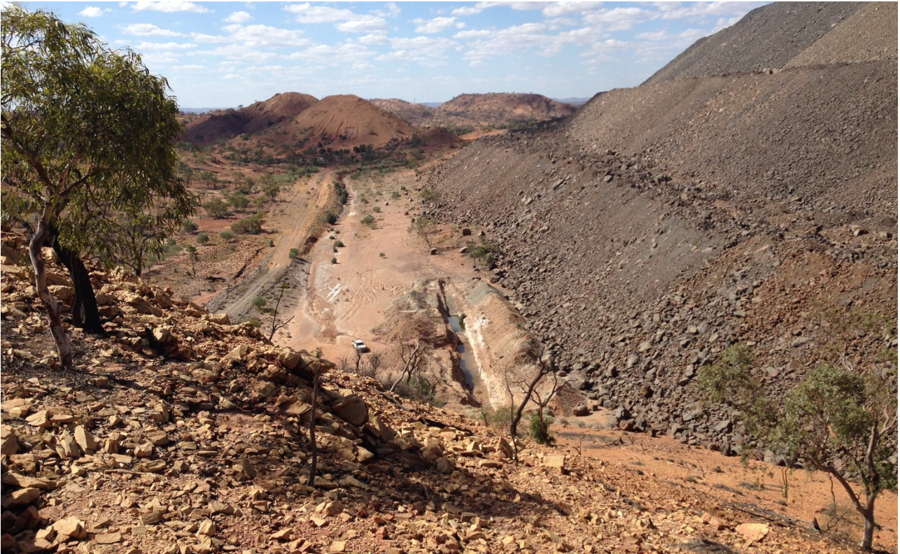
Photograph I-16: Western Edge of BSOC WRD, Facing North; Seepage Trench at BSOC WRD South – start of diversion drain
