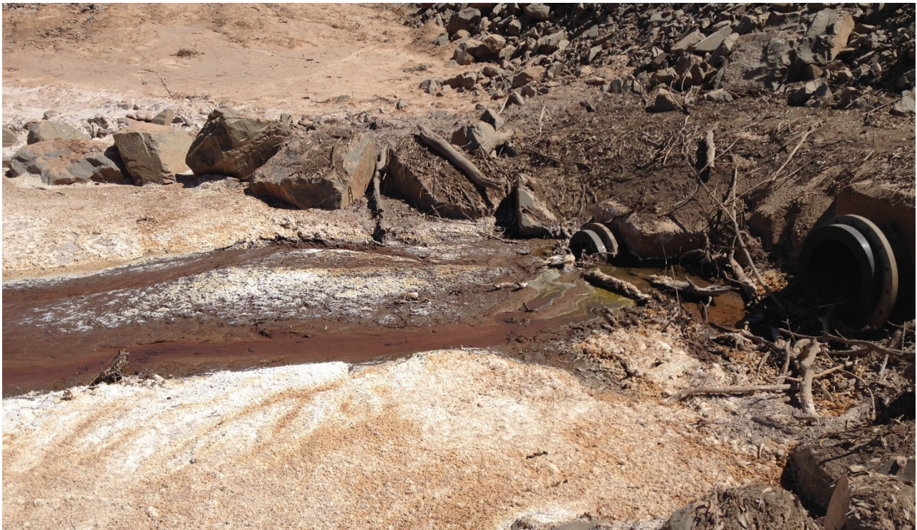
Photograph I-8: King Gully Dam In-Take Pipe, Upstream
