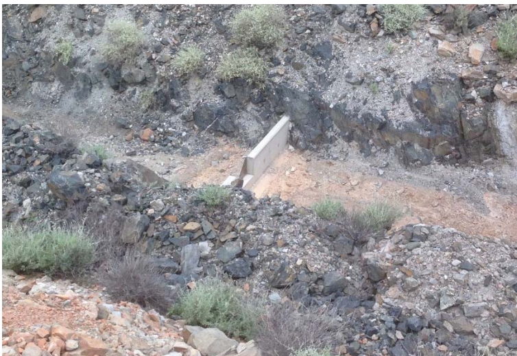
Figure 5-27: BSOC WRD Weir 2 after construction (January, 2016)
