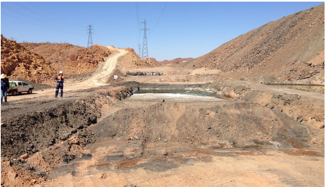
Photograph I-2: Sludge Pit 3 Facing South
