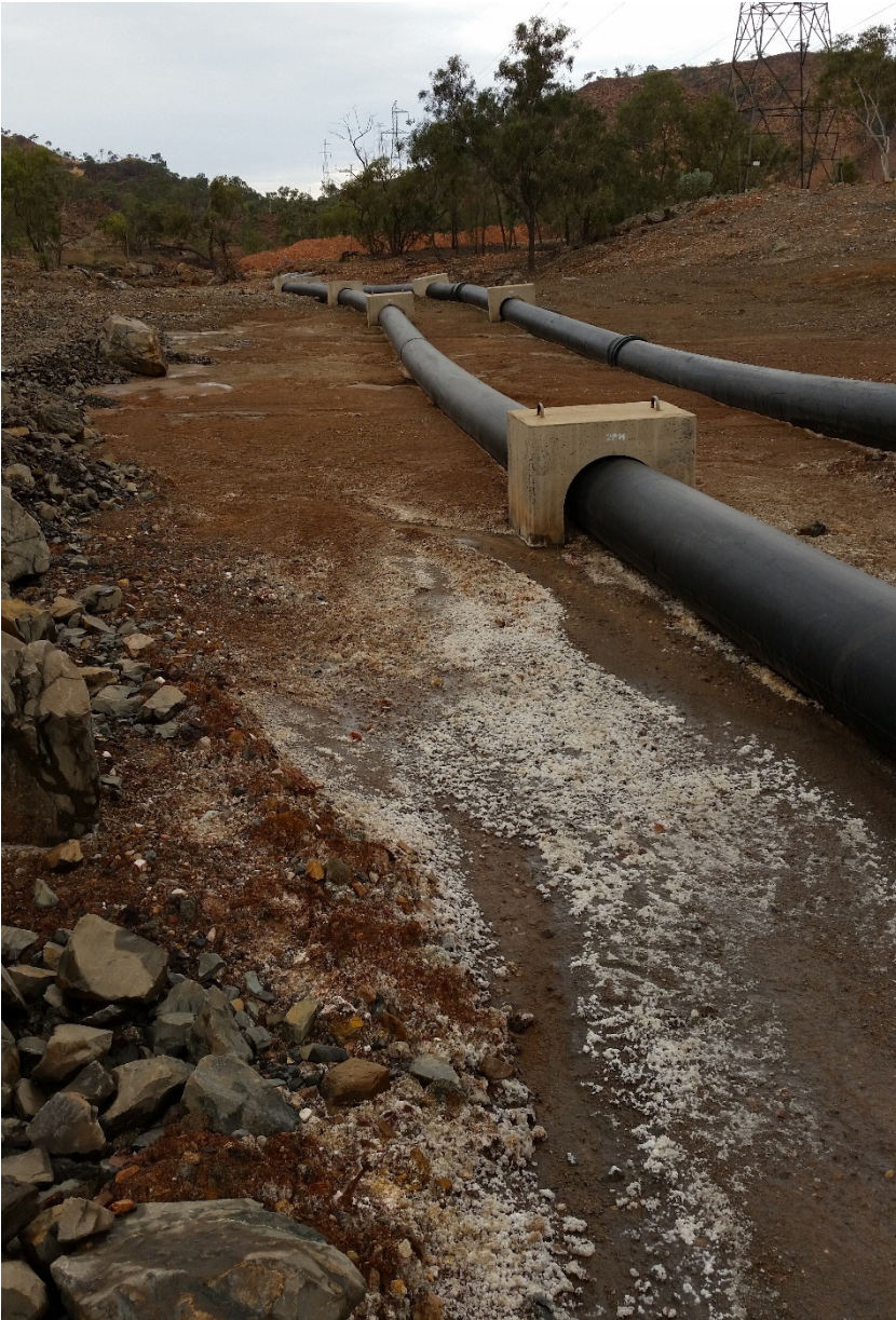
Photograph I-13: King Gully Dam, Downstream
