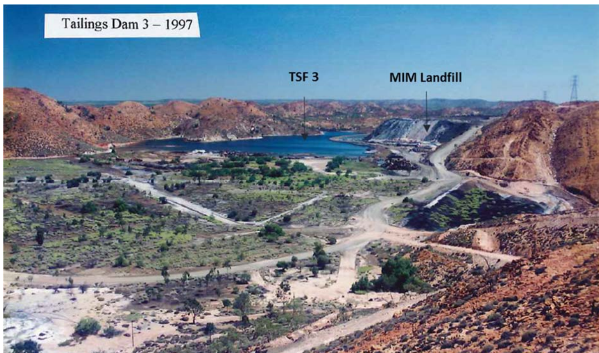
Figure 4-6: TSF3 historical photograph from 1997 facing north and shows the partially rehabilitated TSF3 and MIM landfill to the east
