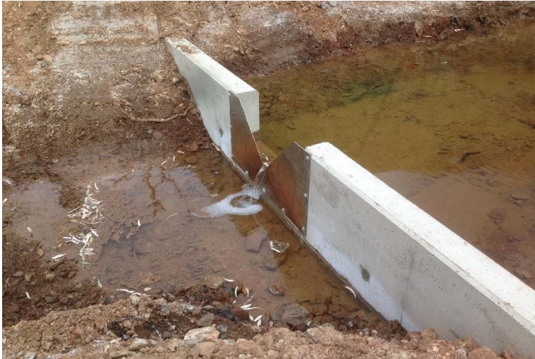
Figure 5-26: BSOC WRD Weir 1 after construction (January, 2016)
