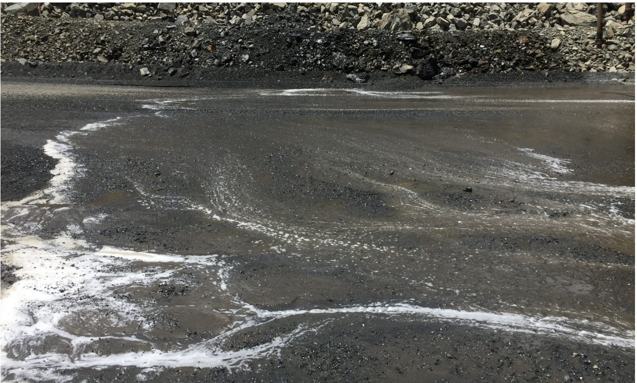
Photograph IX-4: Surface Test at Highly Trafficked Area
